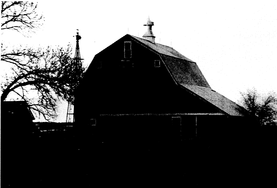
Lehman Barn also constructed by Mr. Monick in 1915, located three miles west of Eliason Barn (Spencer, 2008)
