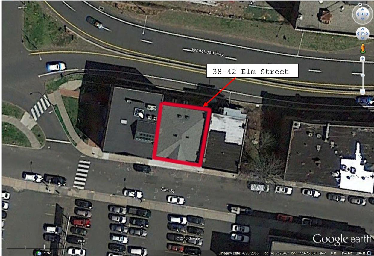
Figure 2. Aerial photograph showing site of Mansuy and Smith Automobile Showroom Building at 38-42 Elm Street.
