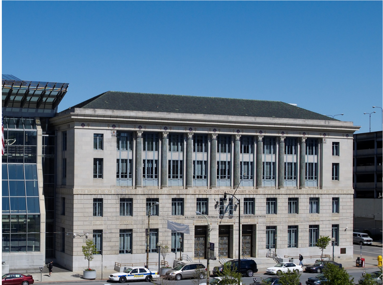
Figure 3. Exterior, view looking northwest, of southeast façade showing 1931 building.
