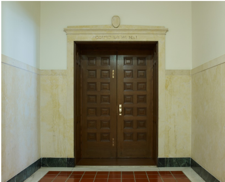
Figure 7. Interior, representative courtroom door.
