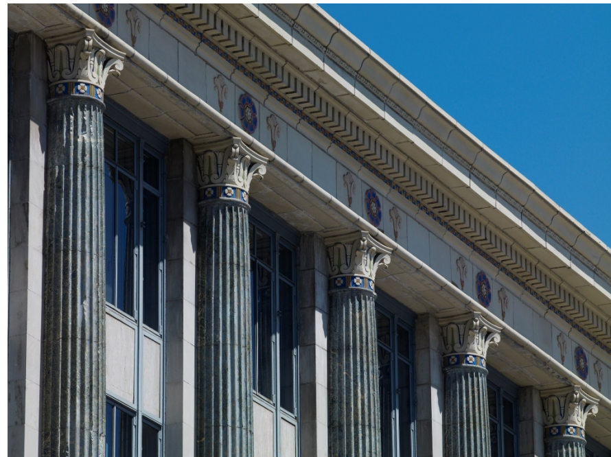
Figure 4. Exterior, view looking northwest, at southeast façade, detail of columns.
