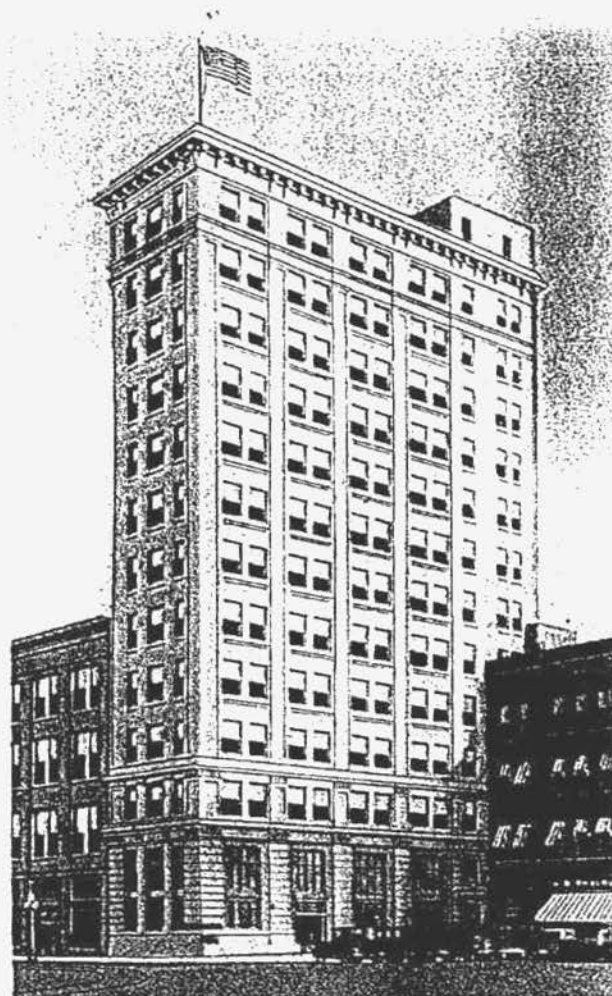
FIRST NATIONAL BANK BUILDING, DANVILLE, ILL.
