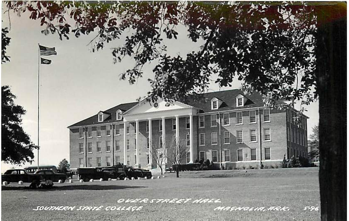
Overstreet Hall – c.1945
