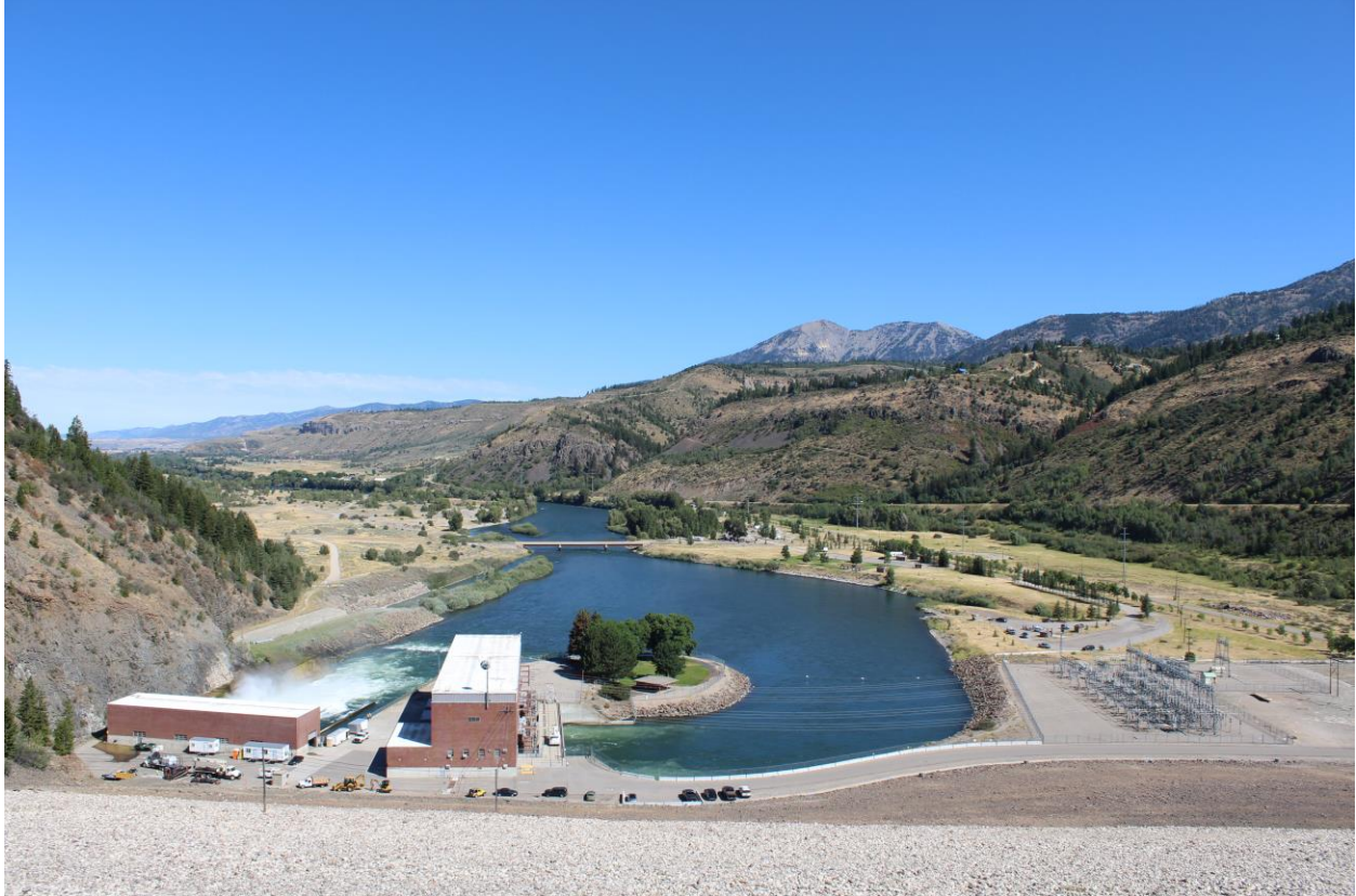
Photo 3 of 30. General view of gate house, powerplant, Vista Park, tailrace and switchyard. View to north.
