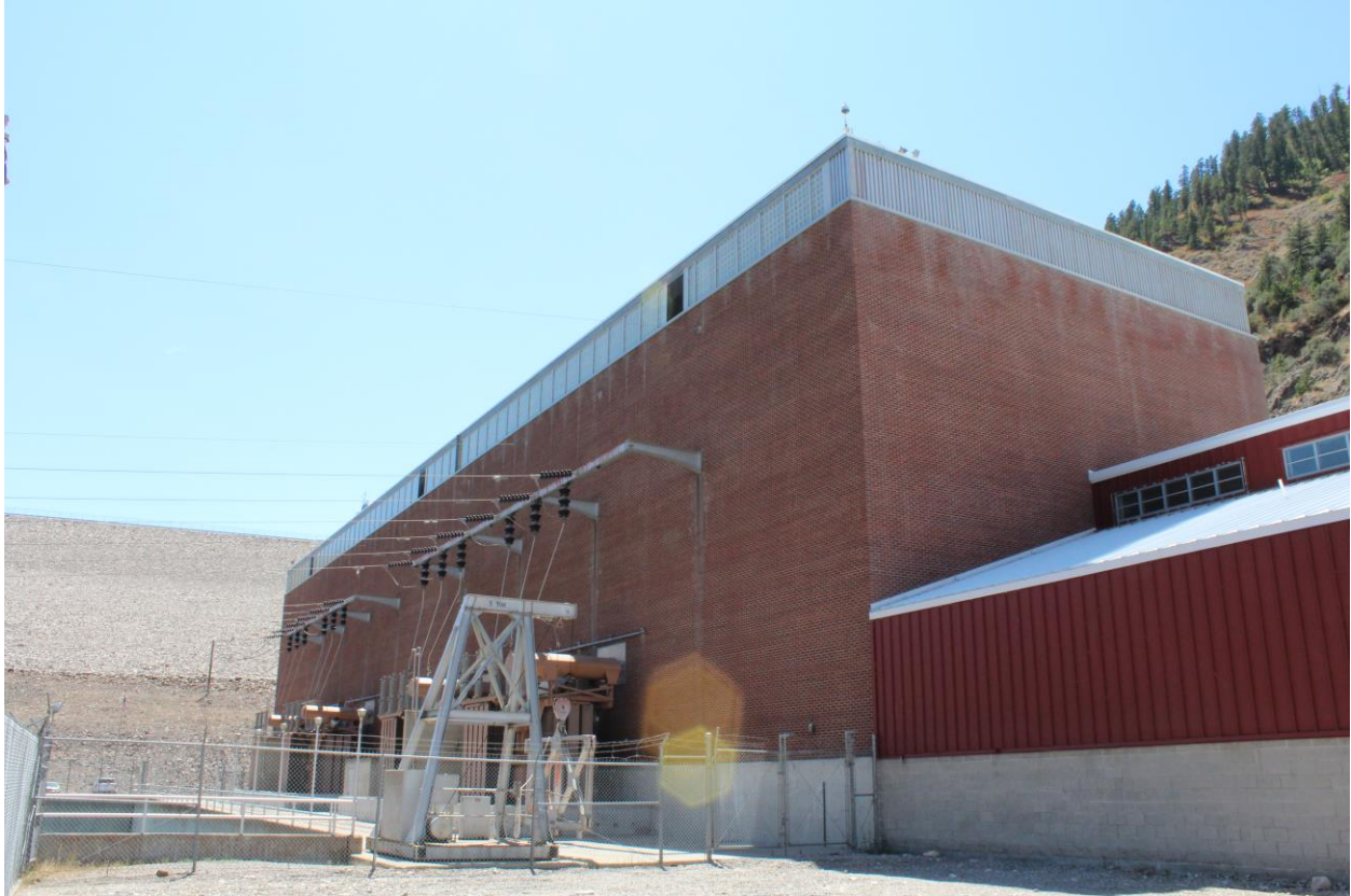
Photo 17 of 30. Powerplant transformer deck. View to southwest.
