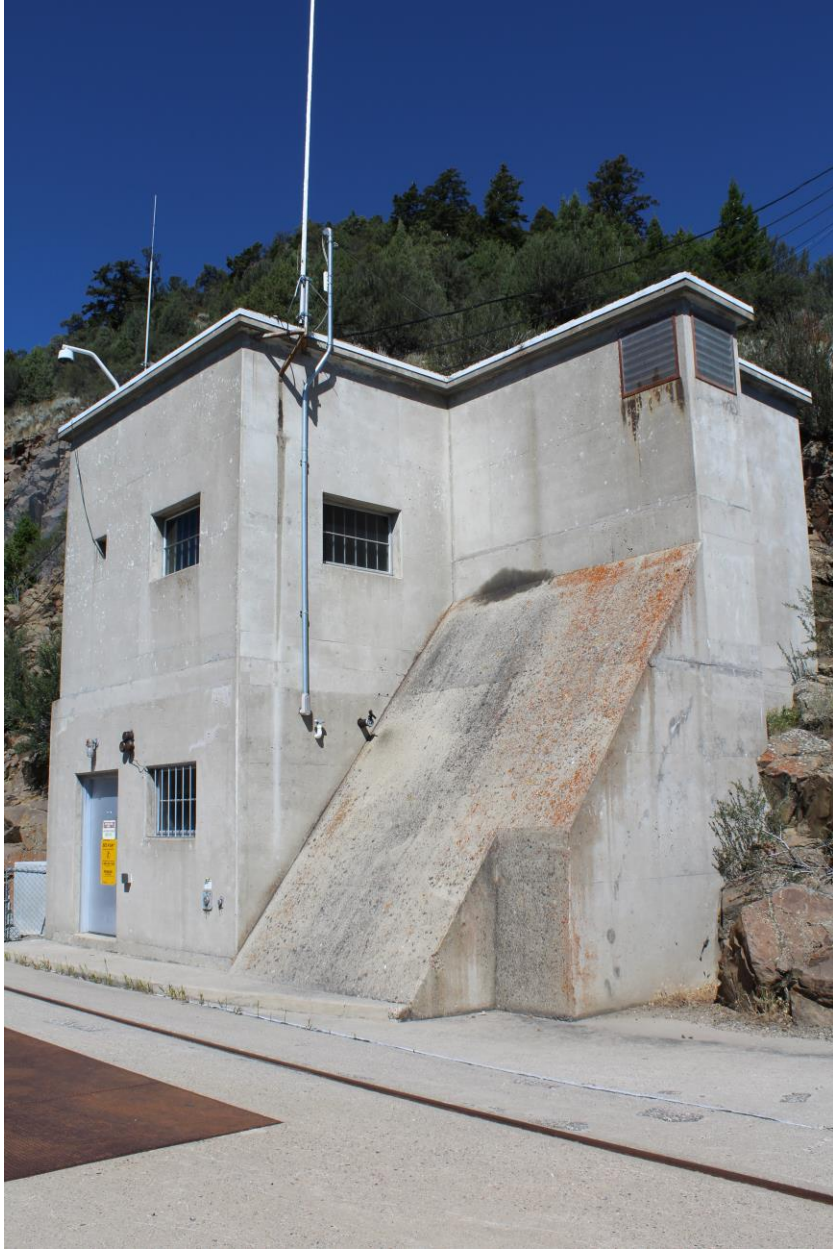
Photo 10 of 30. Power tunnel intake gate structure. View to northwest.
