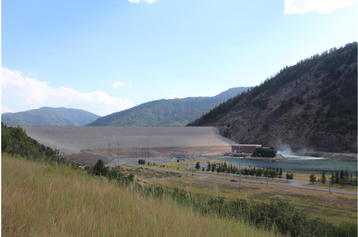
Photo 2 of 30. General view of dam, powerplant and switchyard. View to southwest.
