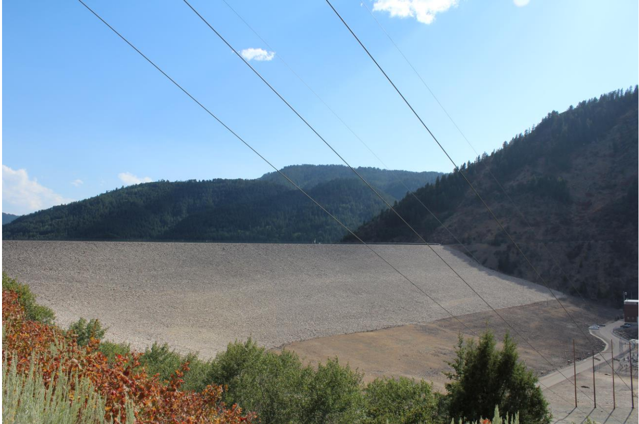
Photo 5 of 30. Dam, downstream slope. View to southwest.
