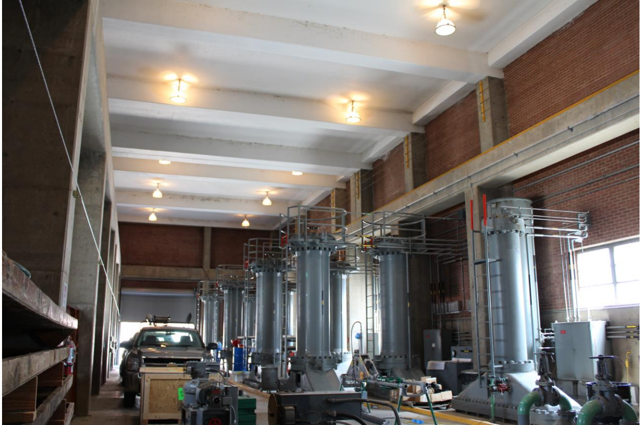
Photo 14 of 30. Interior of gate house. View to east.
