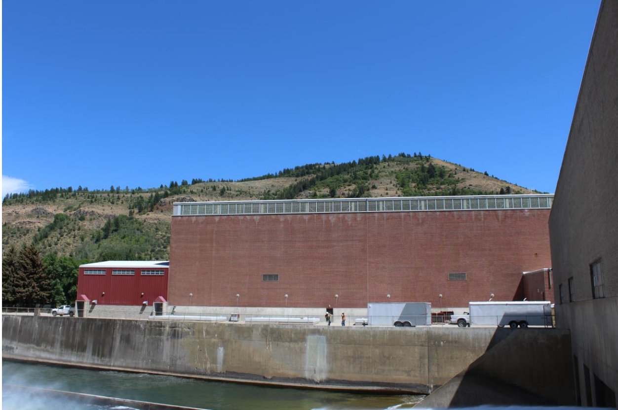
Photo 19 of 30. Powerplant west elevation with stilling basin in foreground. View to east.
