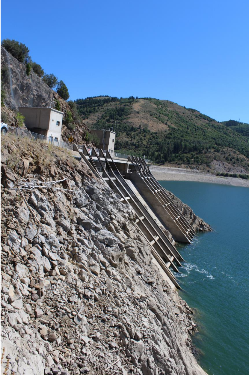
Photo 8 of 30. Outlet and power tunnel intake structures. View to northeast.
