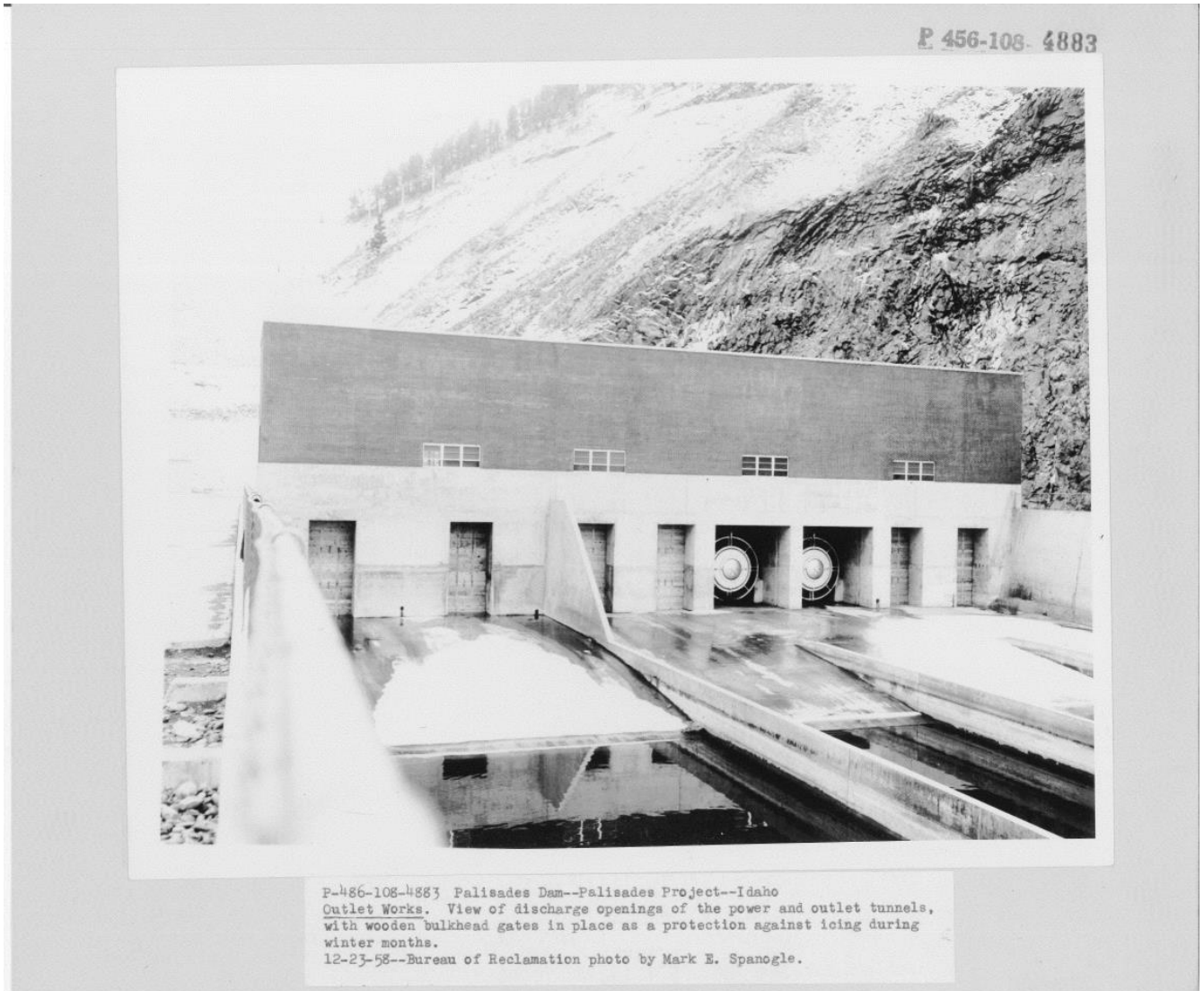
Figure 12. Gate house, discharge openings of the power and outlet tunnels and stilling basin in foreground, 1958.
