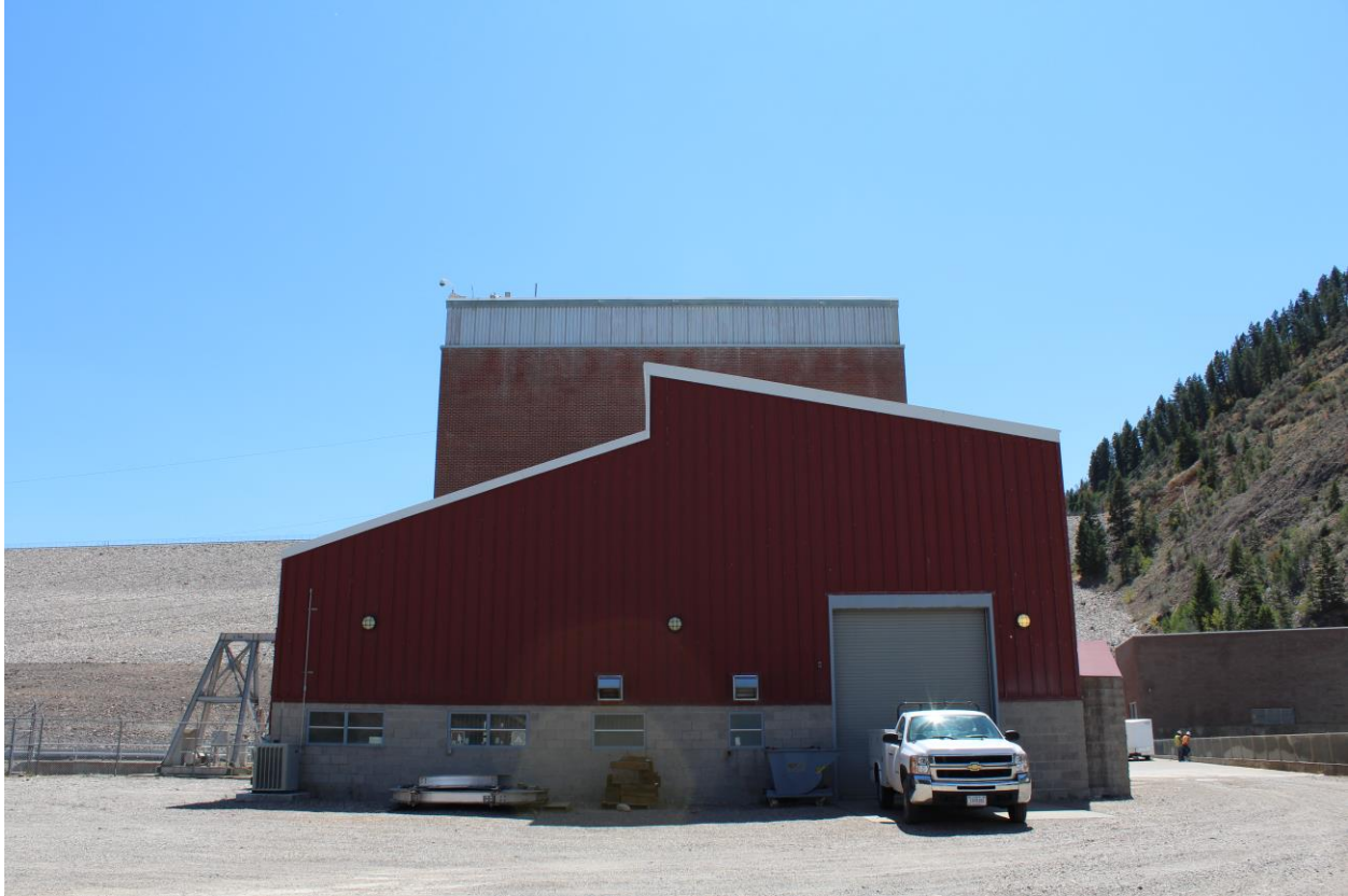
Photo 18 of 30. Powerplant new machine shop addition. View to south.
