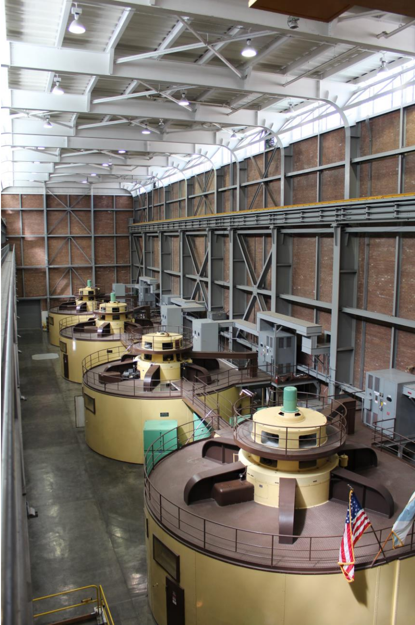
Photo 22 of 30. Interior of powerplant, operating floor. View to northeast.
