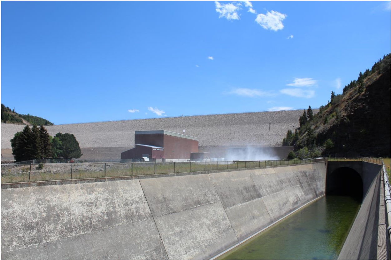
Photo 27 of 30. Spillway channel. View to south.
