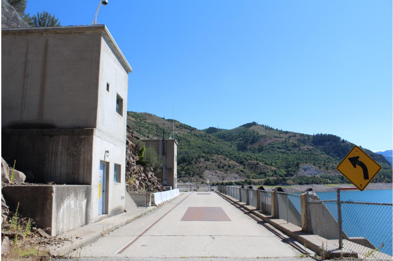
Photo 9 of 30. Bridge crossing intake structures; intake gate structures on left. View to east.
