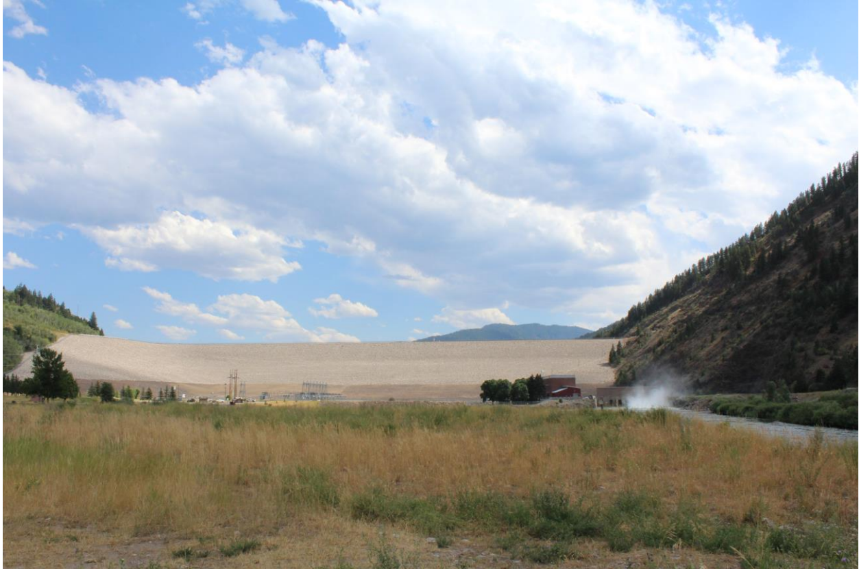
Photo 4 of 30. General view of dam, downstream slope. View to south.
