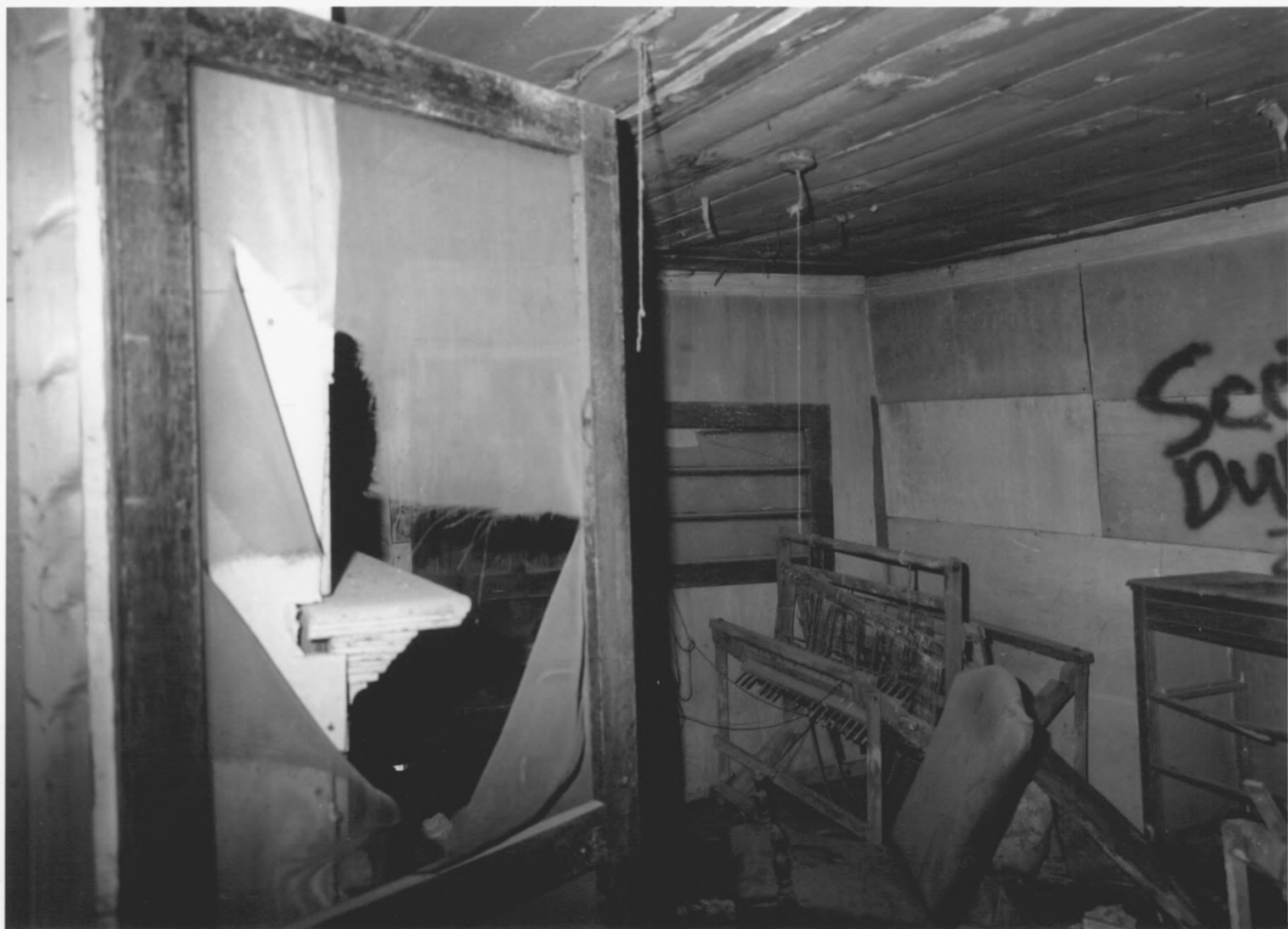
Benlah Rucker House/School Gainesville, Hall County, GA 4 of 5
