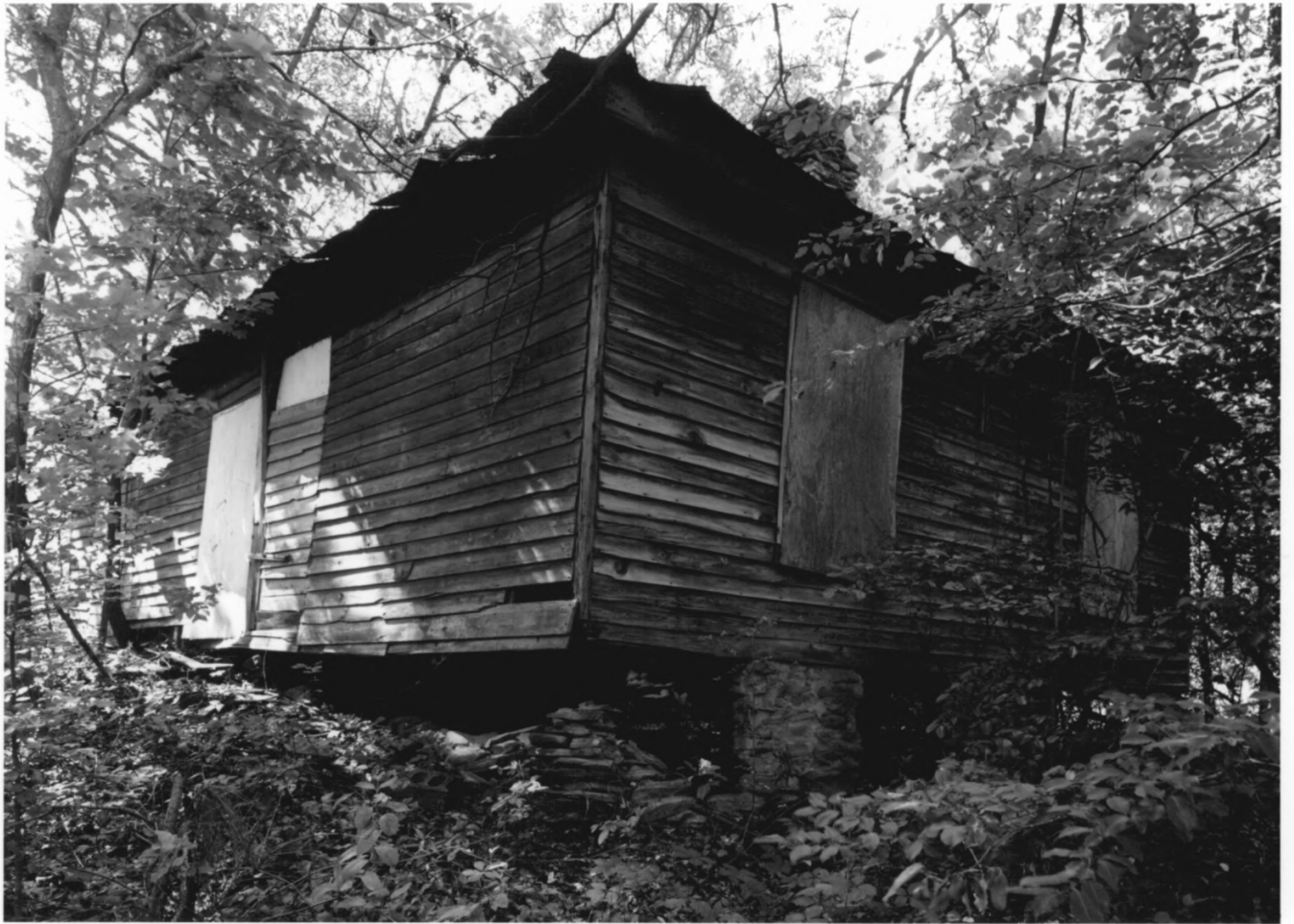
Beulah Rucker House/School Gainesville, Hall County GA 2 of 5
