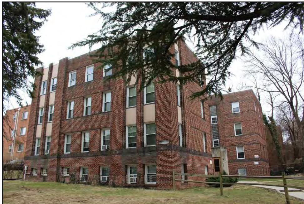
Photo 1 of 18: North and west elevations, looking SE.
