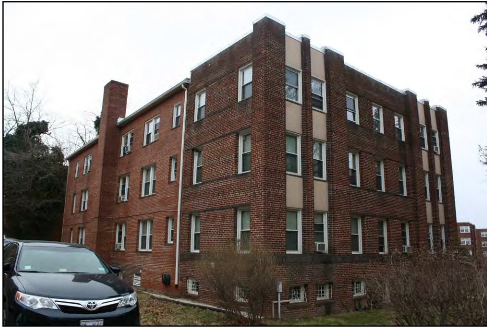
Photo 14 of 18: North and East elevation, looking SW.
