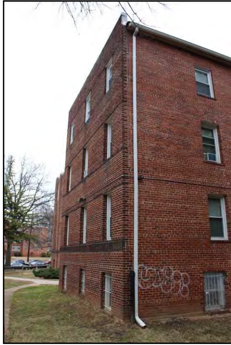
Photo 18 of 18: Southwest corner of building, looking NE.
