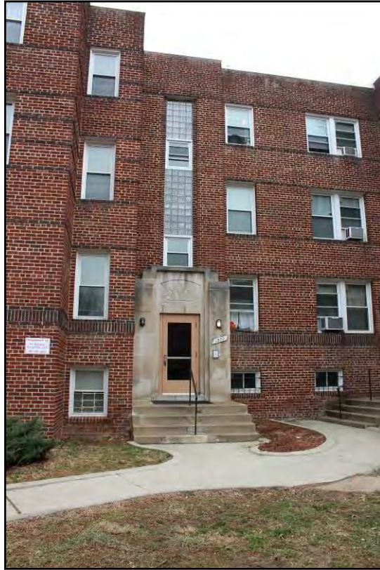
Photo 10 of 18: 1370 entrance, looking SE.
