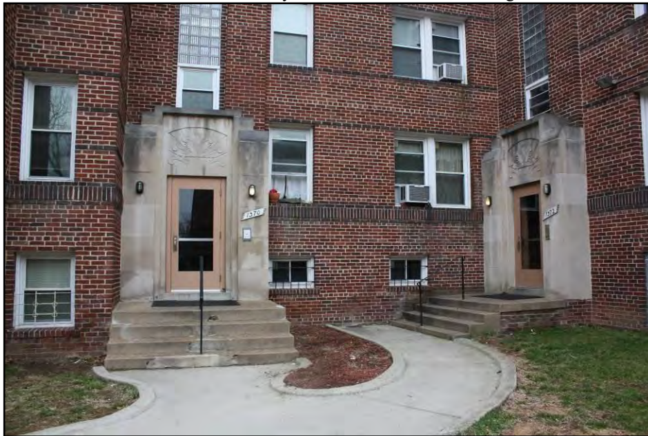
Photo 9 of 18: Main entrances labelled 1370 and 1372, looking SE.
