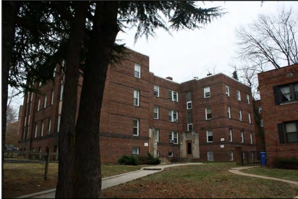
Photo 6 of 18: North and west elevation, looking SE.
