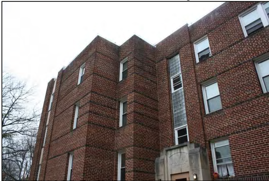
Photo 11 of 18: Northern portion of West elevation, looking NE.
