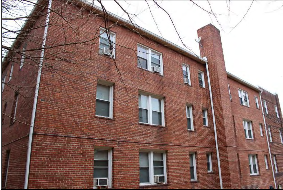
Photo 16 of 18: East elevation, looking NW.
