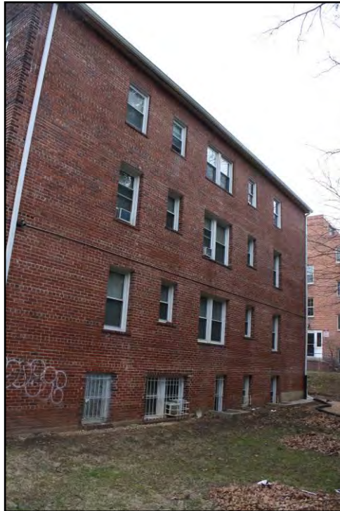
Photo 17 of 18: South (rear) elevation, looking E.
