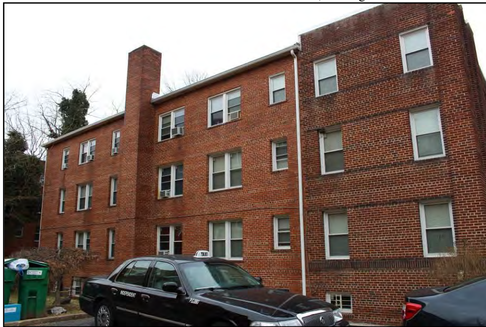
Photo 15 of 18: East elevation, looking SW.
