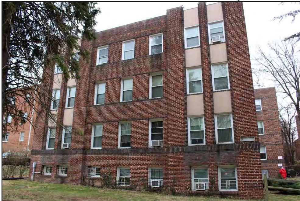
Photo 13 of 18: North elevation, looking S.
