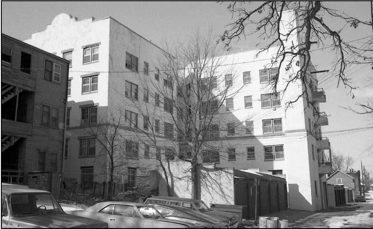
Figure 6: Rear of Hanscom Apartments, circa 1985. Note the garage structure visible in the center foreground, and the other garage structure just visible near the bottom right corner, along the alley. Photo available from the Omaha Planning Department.
