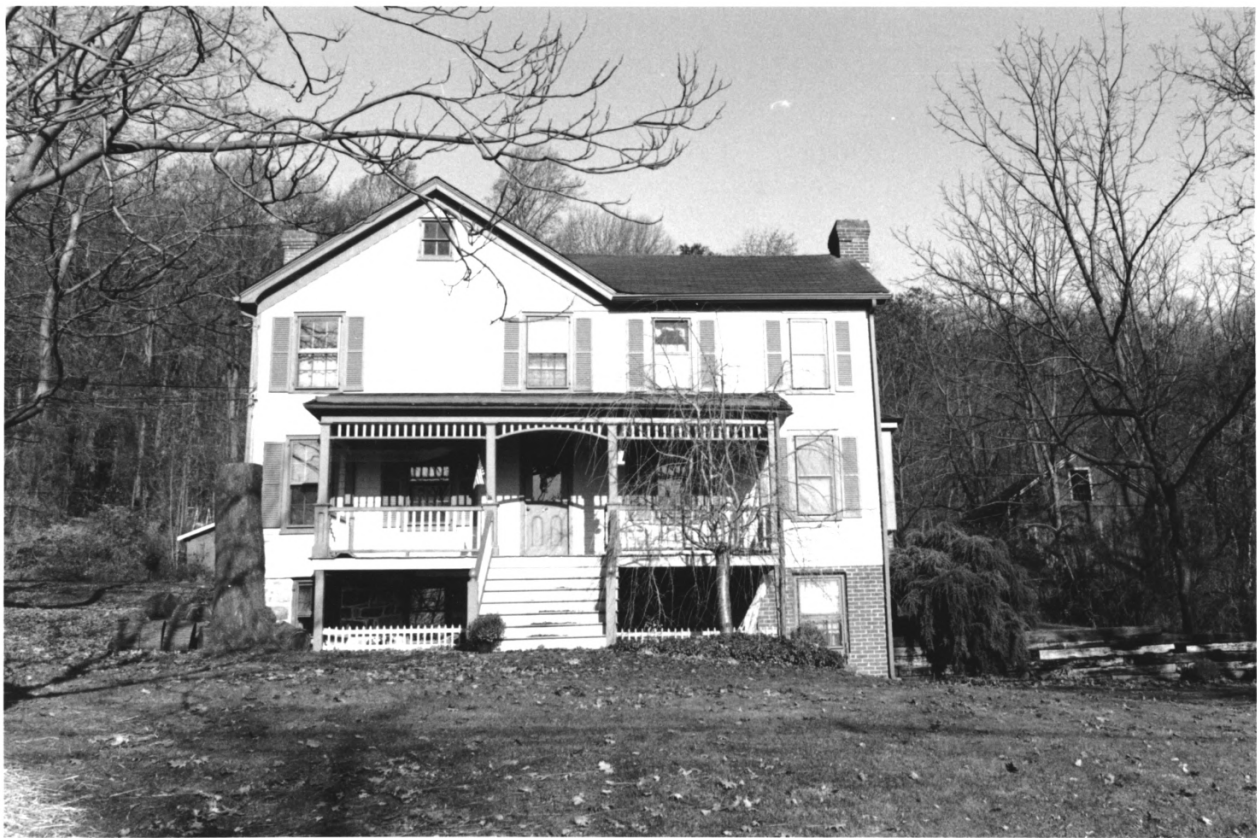
BROOKSIDE HISTORIC DISTRICT 034/027 PHOTO 3 OF 47
