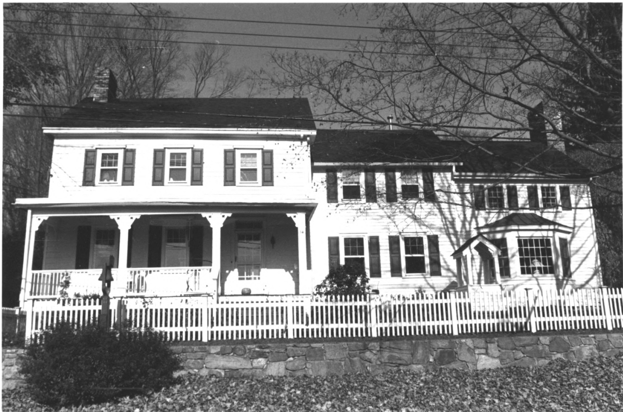
BROOKSIDE HISTORIC DISTRICT 034/027 PHOTO 19 OF 47
