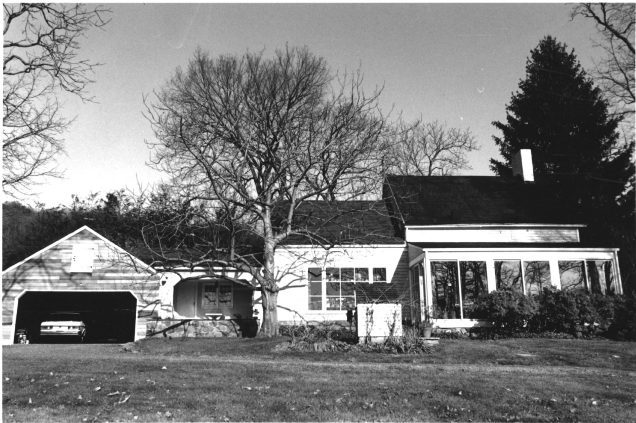
BROOKSIDE HISTORIC DISTRICT 034/027 PHOTO 1 OF 47
