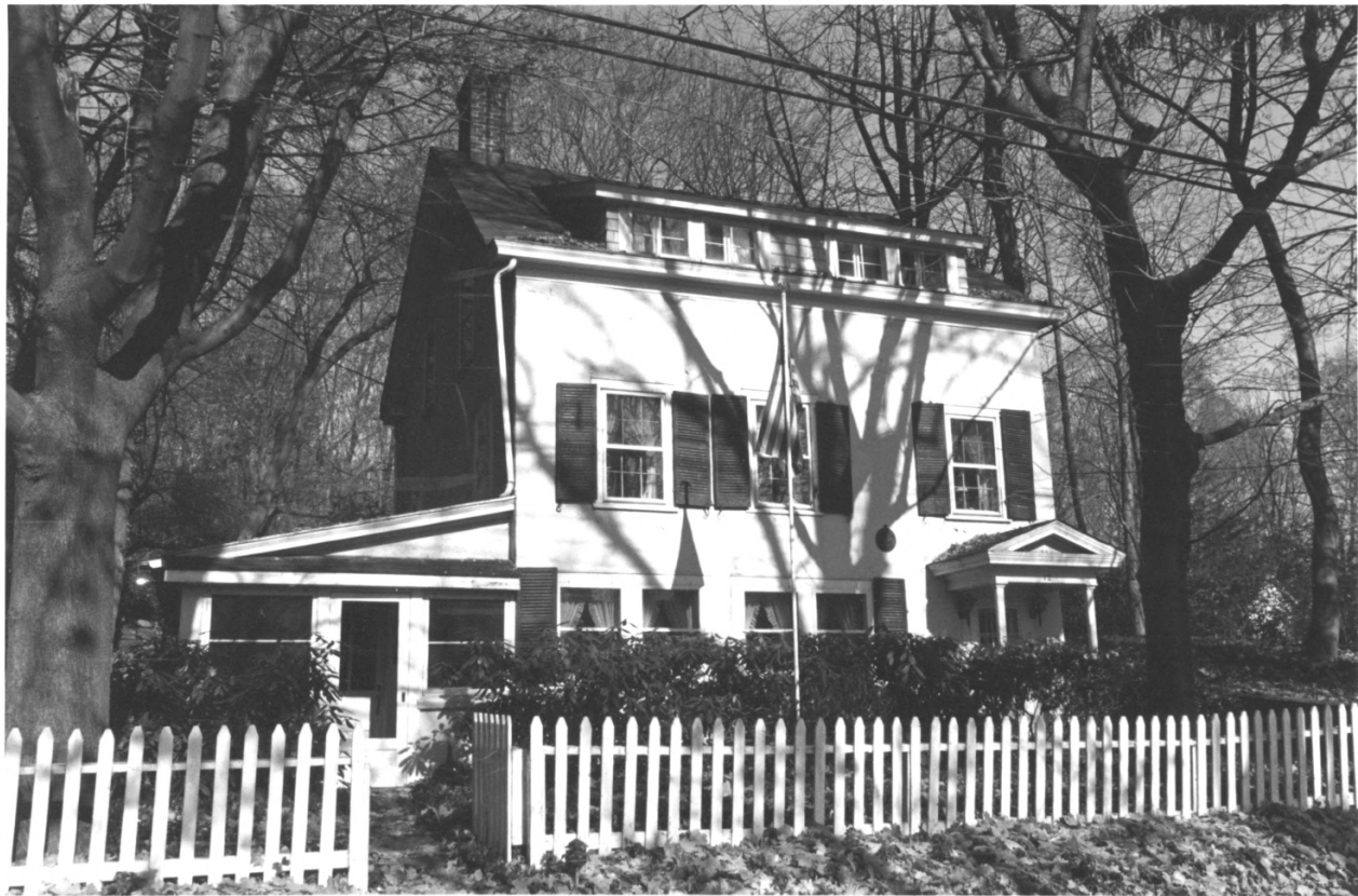
BROOKSIDE HISTORIC DISTRICT 034/027 PHOTO 18 OF 47
