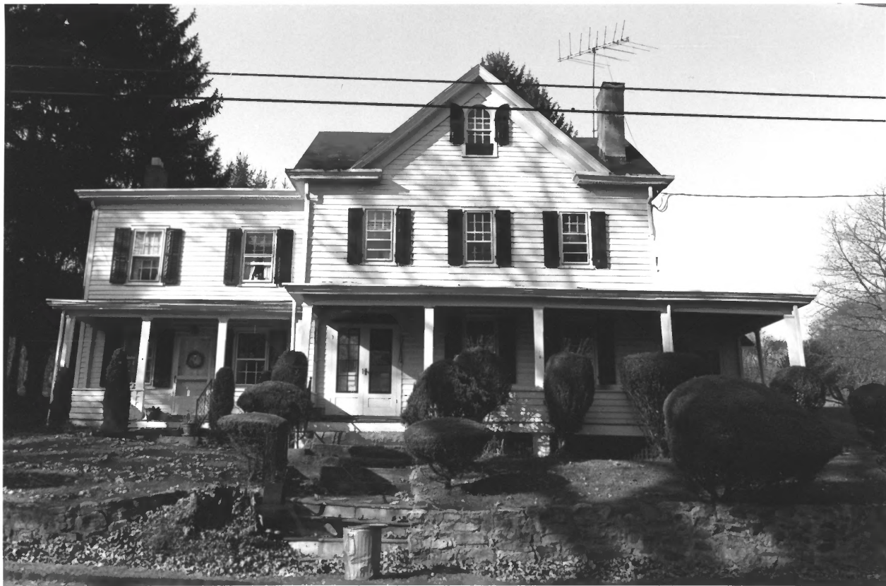
BROOKSIDE HISTORIC DISTRICT 034/027 PHOTO 23 OF 47
