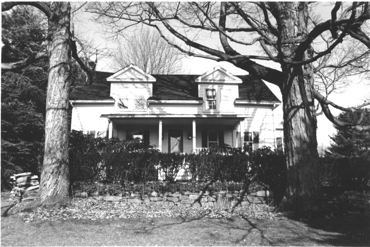
BROOKSIDE HISTORIC DISTRICT 034/027 PHOTO 5 OF 47
