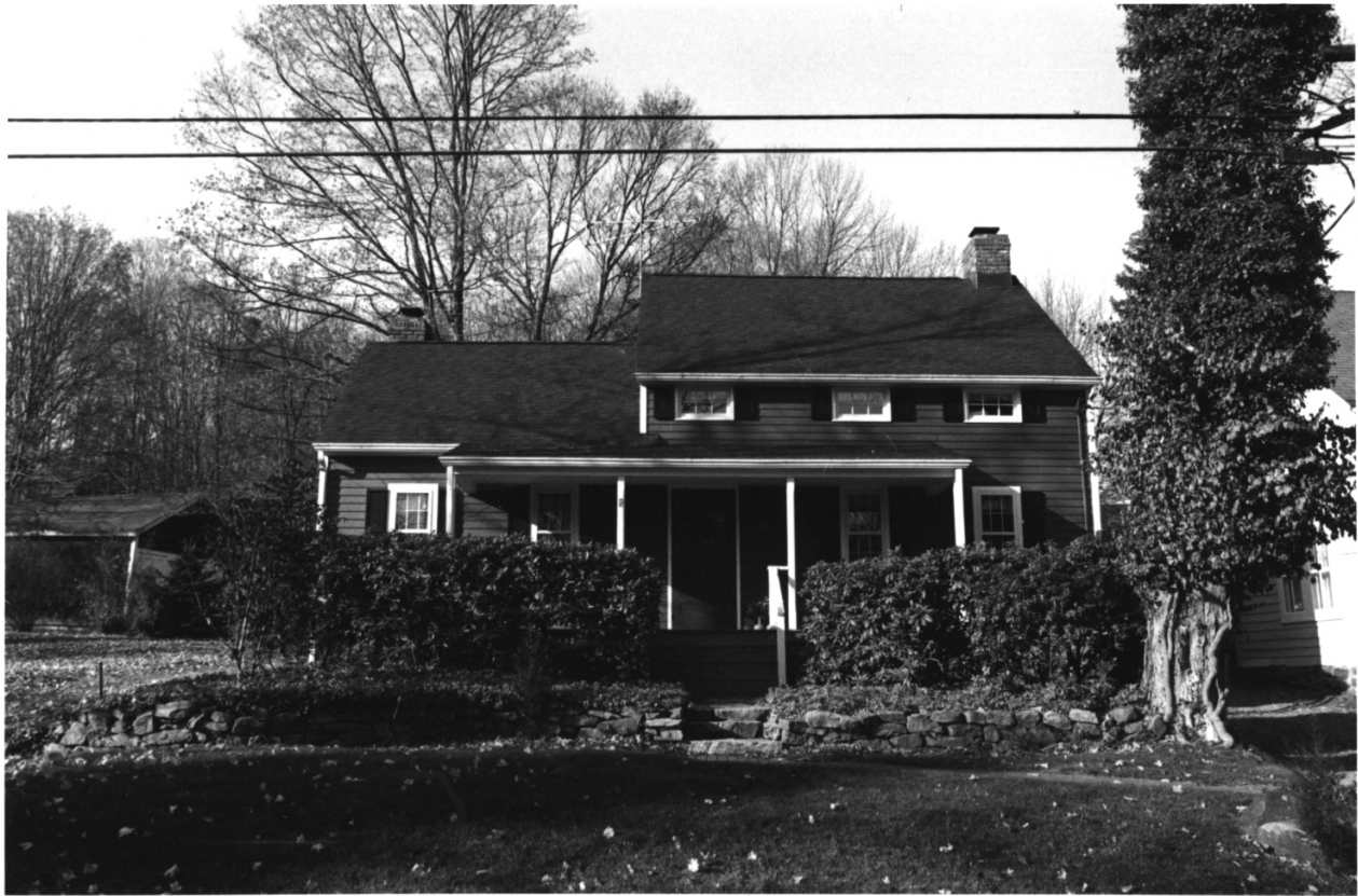
BROOKSIDE HISTORIC DISTRICT 034/027 PHOTO 21 OF 47
