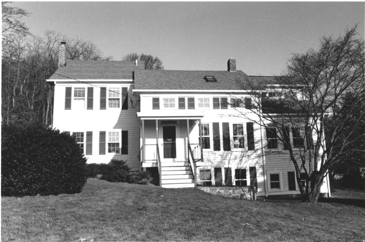
BROOKSIDE HISTORIC DISTRICT 034/027 PHOTO 4 OF 47
