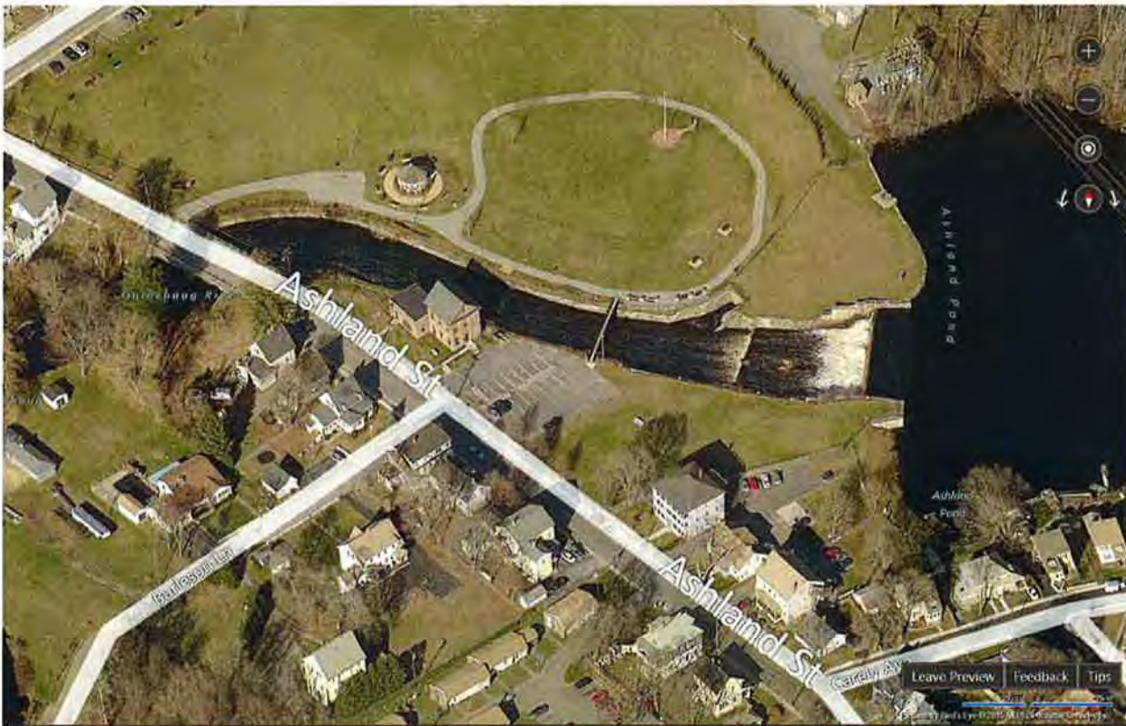
Aerial image showing location of former Ashland Mill Bridge and location of the new pedestrian bridge (source: Bing.com, November 2015).
