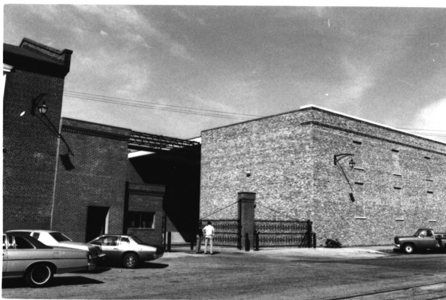
6. View of same entrance facing Northwest. New building on right.
