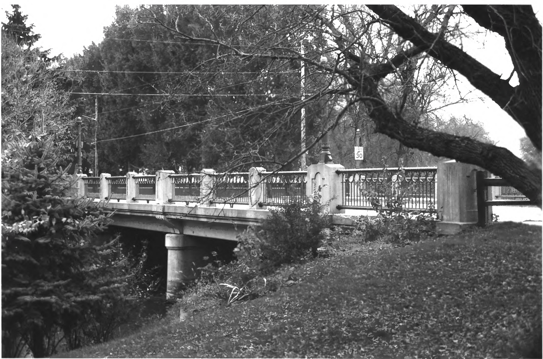
Bridge no. 5151 Mn Highway 19 over Redwood River, Marshall Lyon Co., Mn 012684-13
