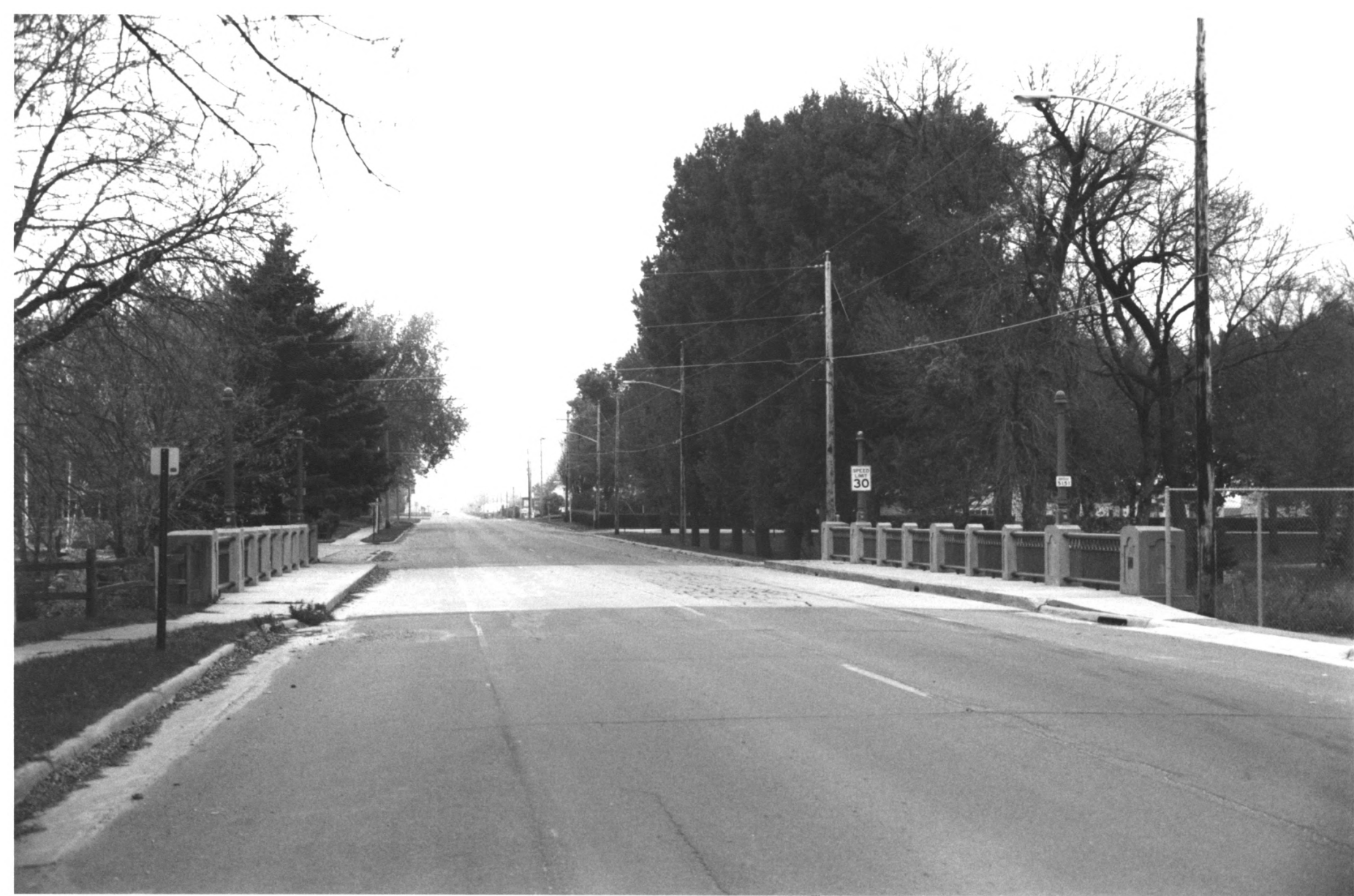
Bridge No. 5151 Mn Highway 19 over Redwood River, Marshall Lyon Co., Mn
