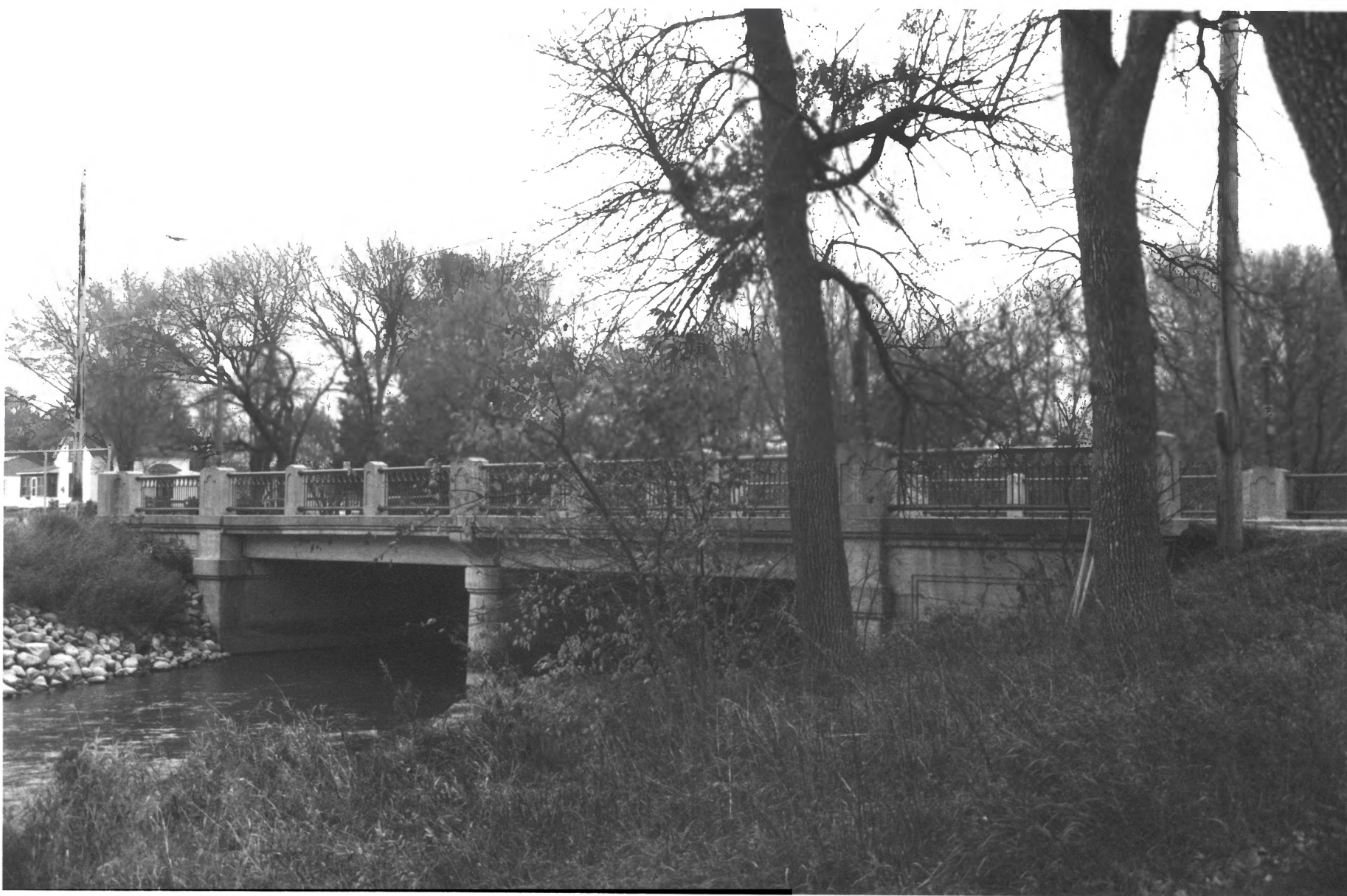
Bridge no. 5151 Mn Highway 19 over Redwood River, Marshall Lyon Co., Mn 012684-17
