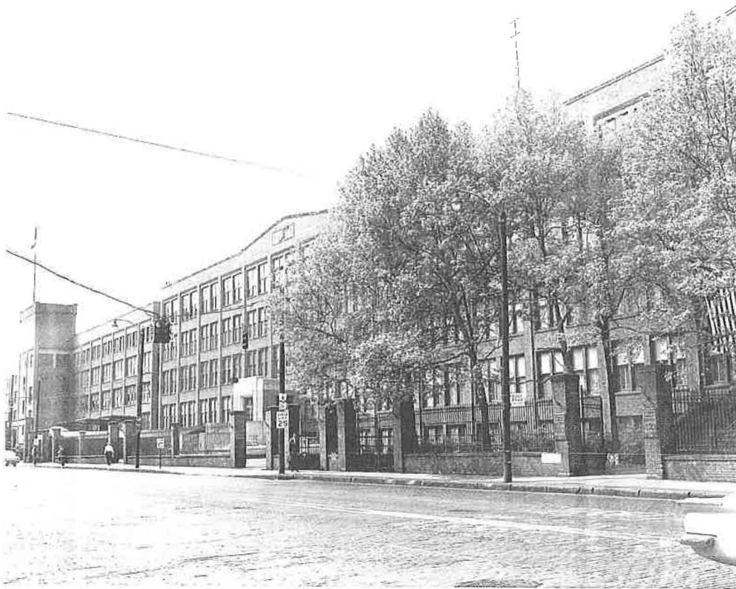
Images Courtesy of the University of Akron, Goodyear photograph files Goodyear Plant No. 1 Circa 1950, East Market Street looking south west.
