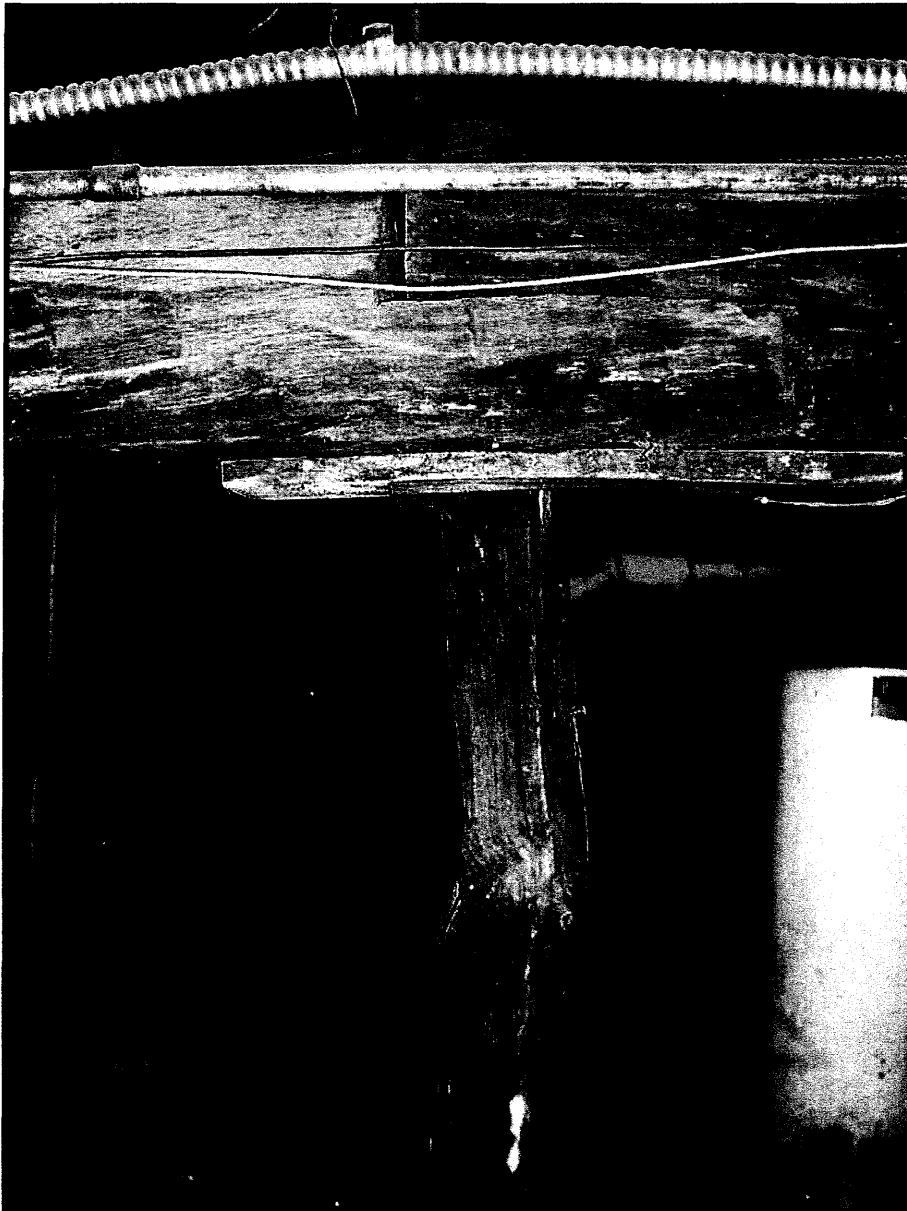
Image 11: Basement "Summer" beam, typical down length of building in both rooms.
