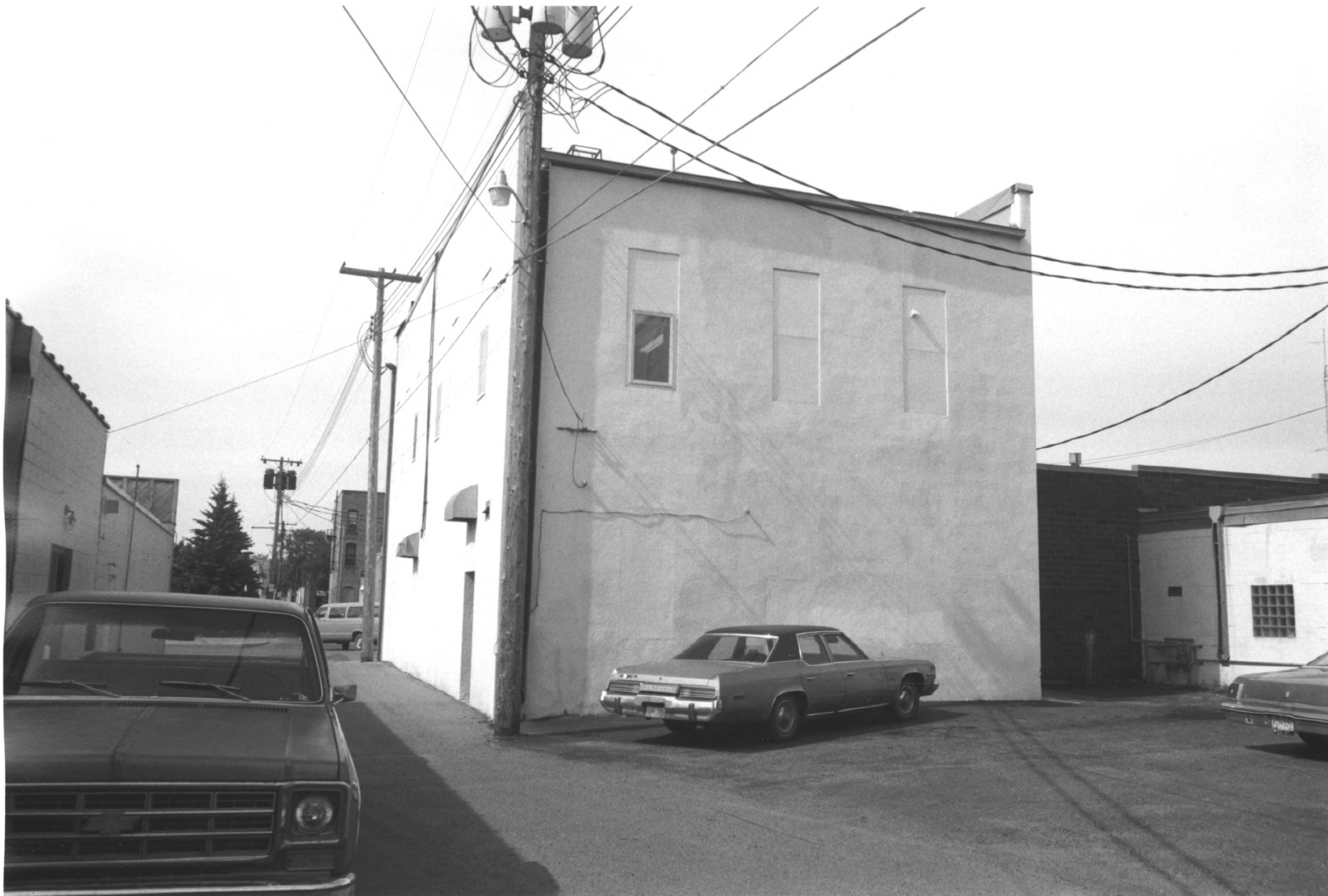
Wadena Fire and City Hall Wadena, MN 09326-7
