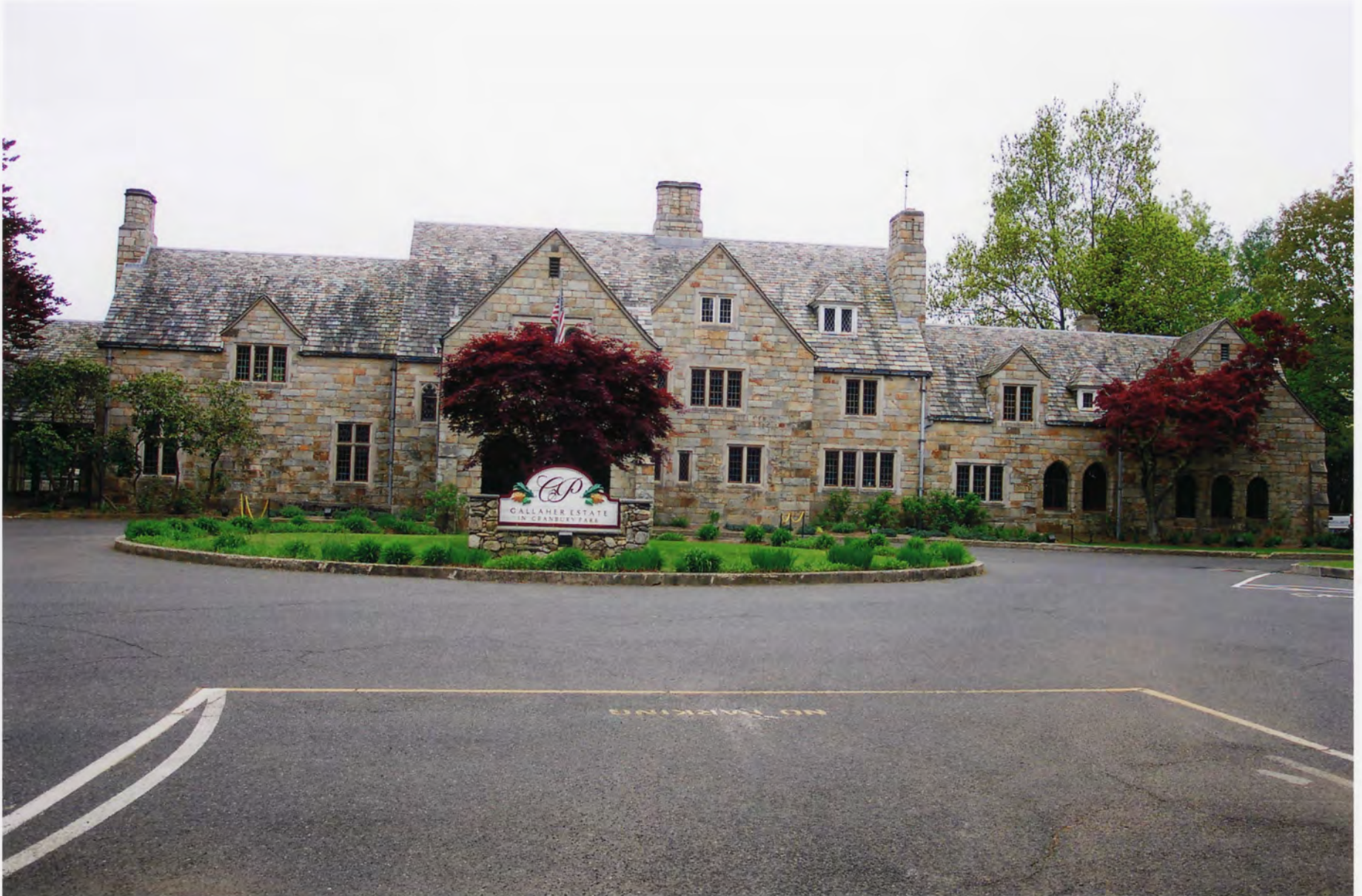
Photo # 1 Gallaher Estate-Cranbury Park, Norwalk, Fairfield County, CT Manor House, north elevation, view south.
