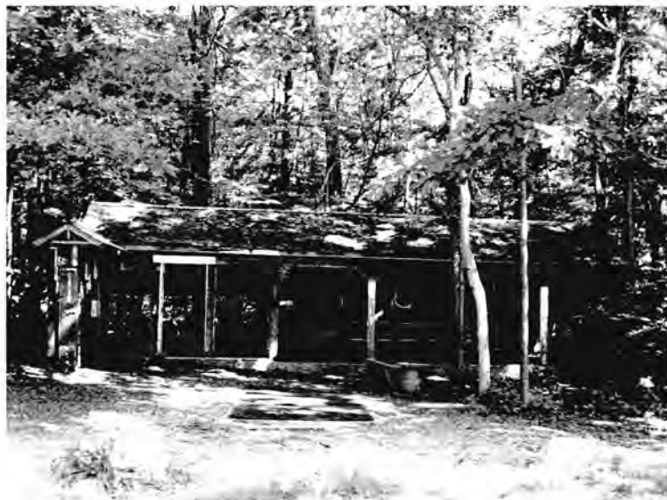
Photograph 30. Shed, south elevation, view north.
