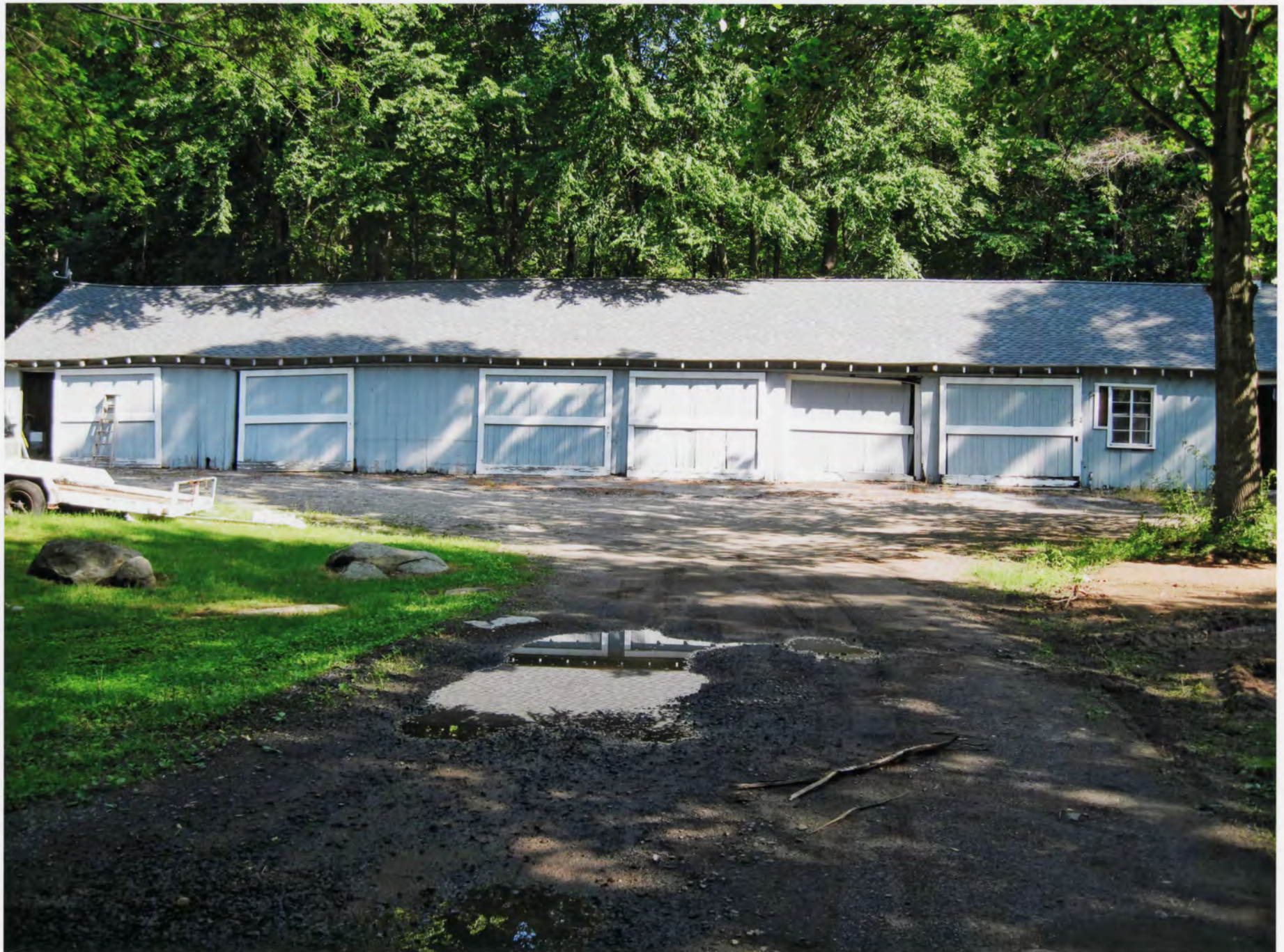
Photo # 34 Gallaher Estate-Cranbury Park, Norwalk, Fairfield County, CT Barn, south elevation, view north.
