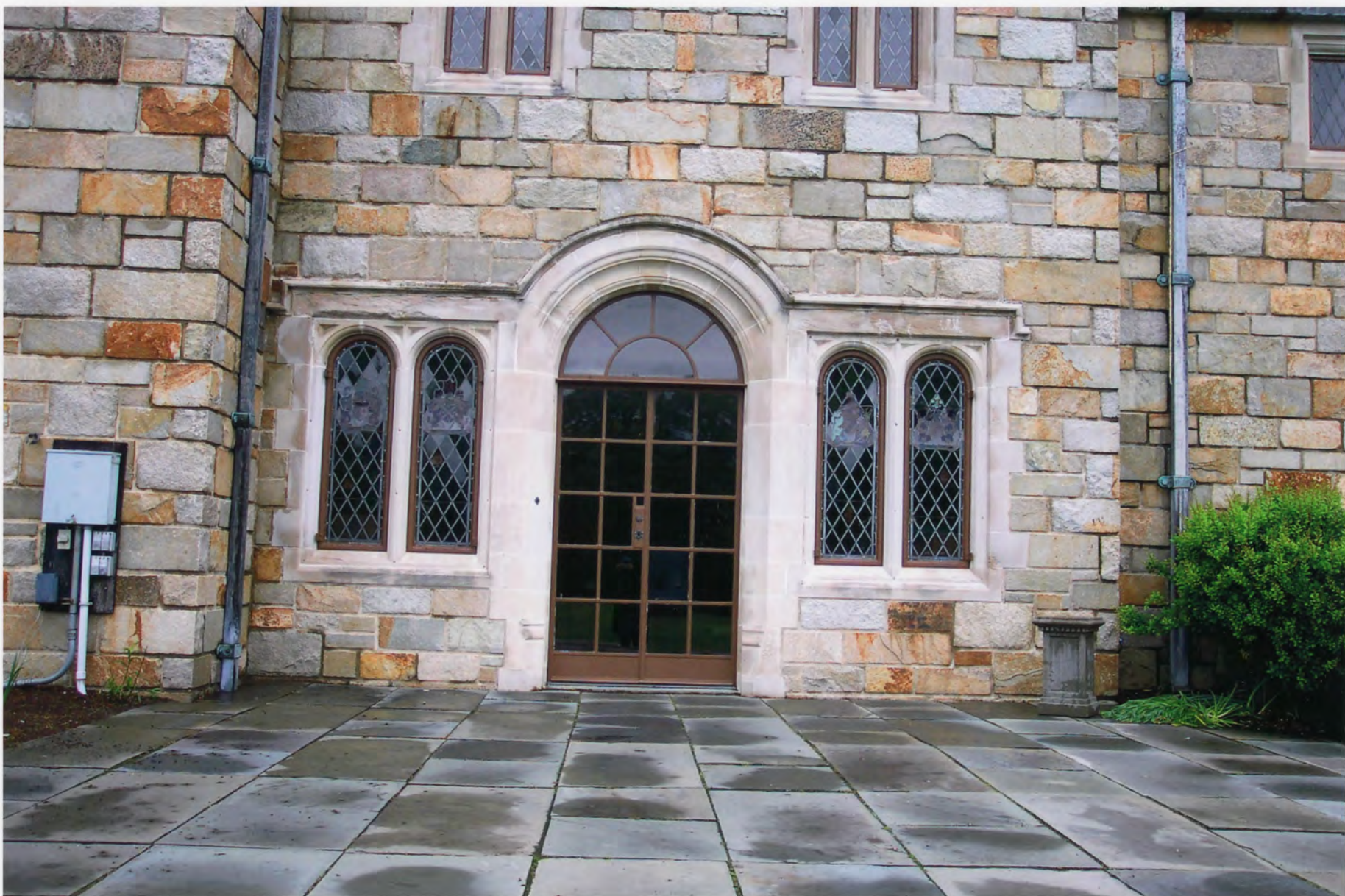
Photo # 5 Gallaher Estate-Cranbury Park, Norwalk, Fairfield County, CT Manor House, southern elevation, showing an arched doorway, flanked by paired arched casement windows, view north.
