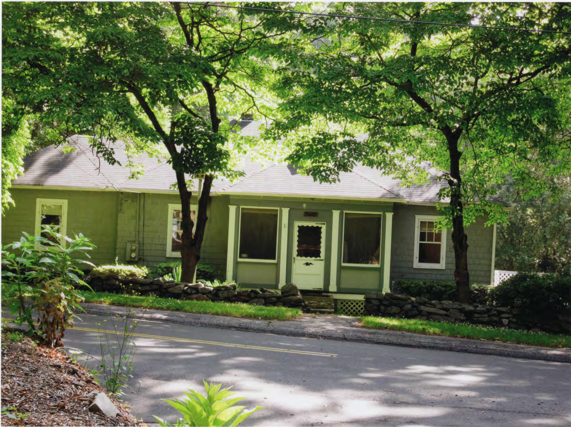
Photo # 33 Gallaher Estate-Cranbury Park, Norwalk, Fairfield County, CT Bungalow (gardener's house, west elevation, view east.
