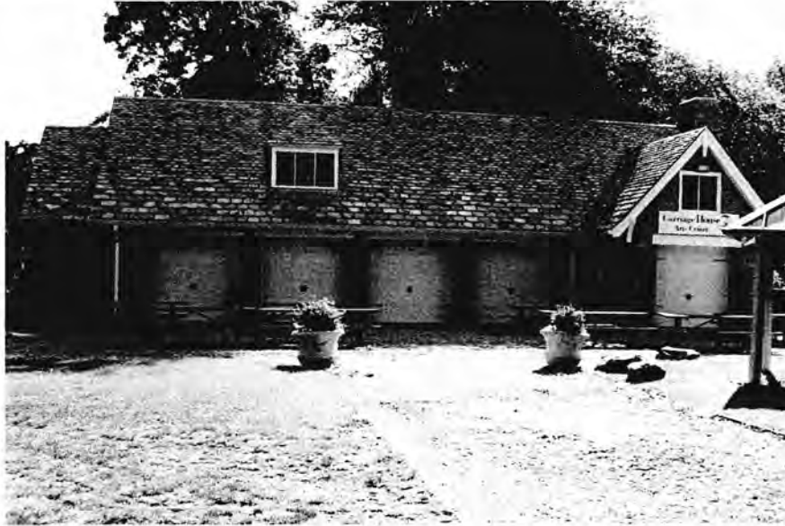
Photograph 25. Carriage House, west elevation, view east.
