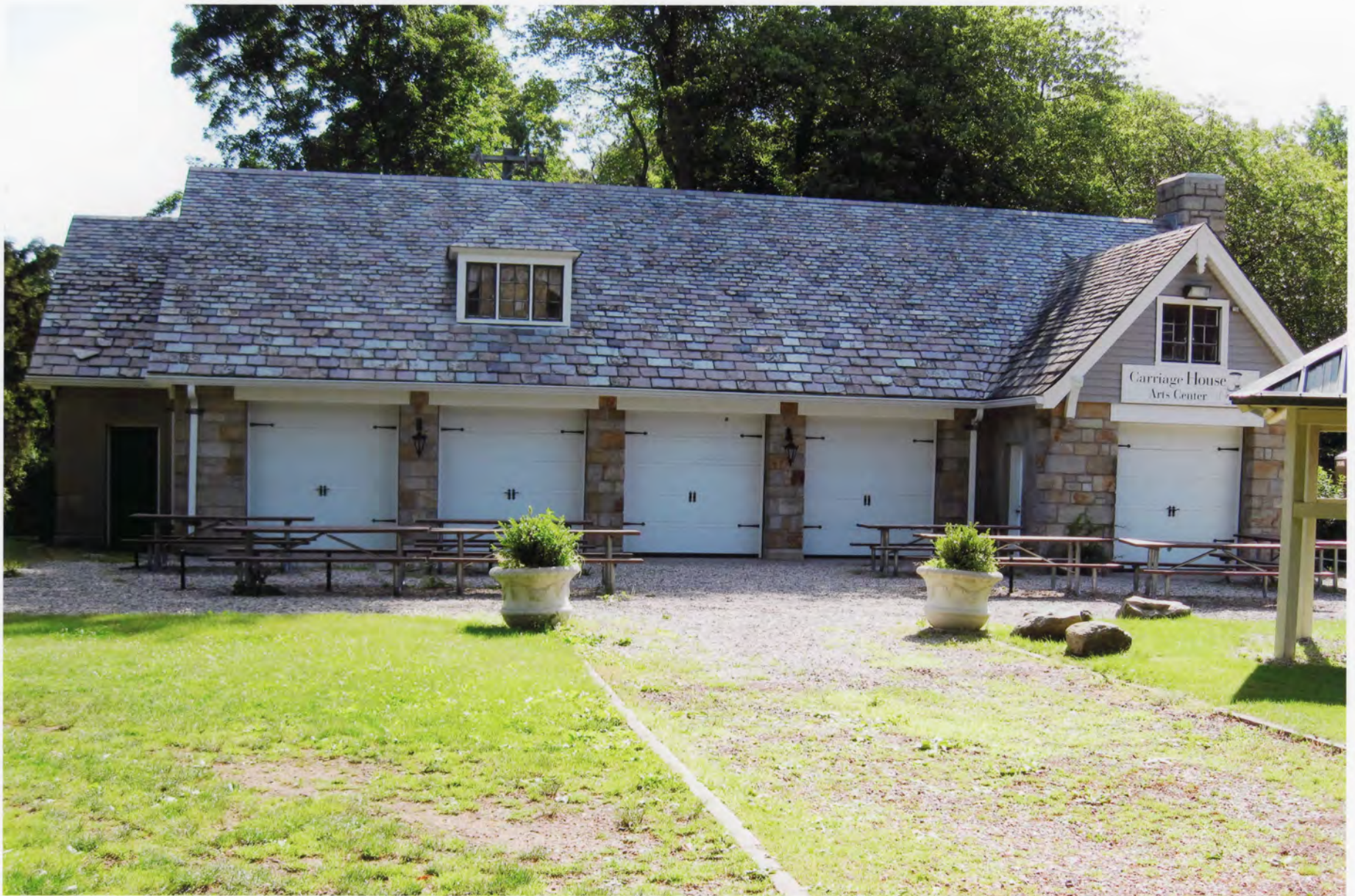
Photo #25 Gallaher Estate-Cranbury Park, Norwalk, Fairfield County, CT Carriage House, west elevation, view east.
