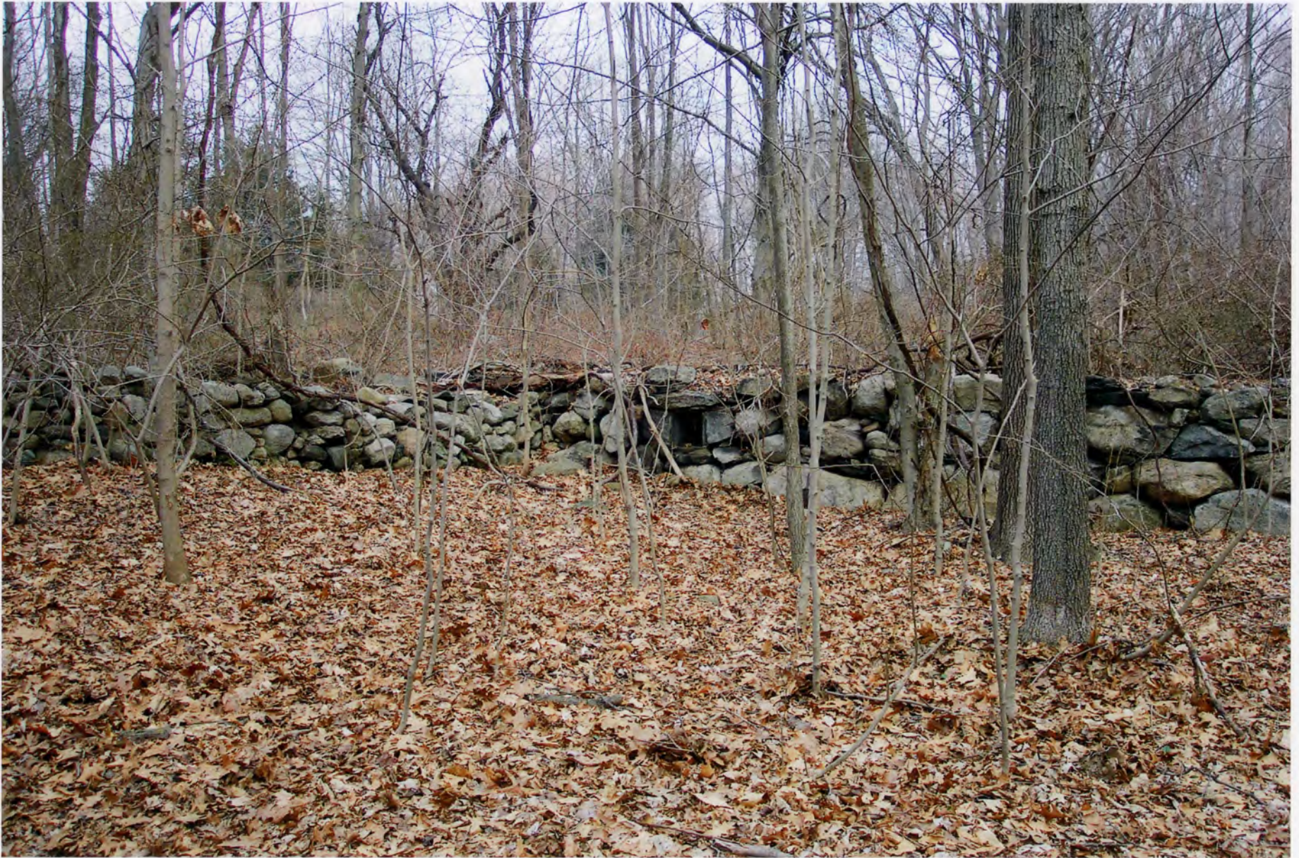
Photo # 24 Gallaher Estate-Cranbury Park, Norwalk, Fairfield County, CT Stone wall, east to west, view south.
