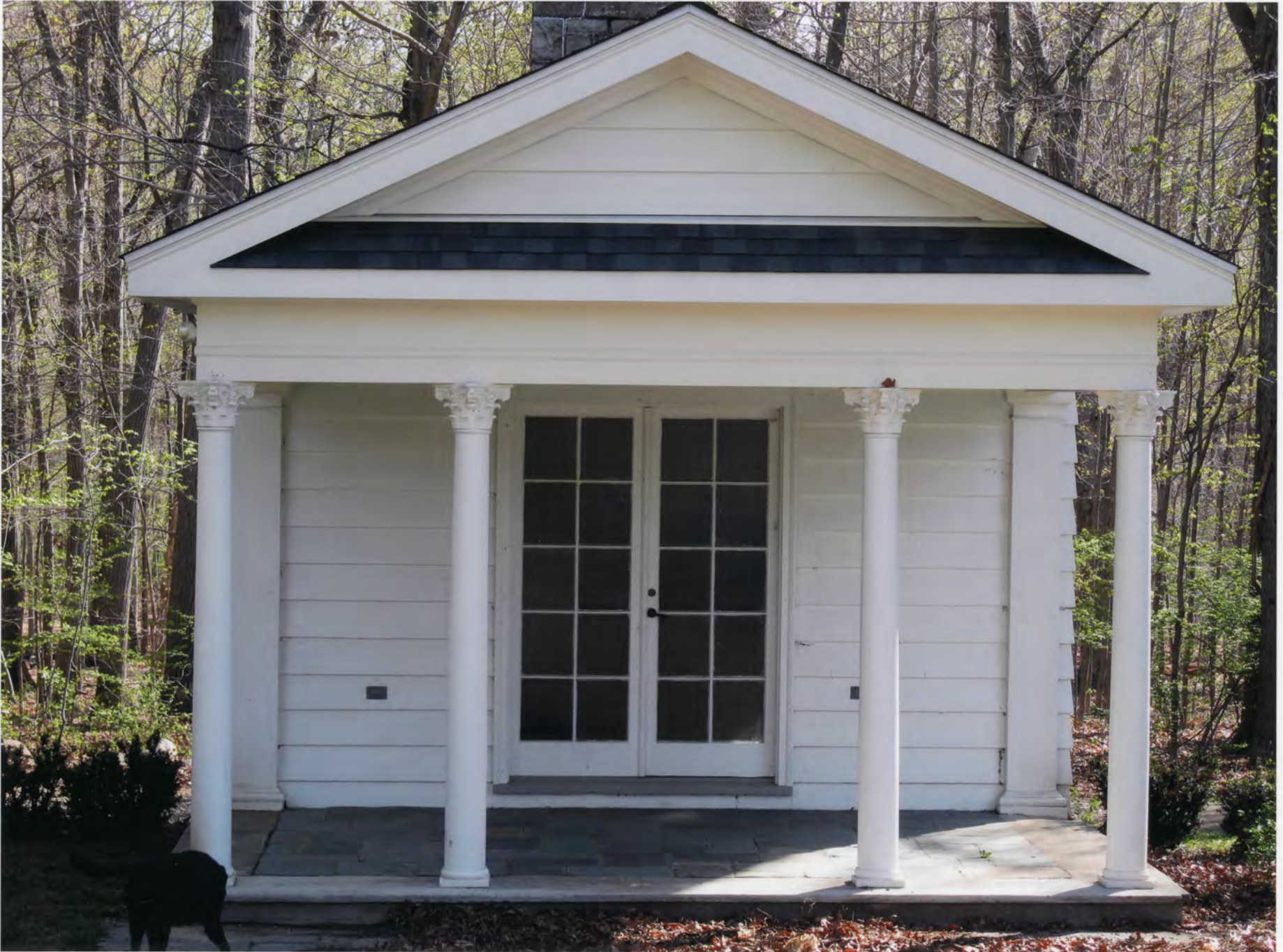
Photo #27 Gallaher Estate-Cranbury Park, Norwalk, Fairfield County, CT Tea house, exterior, west elevation, view east.
