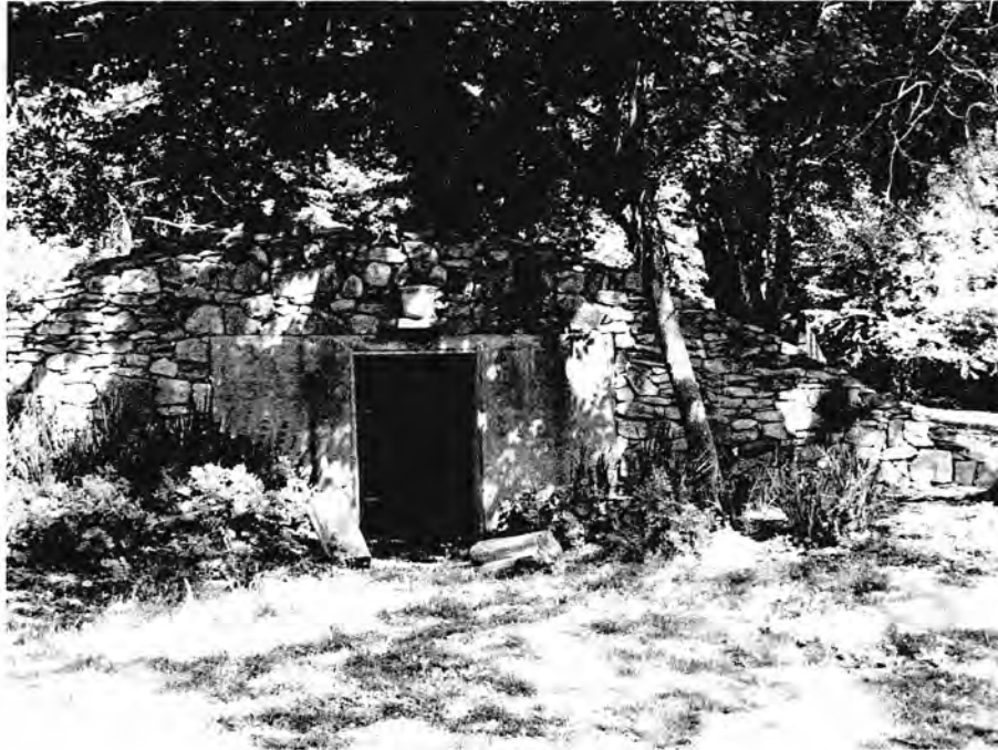
Photograph 31. Underground shelter, south elevation, view north.
