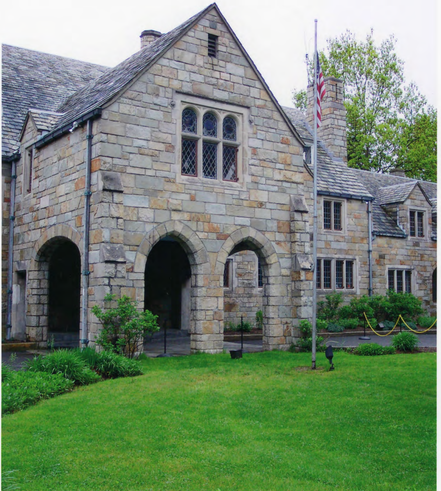
Photo # 2 Gallaher Estate-Cranbury Park, Norwalk, Fairfield County, CT Manor House, north and east elevation, view southwest.
