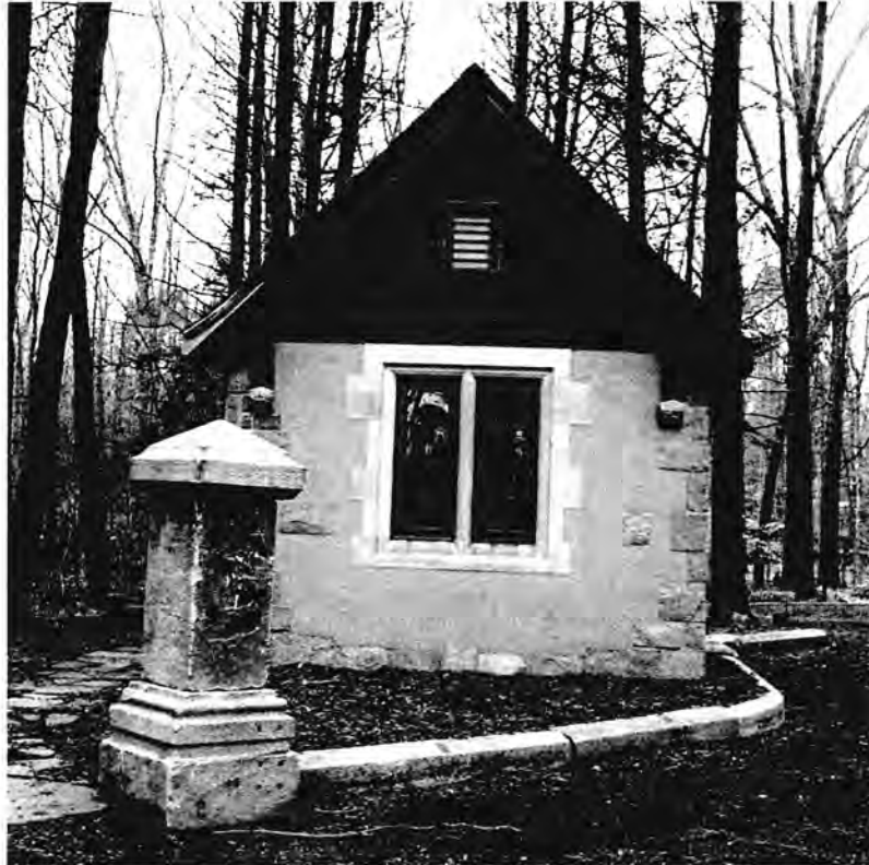
Photograph 29. Pump House, south elevation, view north.
