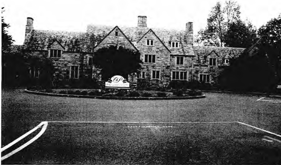
Photograph 2. Manor House, north and east elevation, view south.
