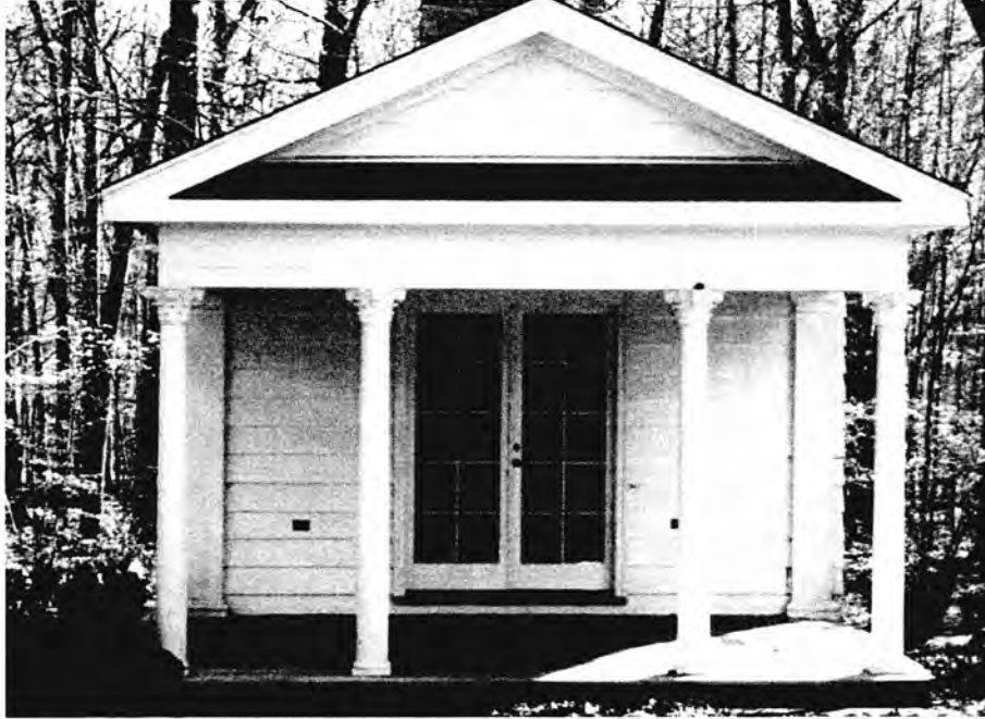
Photograph 27. Tea House, exterior, west elevation, view east.
