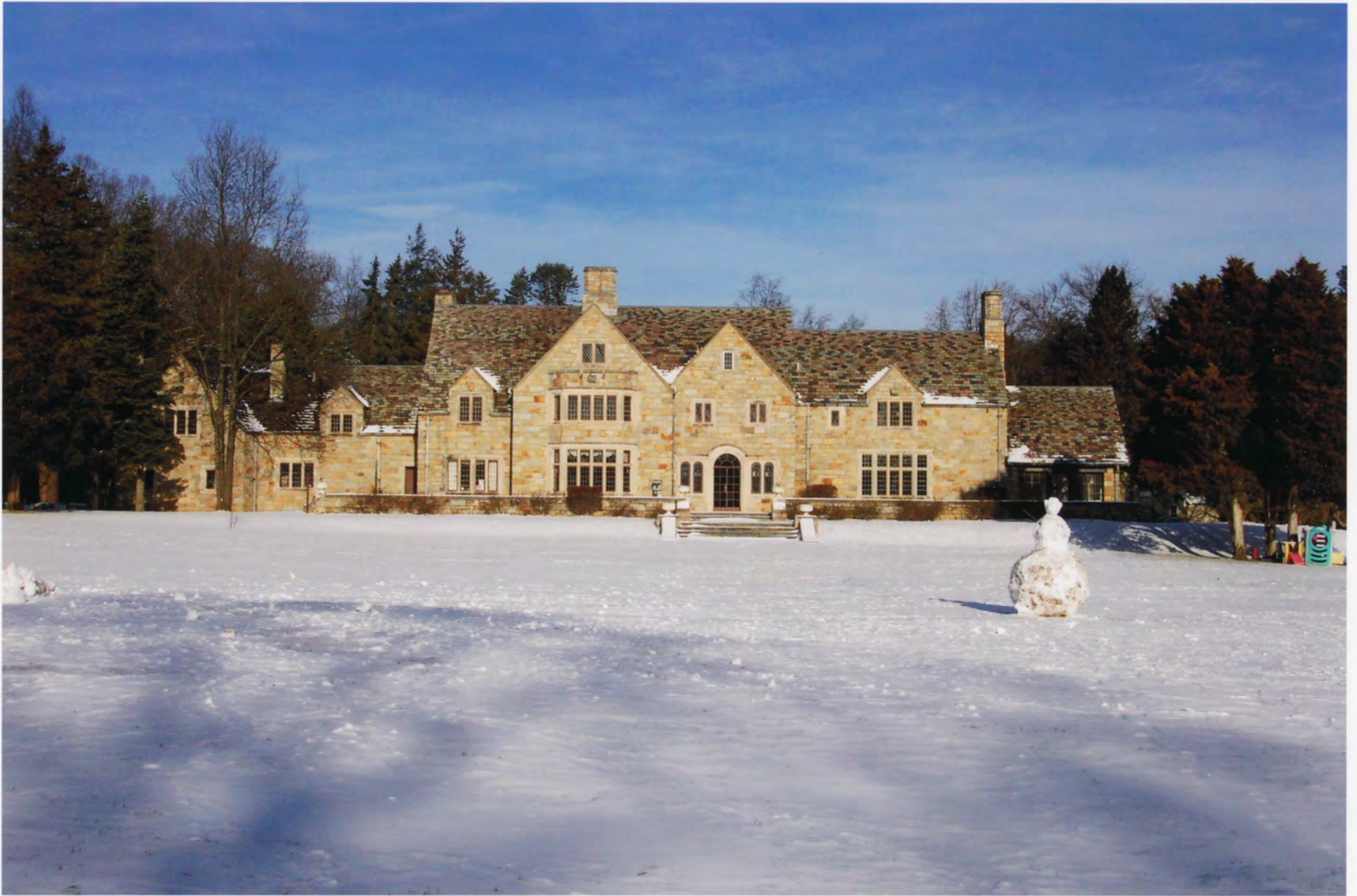
Photo # 4 Gallaher Estate-Cranbury Park, Norwalk, Fairfield County, CT Manor House, south elevation, view north
