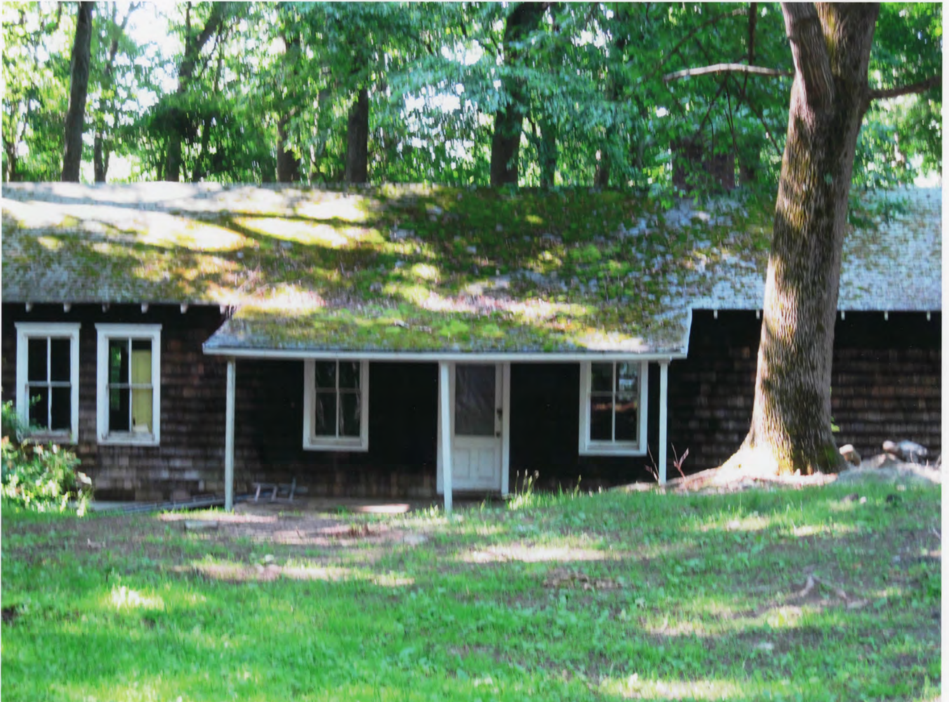
Photo # 32 Gallaher Estate-Cranbury Park, Norwalk, Fairfield County, CT Ranch house (bunkhouse), north elevation, view south.
