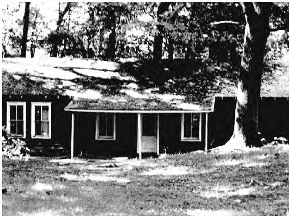
Photograph 32. Ranch House (Bunkhouse), north elevation, view south.
