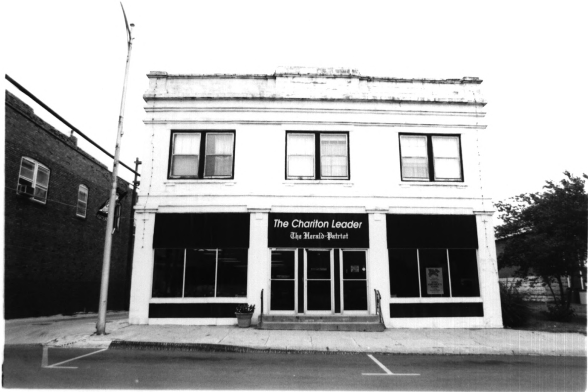
HERALD-PATRIOT BUILDING LUCAS COUNTY, IA photo #1
