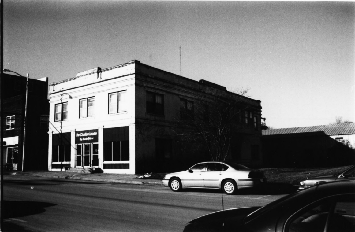
HERALD-PATRIOT BUILDING LUCAS COUNTY, IA Photo #4
