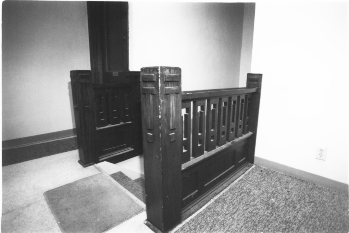
HERALD-PATRIOT BUILDING LUCAS COUNTY, IA PHOTO #6
