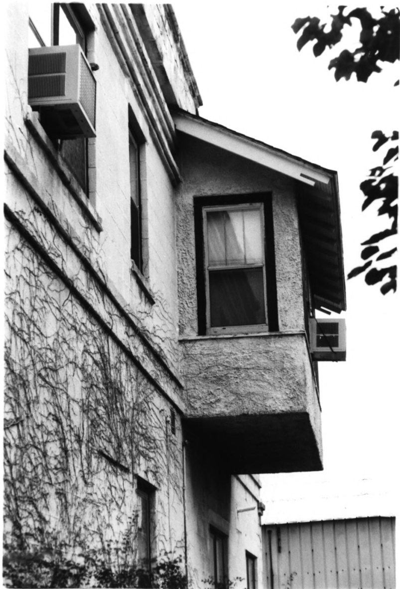
HERALD-PATRIOT BUILDING LUCAS COUNTY, IA Photo #5
