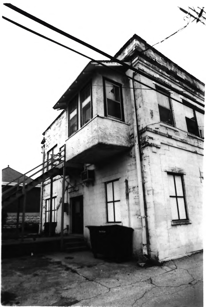
HERALD-PATRIOT BUILDING LUCAS COUNTY, IA Photo #3
