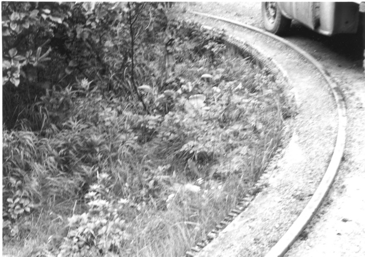
6. Panama mount for a 155mm gun, one of four at a battery on Buskin Hill, Fort Greely, Kodiak. These guns protected the naval base.
