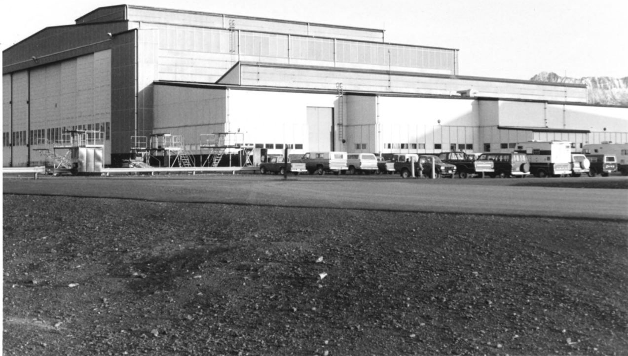
3. Engine overhead and aircraft maintenance building at former Kodiak naval base.
