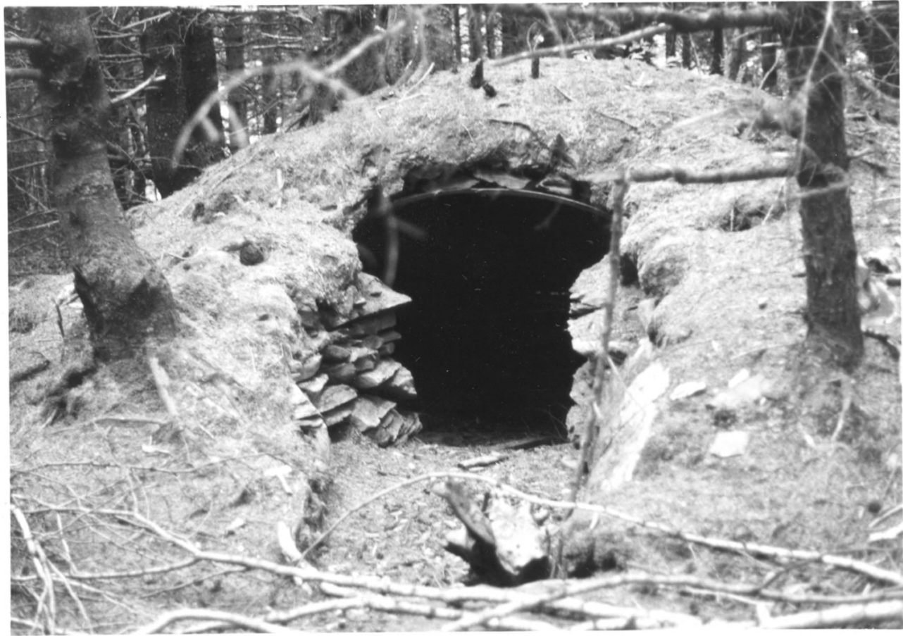
7. Personnel shelter, corrugated steel, rock, and earth. One of several in the vicinity of Artillery Hill, Fort Greely.
