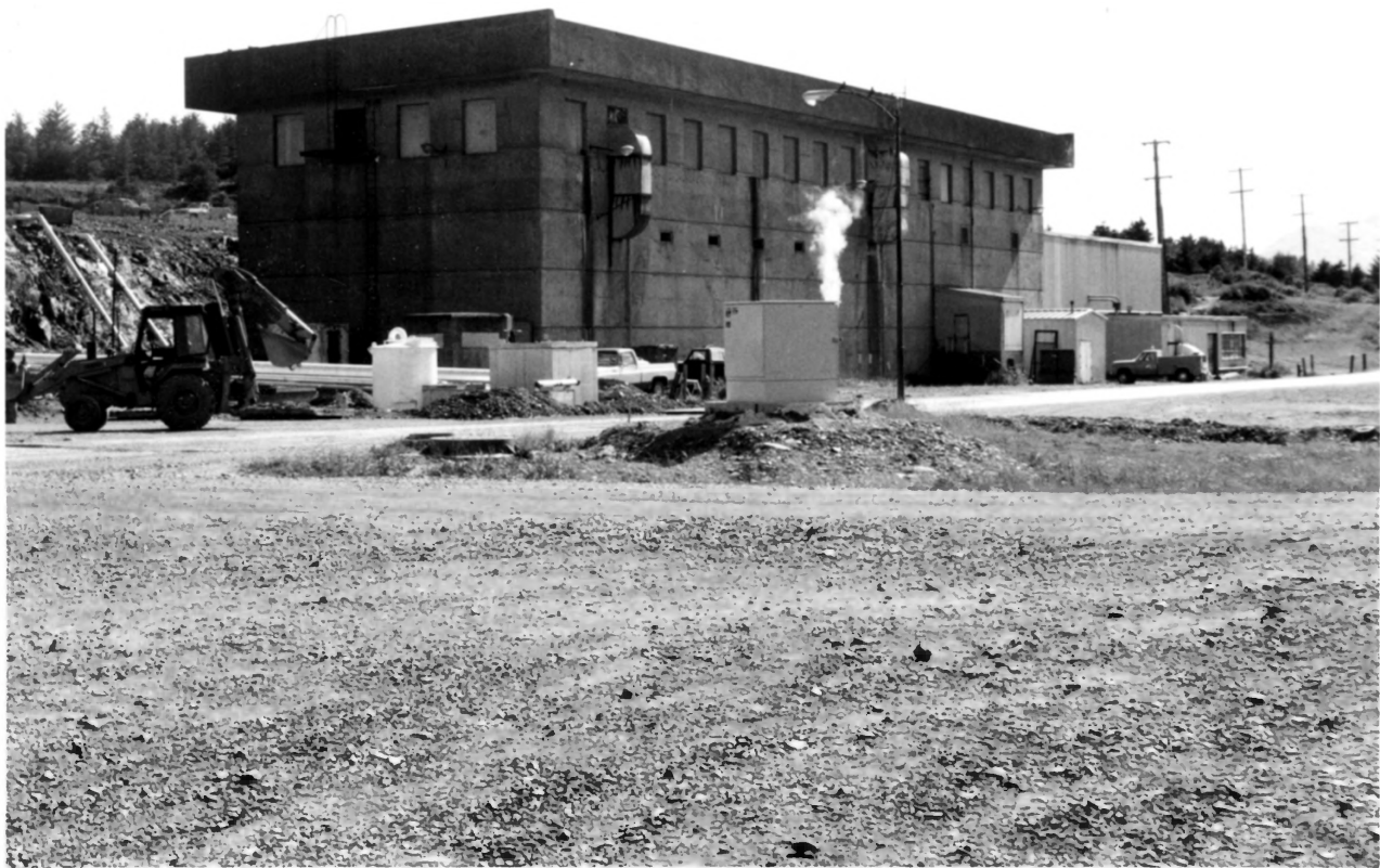
4. Bombproof power plant at Kodiak Naval Air Station.
