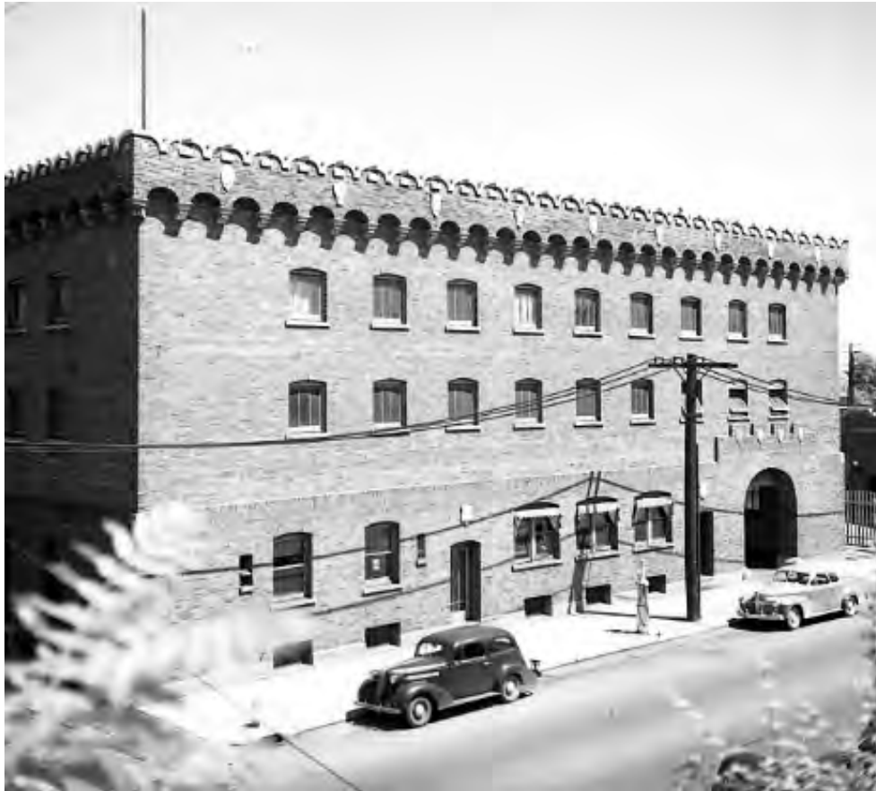
Figure 8: Photograph of the S. Zollinger Company Building looking southeast, 101 South Wayne Street, Piqua, ca. 1945 (Piqua Chamber of Commerce File, Piqua Public Library).
