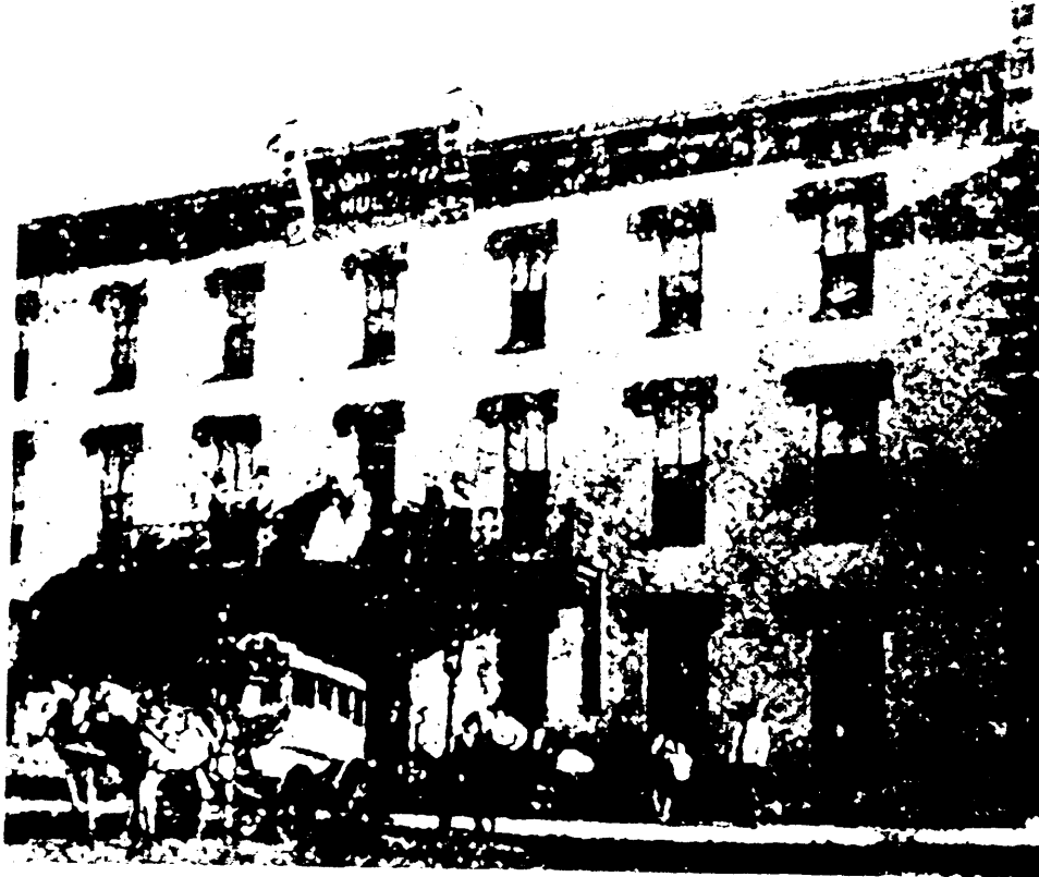
Front of The Bedford House (now Garland Hotel).
