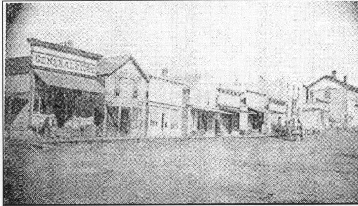
Figure 9: West Side of Davis Avenue, 700s block, Twining Corner (now 723-29 Davis) at upper right, view northwest from 7th, c.1885, 715 Davis, the only extant (and brick) building in this view, is shown just behind the parked wagon to the right
