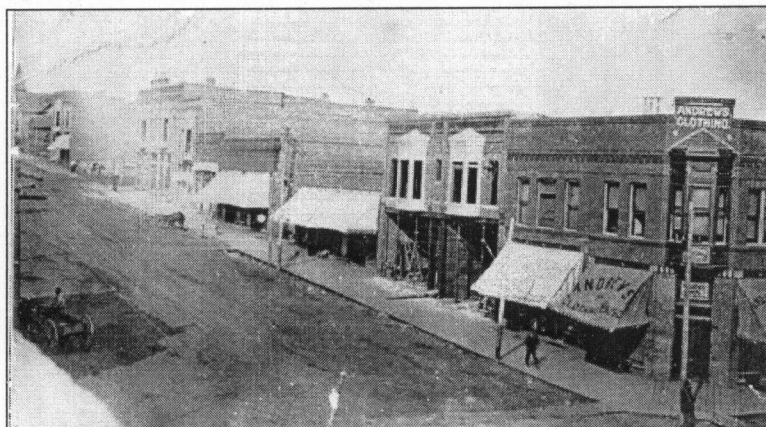
Figure 21: The newly rebuilt east side of Davis Avenue, 1897, looking northeast from 7 th Street, the Andrews Clothing occupies the new Beymer Building (700 Davis), note the Turner buildings (720, 722, 724-26 Davis)s, the Hefling and Mitchell buildings (804-06 Davis and the still vacant 800 Davis parcel) and the belfry on the United Brethren Church at upper left (Corning House of History)
