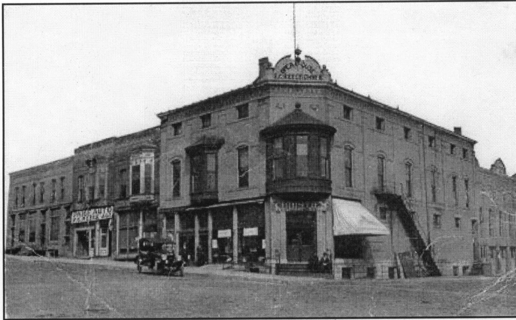
Figure 27: East side of Davis Avenue, viewed ca. 1902 from 8 th Street, showing the new Opera House and City Hall (far right), the Hefling and Mitchell Buildings (804-06 Davis), and the Park Hotel/Armory (non-extant), right to left (Corning House of History)
