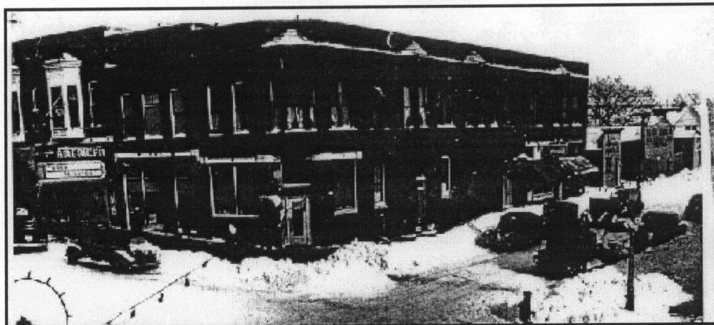
Figure 39: 700 Davis, ca. 1940, view northeast, note movie theater (Lauvstadt Center Photo Collection)
