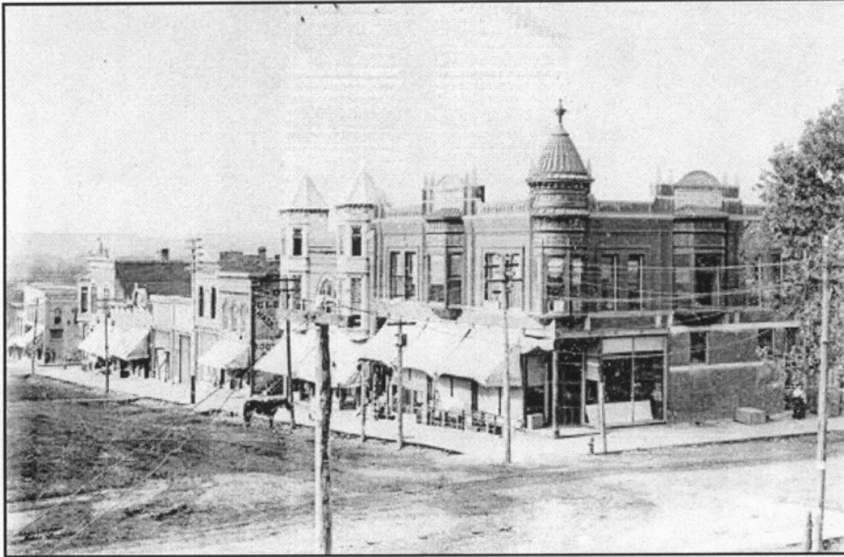
Figure 17: Repairing the fire damage on the west side of Davis Avenue, 1896, note the boarded up windows on the Widner Building in the foreground, view southwest from atop ruins of the Johnson Hotel (Corning House of History)
