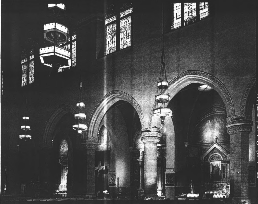
St. Paul the Apostle, New York City, Interior Historic American Buildings Survey on data return
