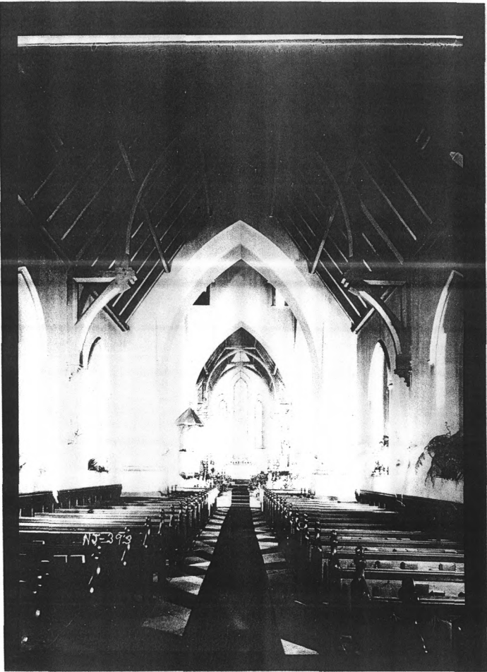
St. Mary's Church (new), Burlington, Interfor Historic American Building Survey, no date given
