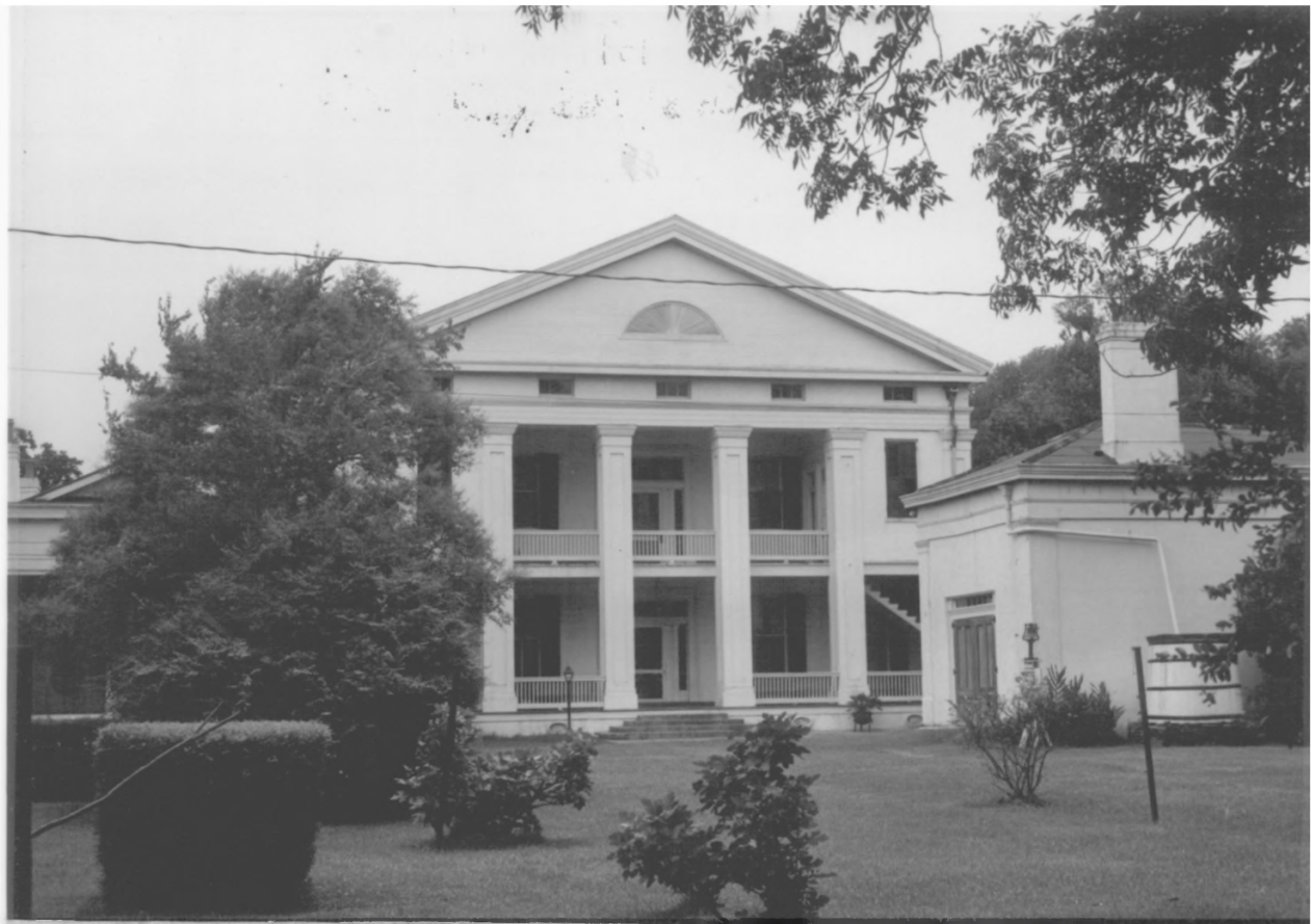
Rear (northeast) elevation of Main house; kitchen at right -- 1973
