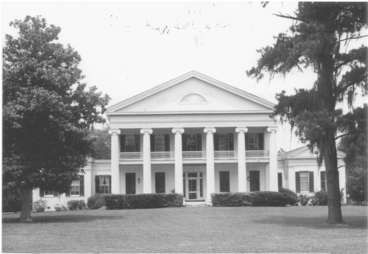
Front (southwest) elevation of Main house -- 1973
