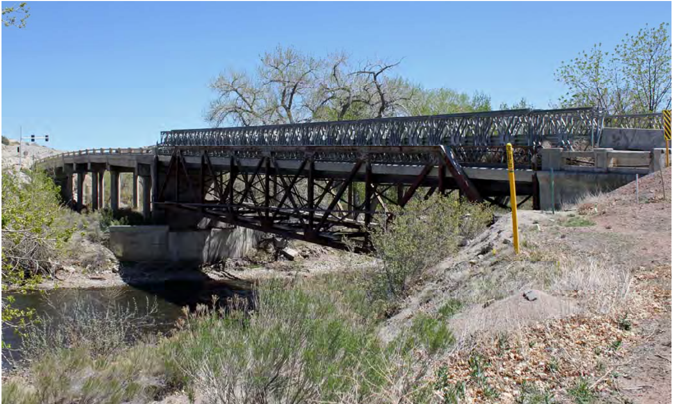
Bridge as seen in 2012, looking northwest, photo by Jeffrey Beal, https://en.wikipedia.org/wiki/File:Portland_Bridge.JPG (accessed 30 August 2017). A temporary bridge structure was placed over the historic bridge as part of an emergency repair, prior to eventual complete replacement in 2014.
