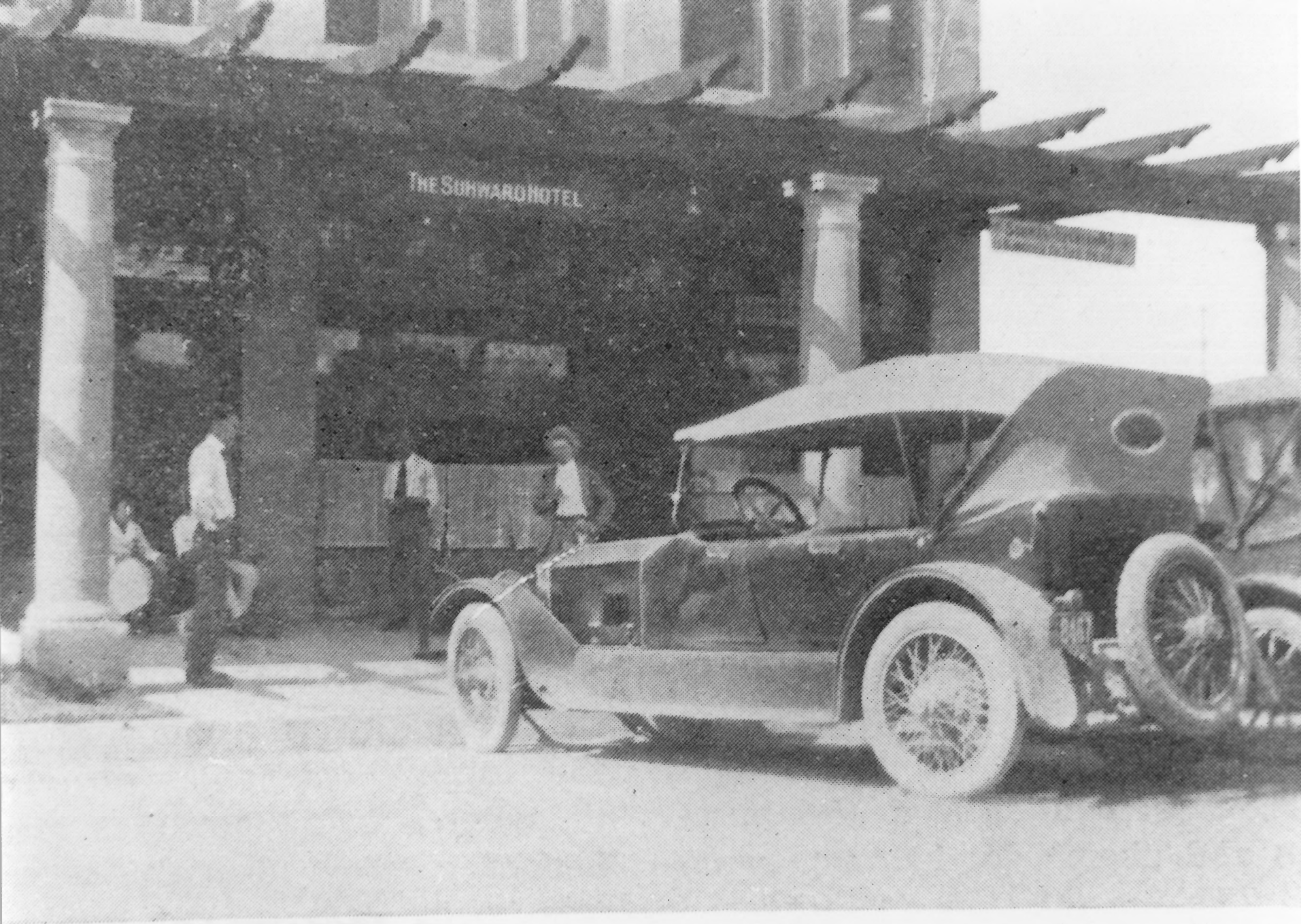
Scene in Front of the Suhward Hotel, Chandler.
