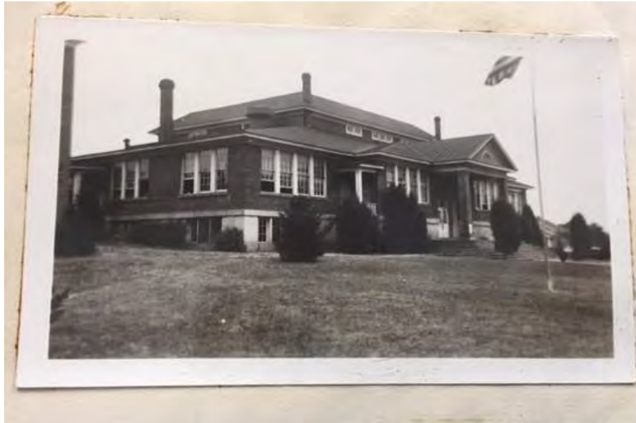
Figure 1: Madison Heights High School, Photograph from 1941 Engineering Report prepared for the School Board of Amherst County by W. D. Campbell & Son, Inc. of Lynchburg, Virginia
