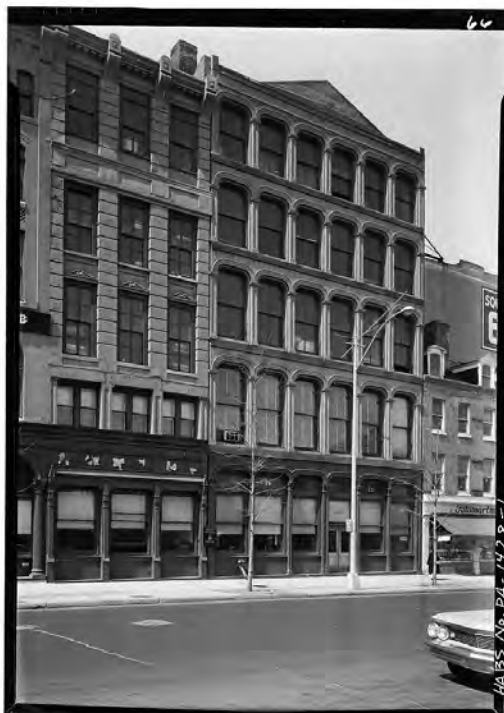
Figure 30 – Historic American Building Survey, 1961. Photo of the former Howell & Brothers' store at 12-14 S. 6 th Street shortly before its demolition (HABS PA-1428).
