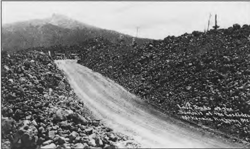
Completion of gravel surfacing in the lava beds near the summit in the mid-1920s; view east towards Black Crater. (Photograph, Collection of David Sell)
