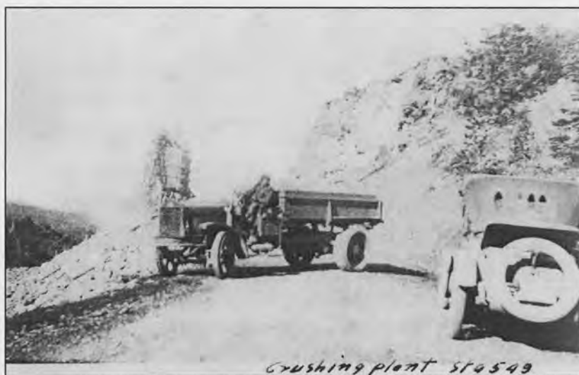
Crushing plant at Windy Point during road surfacing in the mid-1920s (USBPR Records).
