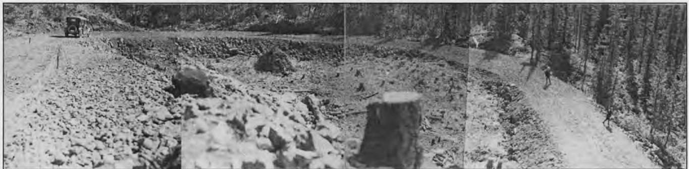
Construction of a loop on the Deadhorse Grade section in the early 1920s (USBPR Records).
