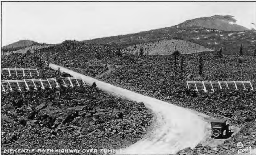
Snow fences near the summit in the mid-1920s; view to the north-west towards Belknap Crater from the location of Dee Wright Observatory. (Photograph, Collection of David Sell)
