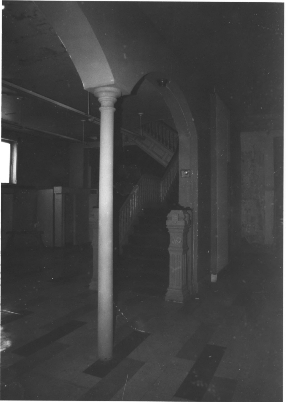
KIRSCHBAUM, RATHAEL, BLDG, RANDOLPH CO., IN #16
