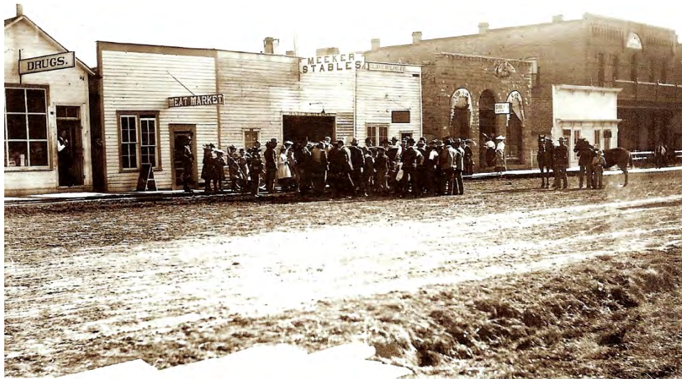
Figure 4: Buildings on the south side of the 500 block of Main Street, view to southwest, circa 1901, courtesy of Rio Blanco County Historical Society and White River Museum.
