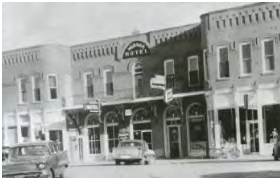
Figure 10: Meeker Hotel (560 Main Street, 5RB.985), view to south, circa 1955, courtesy of Denver Public Library, z-11990.
