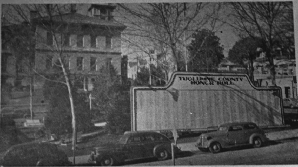
Tuolumne County Court House
