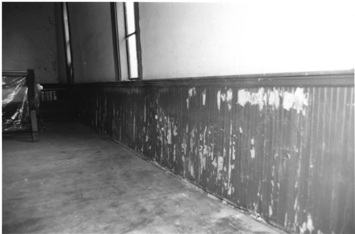
Manchester Cumberland Presbyterian Church Manchester, Coffee County, TN #10 of 15
