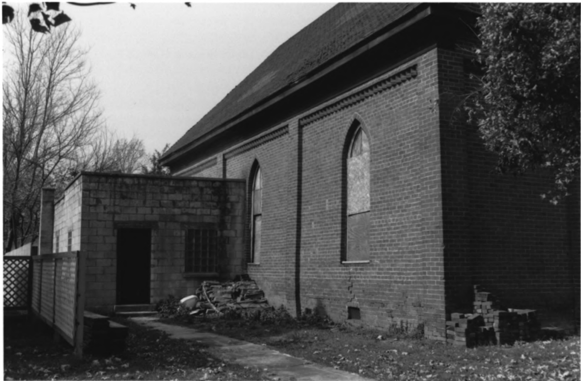
Manchester Cumberland Presbyterian Church Manchester, Coffee County, TN #6 of 15
