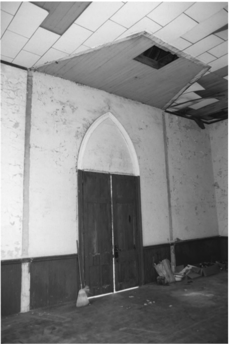
Manchester Cumberland Presbyterian Church Manchester, Coffee County, TN #8 of 15
