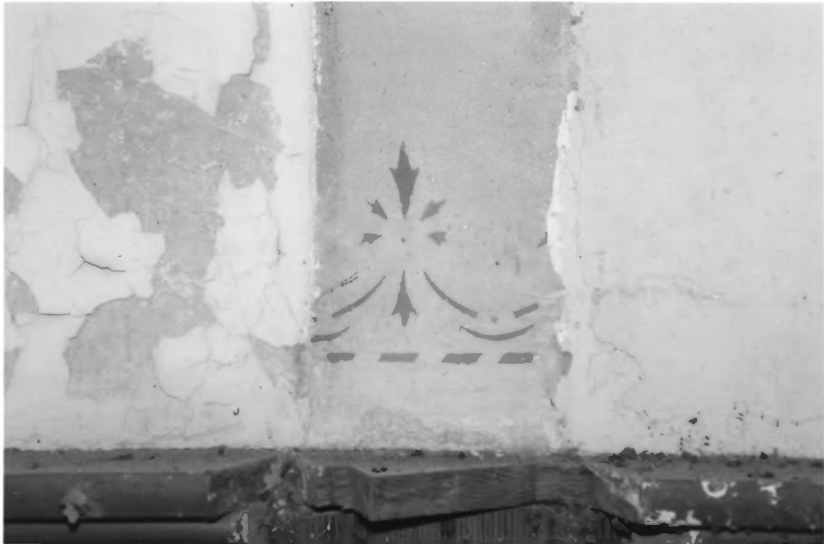
Manchester Cumberland Presbyterian Church Manchester, Coffee County, TN #9 of 15
