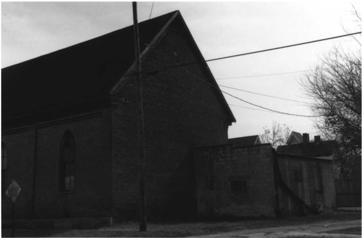
Manchester Cumberland Presbyterian Church Manchester, Coffee County, TN #5of15
