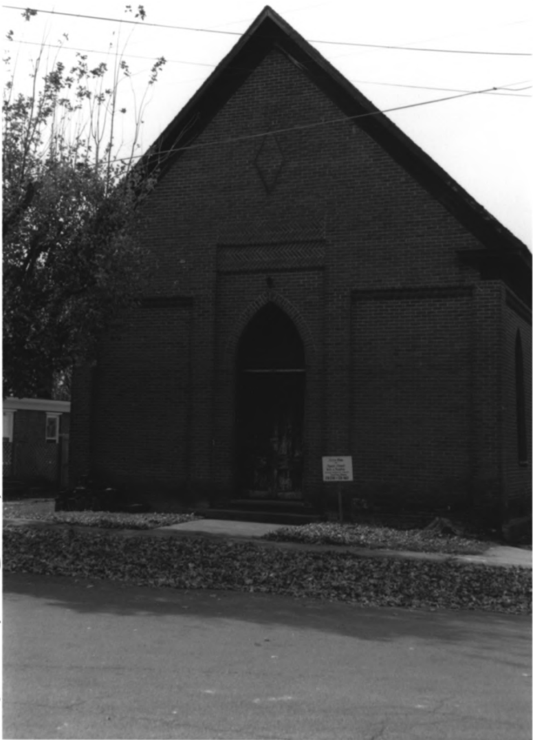
Manchester Cumberland Presbyterian Church Manchester, Coffee County, TN #1 of 15
