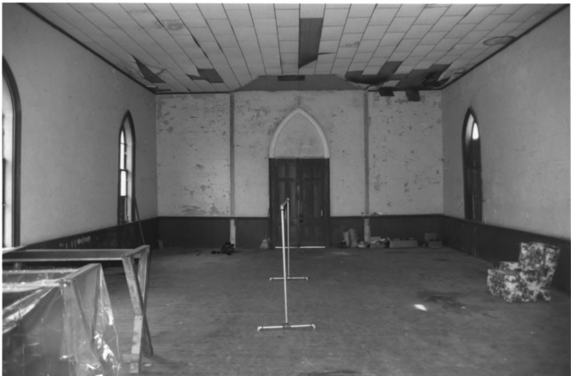
Manchester Cumberland Presbyterian Church Manchester, Coffee County, TN #7 of 15
