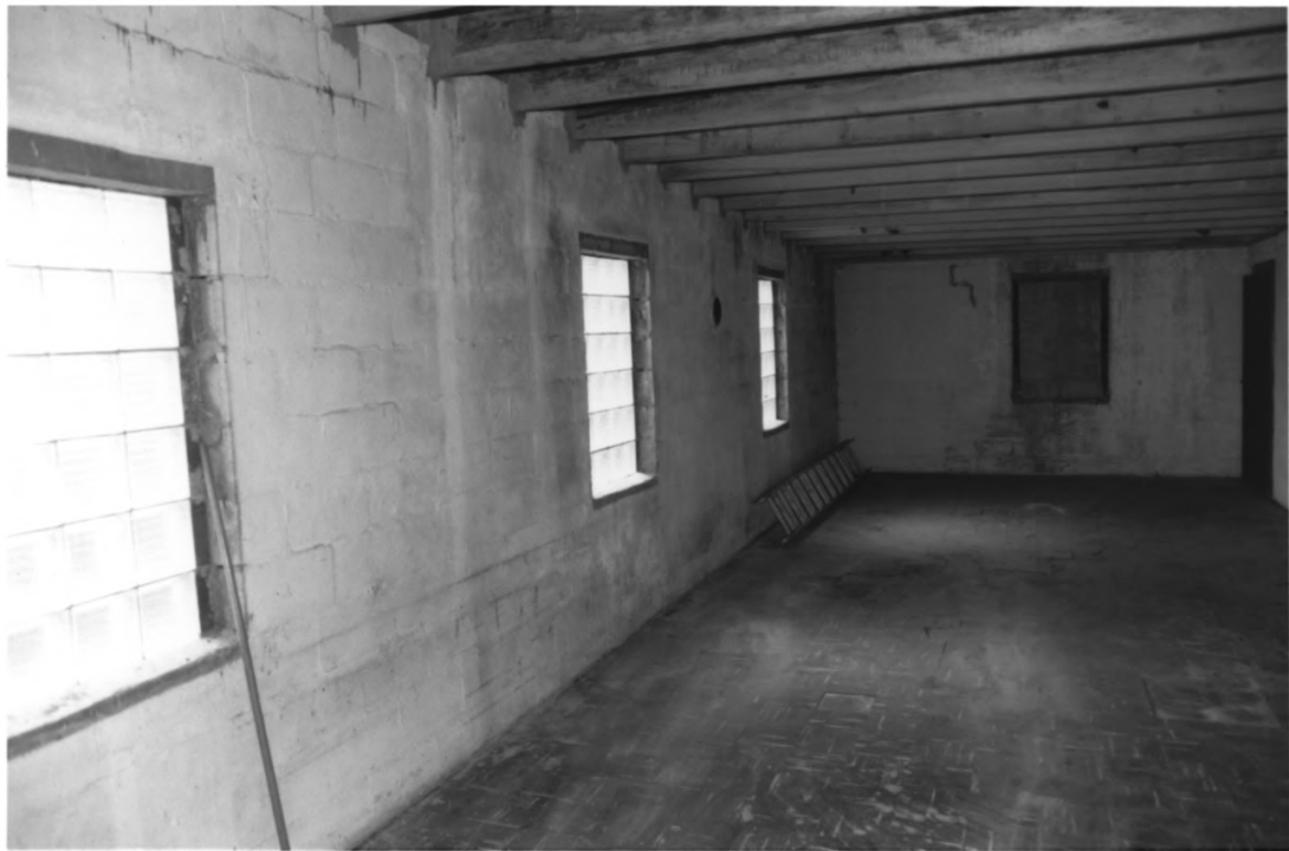
Manchester Cumberland Presbyterian Church Manchester, Coffee County, TN #15 of 15
