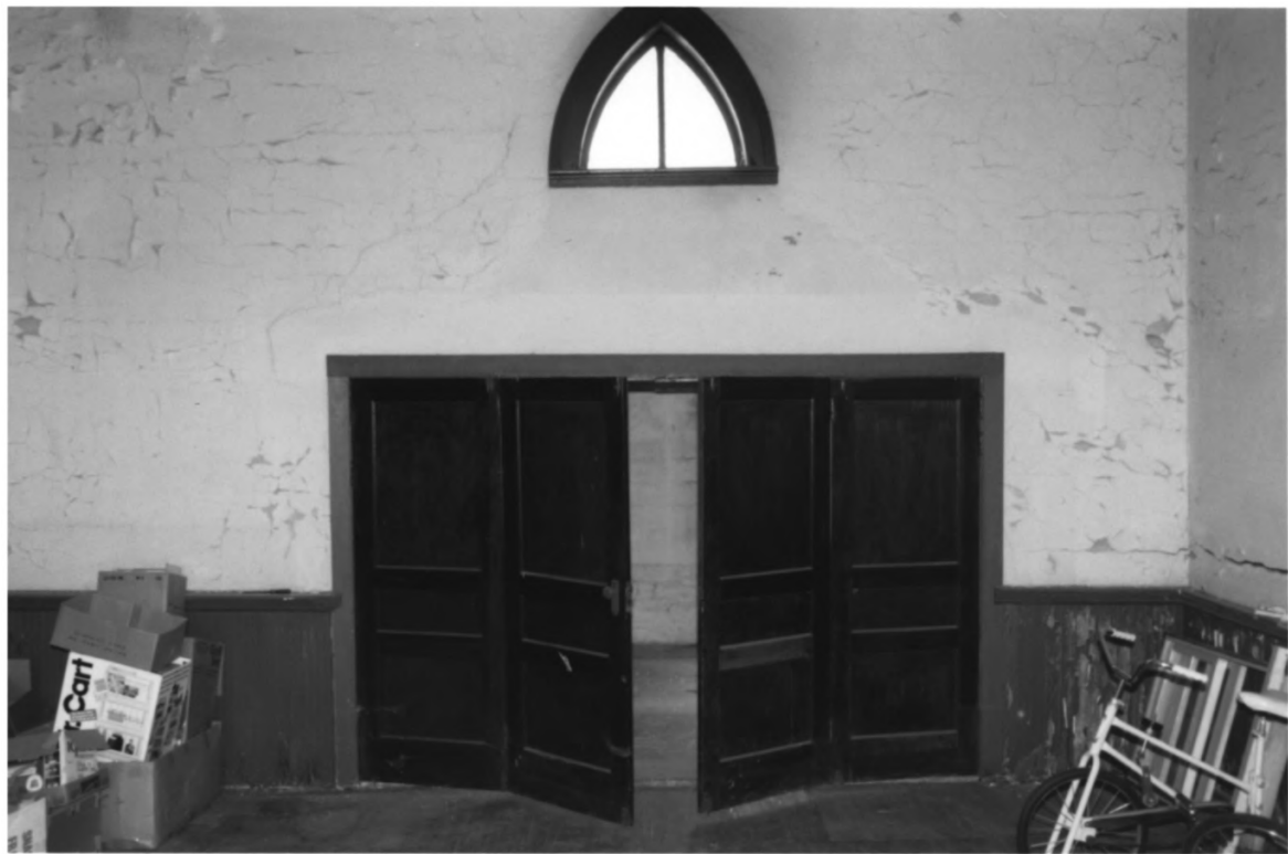
Manchester Cumberland Presbyterian Church Manchester, Coffee County, TN # 14 of 15
