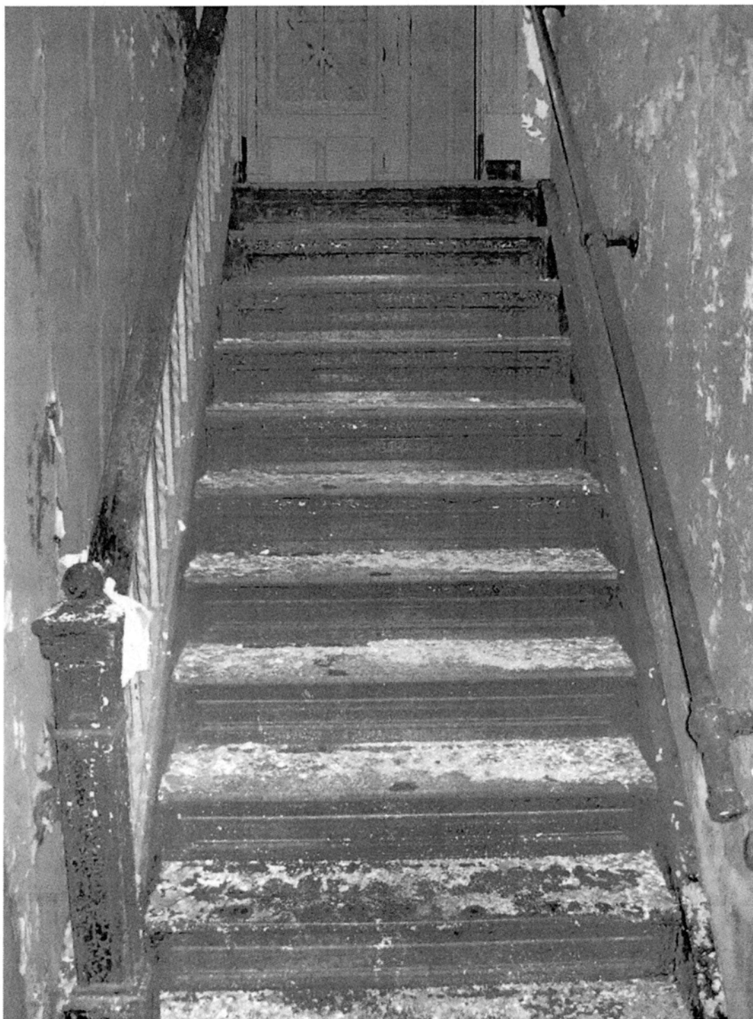
Basement-level stairs, showing stair, baluster, rail, newel post, and wall details. Camera facing west. Photograph 14 of 26.
