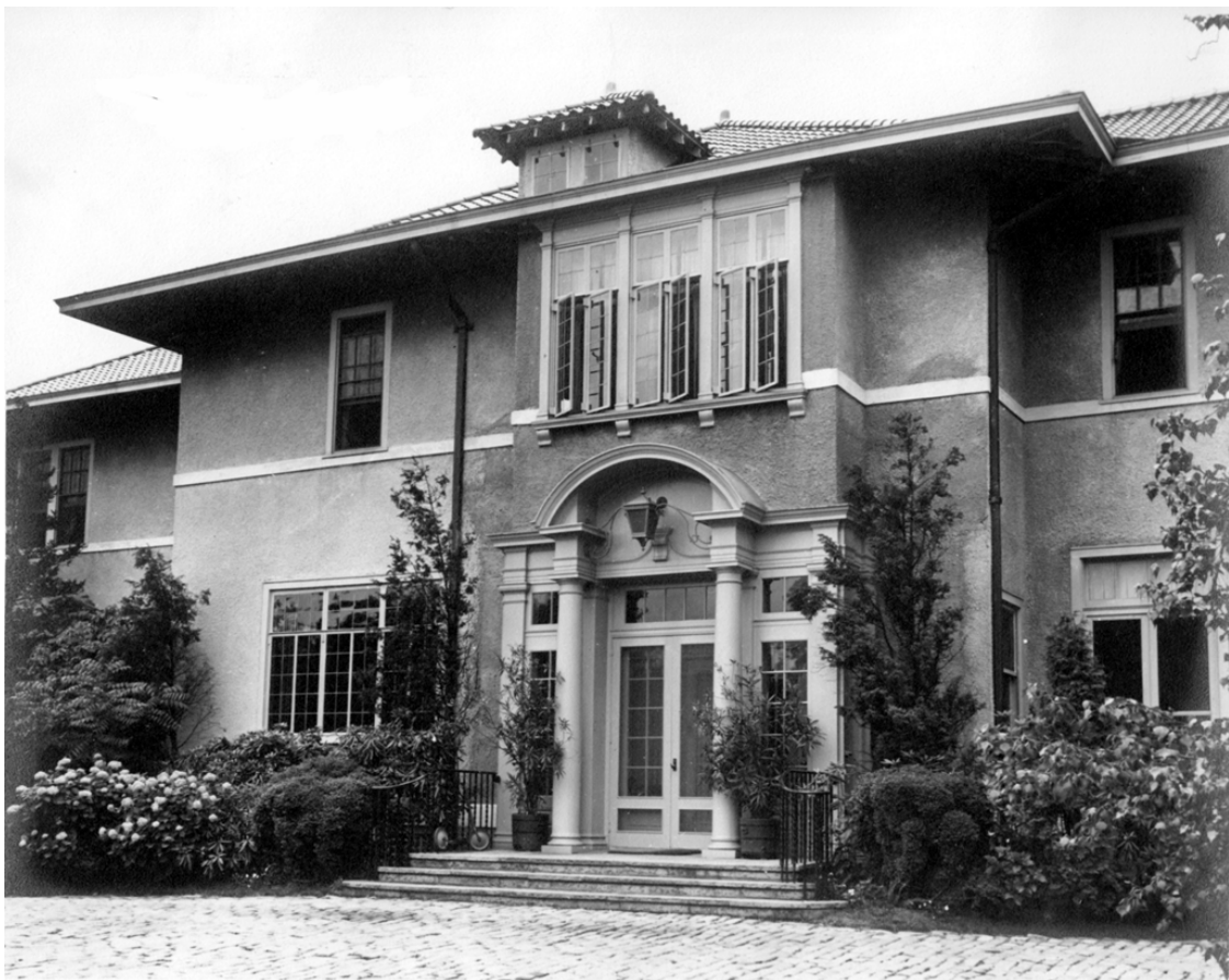
Figure 11. Schenck house (Land Hall), north façade, 1942 (NARA RG 178).
