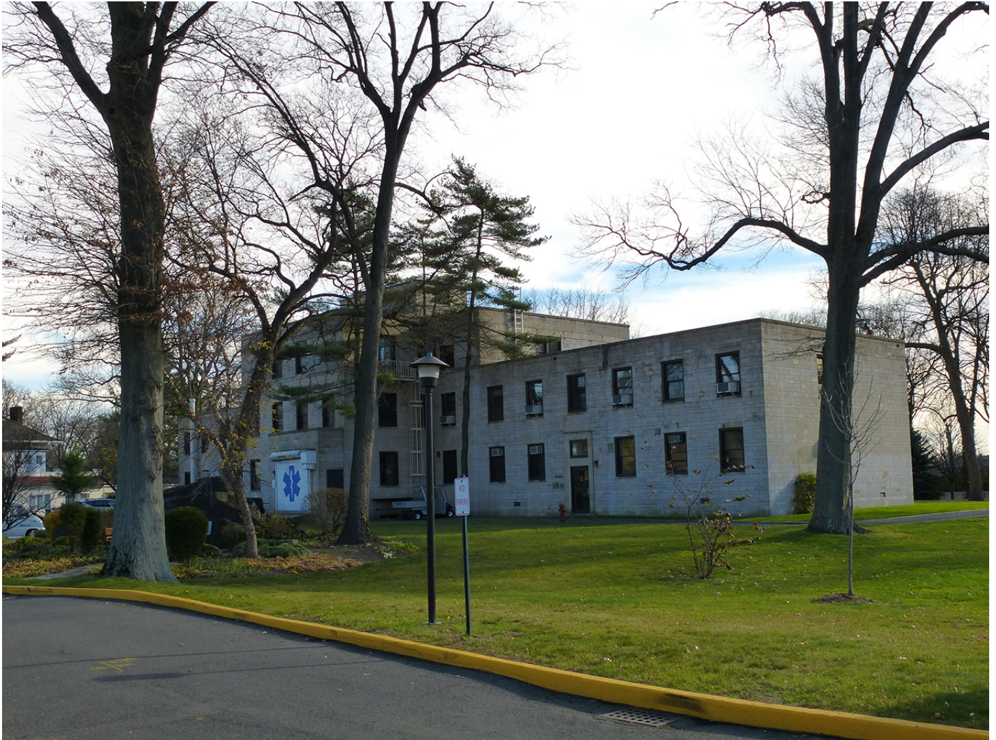
Photo 31. View to the southeast of Patten Health Clinic.
