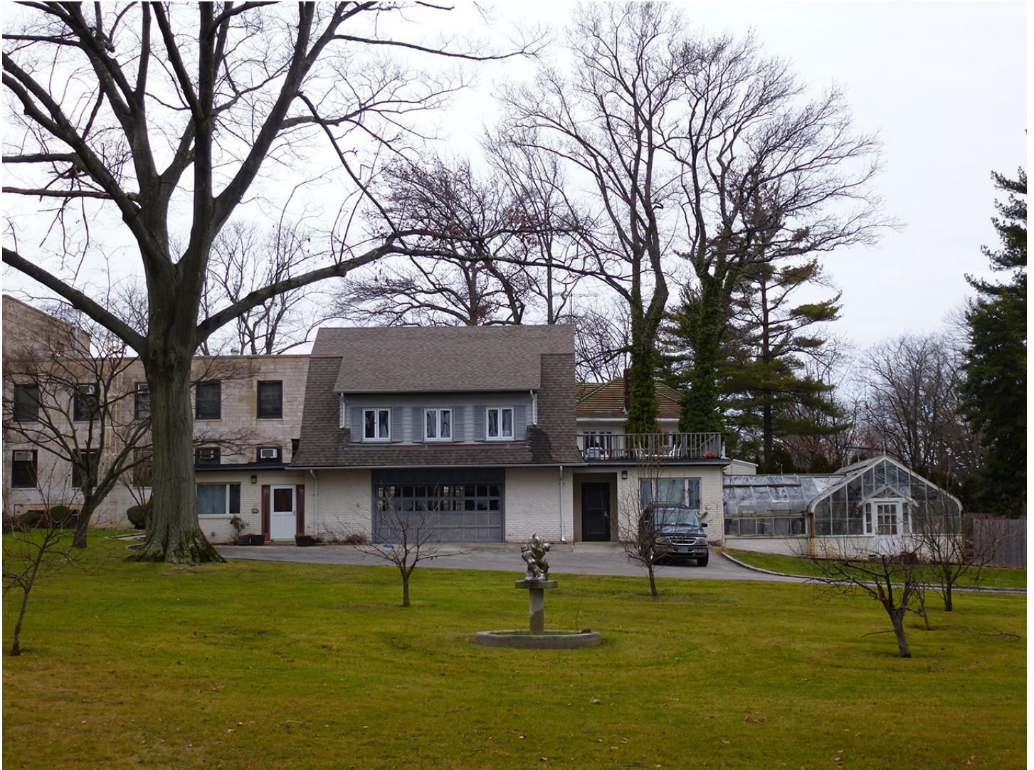
Photo 21. View to the north of Quarters J (Neiley House Garage).
