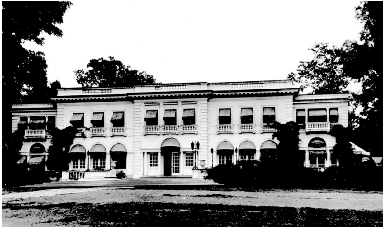
Figure 27. Former west-side loggia, newly enclosed on Wiley Hall, 1942 (Bland Library, USMMA).
