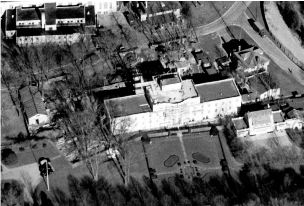
Figure 19. 1943 aerial showing the new Patten Hospital with the Neiley garden in the lower center, the expanded Neiley garage (Quarters J) in the lower right, and the Meighan garage (Quarters K) in the upper right (Bland Library, USMMA).
