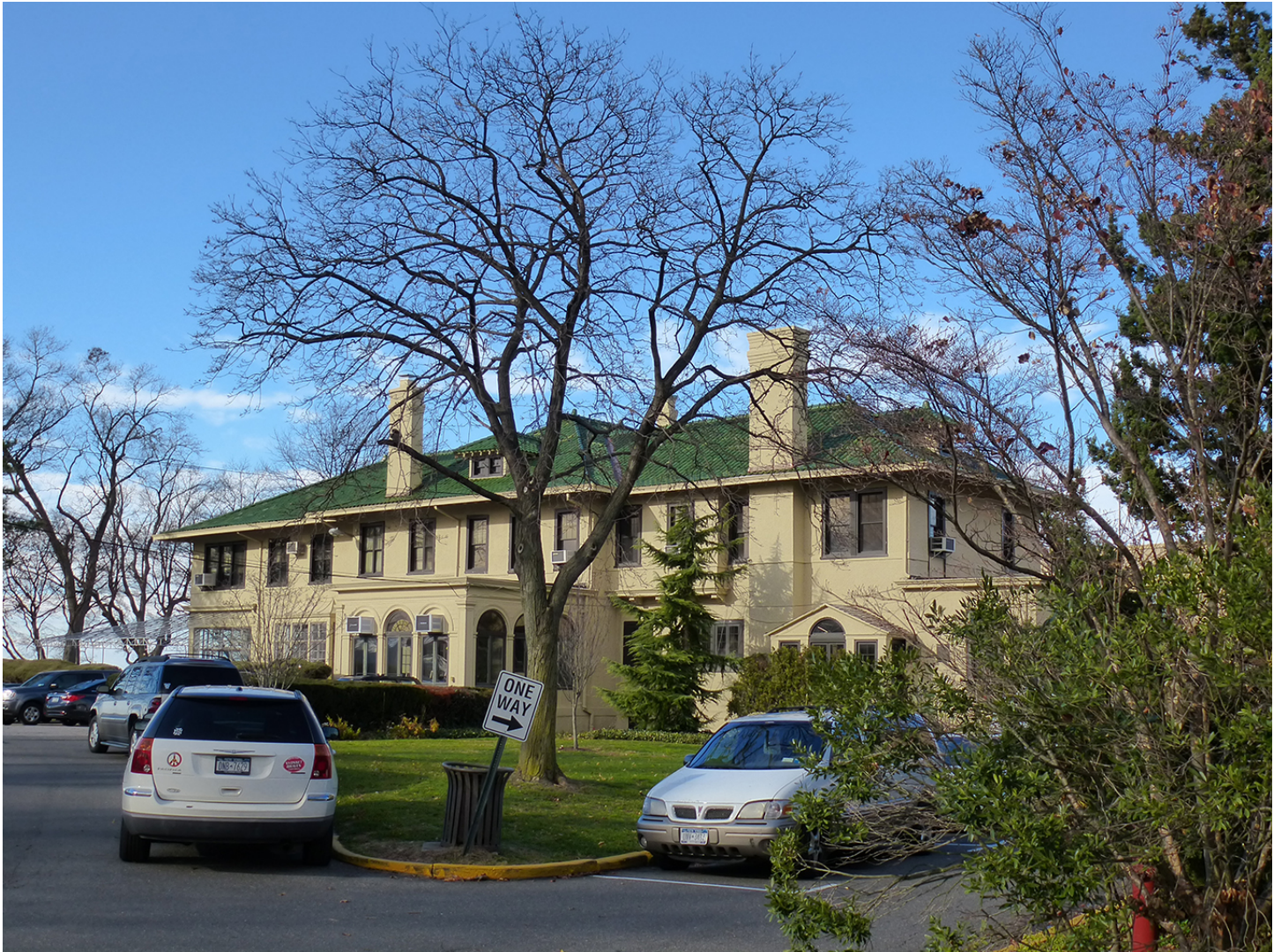
Photo 24. View to the north of Land Hall (Schenck House).
