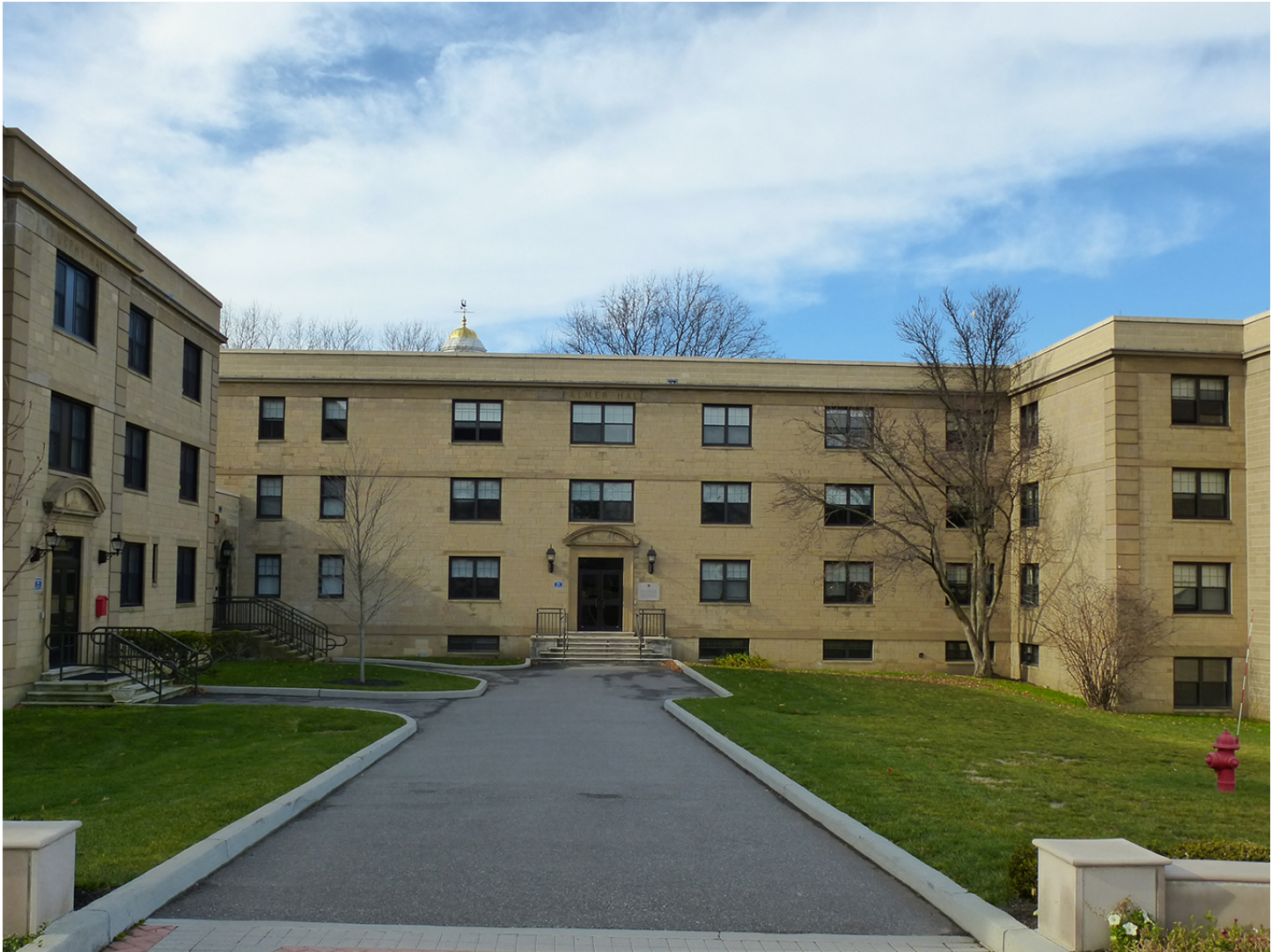
Photo 32. View to the west of Palmer Hall (a typical barracks).
