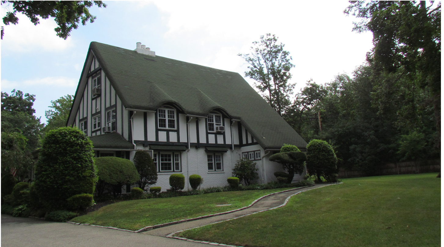
Photo 26. View to the north of Quarters C (Vreeland House).
