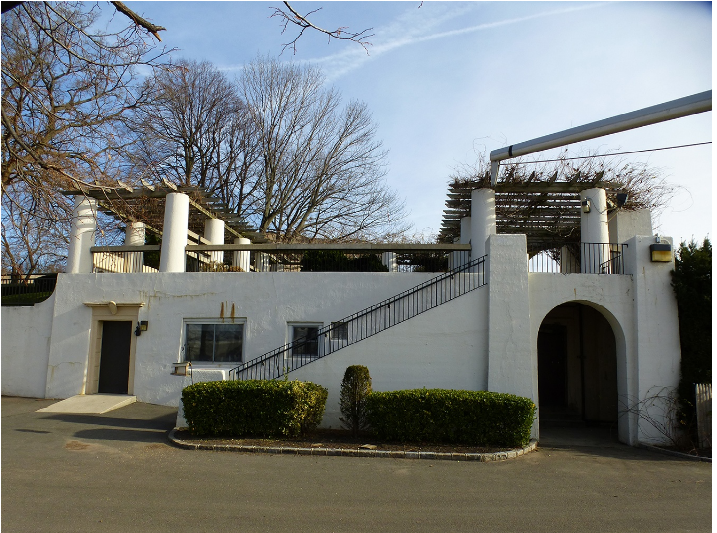
Photo 17. View to the east of the mechanical room for the Eldridge Pool.
