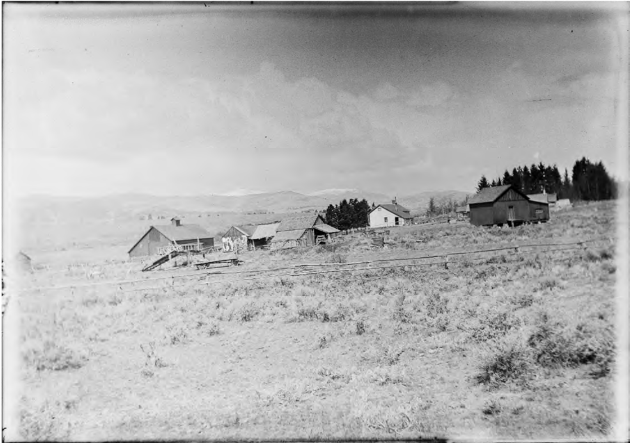
Figure #5 GPC-53 GehringGlassPrint53.tif. Ca. 1914. Ranch Overview. Camera facing northwest.
