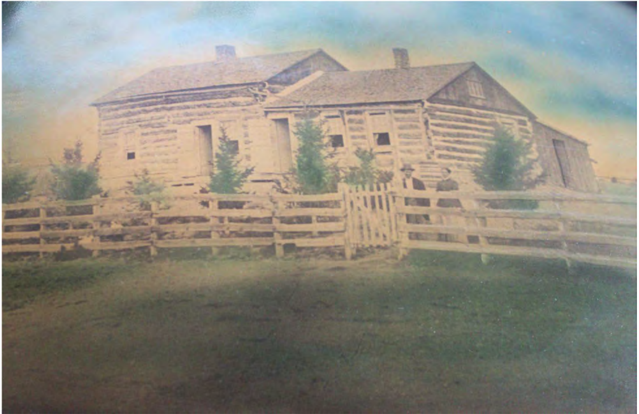
Figure #8 GPC-47 GehringHouse-1870s-2.tif. Ca. 1875-1880. Original log cabins on the Gehring Ranch.
