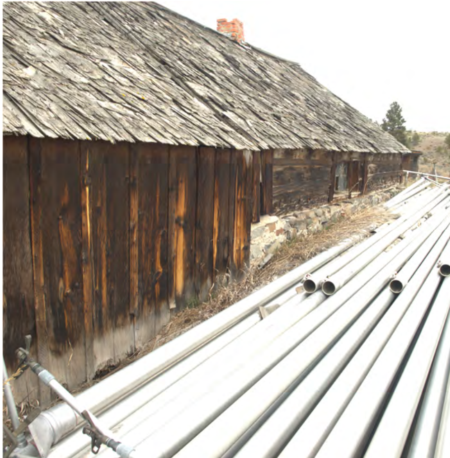
Building #17 Hen House, Contributing, Photo-3 Elevation View. Camera Facing North. Southeast Elevation. Board and Batten Addition Wall (Left) Log On Stone Wall (Right). Shows shingles prior to re-roofing. MT_LewisAndClarkCounty_GehringRanch_0041
