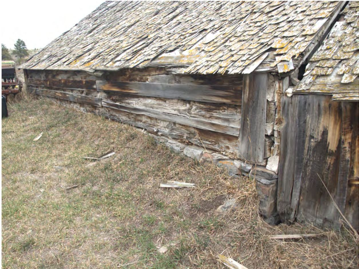
Building #17 Hen House, Contributing, Photo-2 Elevation View. Camera Facing East. Northwest Elevation. Original Log On Stone Wall (Left) Board and Batten Addition Wall (Right). Shows shingles prior to re-roofing. MT_LewisAndClarkCounty_GehringRanch_0040
