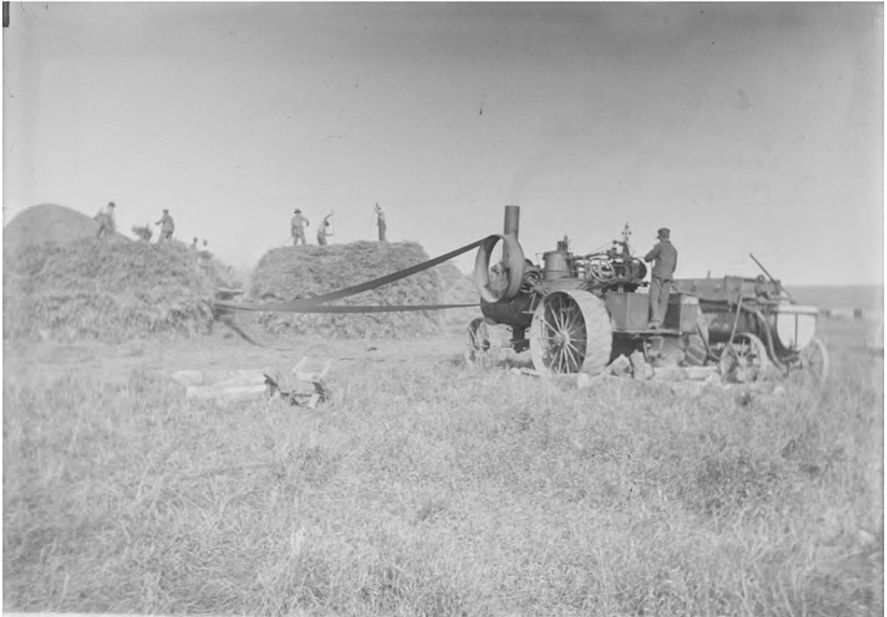
Figure #4 GPC-43 GehringGlassPrint43.tif. Ca. 1910. Steam tractor powering a threshing machine.
