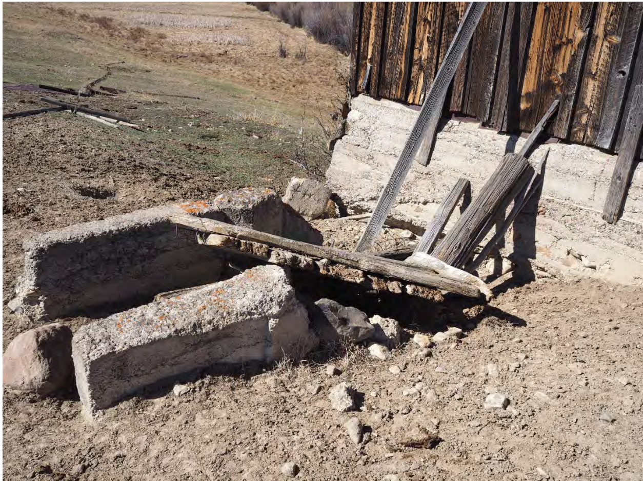
Building #27 Feed Mill, Contributing, Photo-3 Elevation View. Camera Facing North. Concrete Basin (Headgate) to Supply Pipe to Waterwheel (Foreground). Southwest Elevation of Mill (Right) MT_LewisAndClarkCounty_GehringRanch_0070
