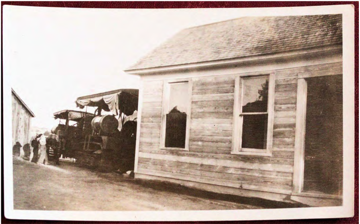
Figure #10 GPC-91 GehringGlassPrint-91.tif. 1929. Moving Bunkhouse #2 from Hardie homestead.
