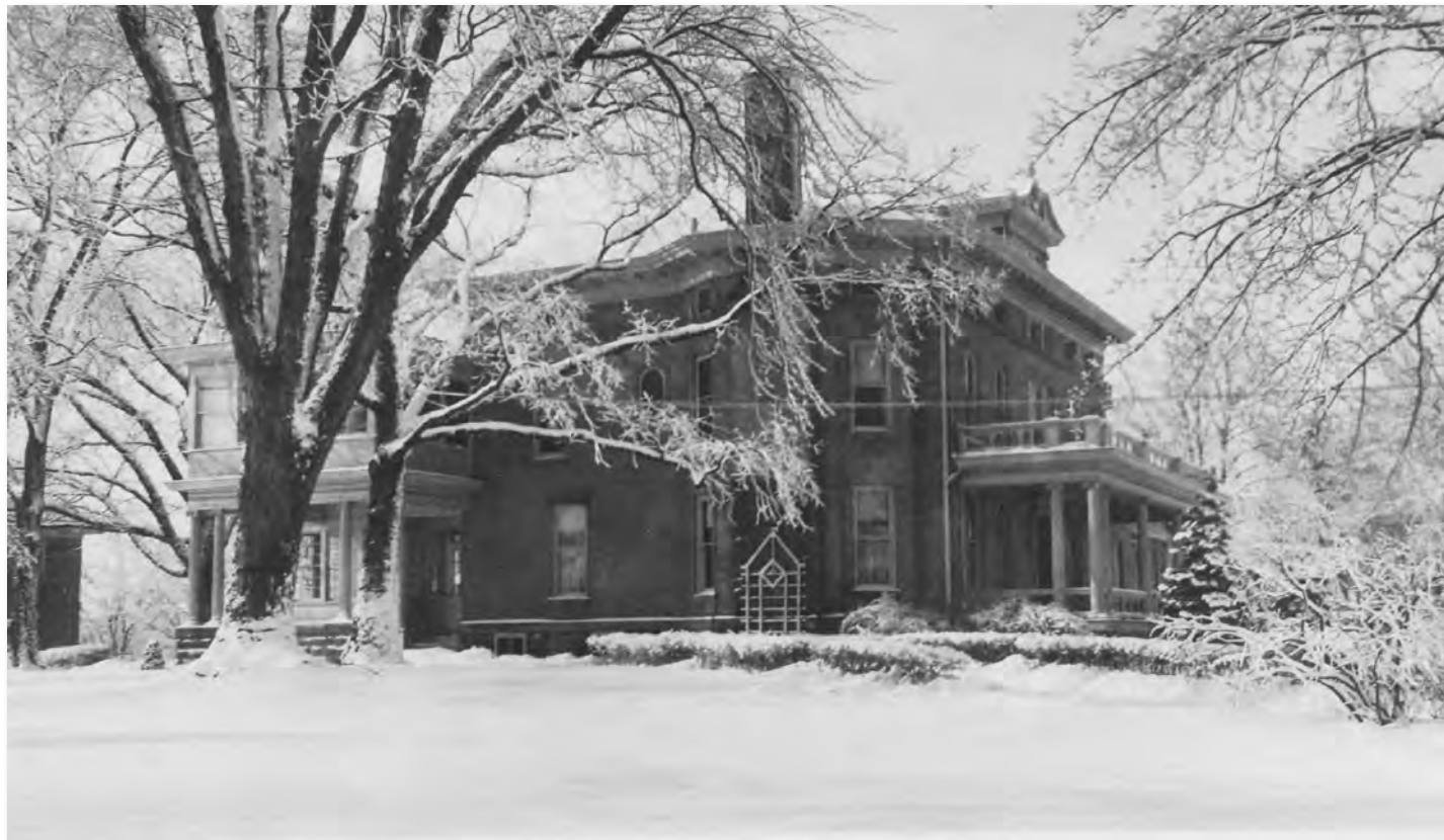
Figure 14. View north of the Laura Musser McColm House, c.1925. Note the second floor sleeping porch has been built above the porte-cochere. Source: Muscatine Art Center, Muscatine, Iowa
