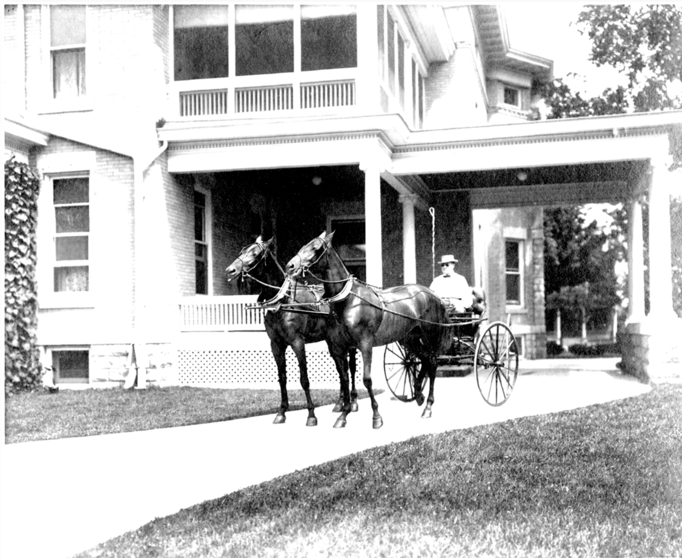
Figure 18. View of original porte-cochere and drive before sleeping porch was added above, early 1910s. Source: Muscatine Art Center, Muscatine, Iowa
