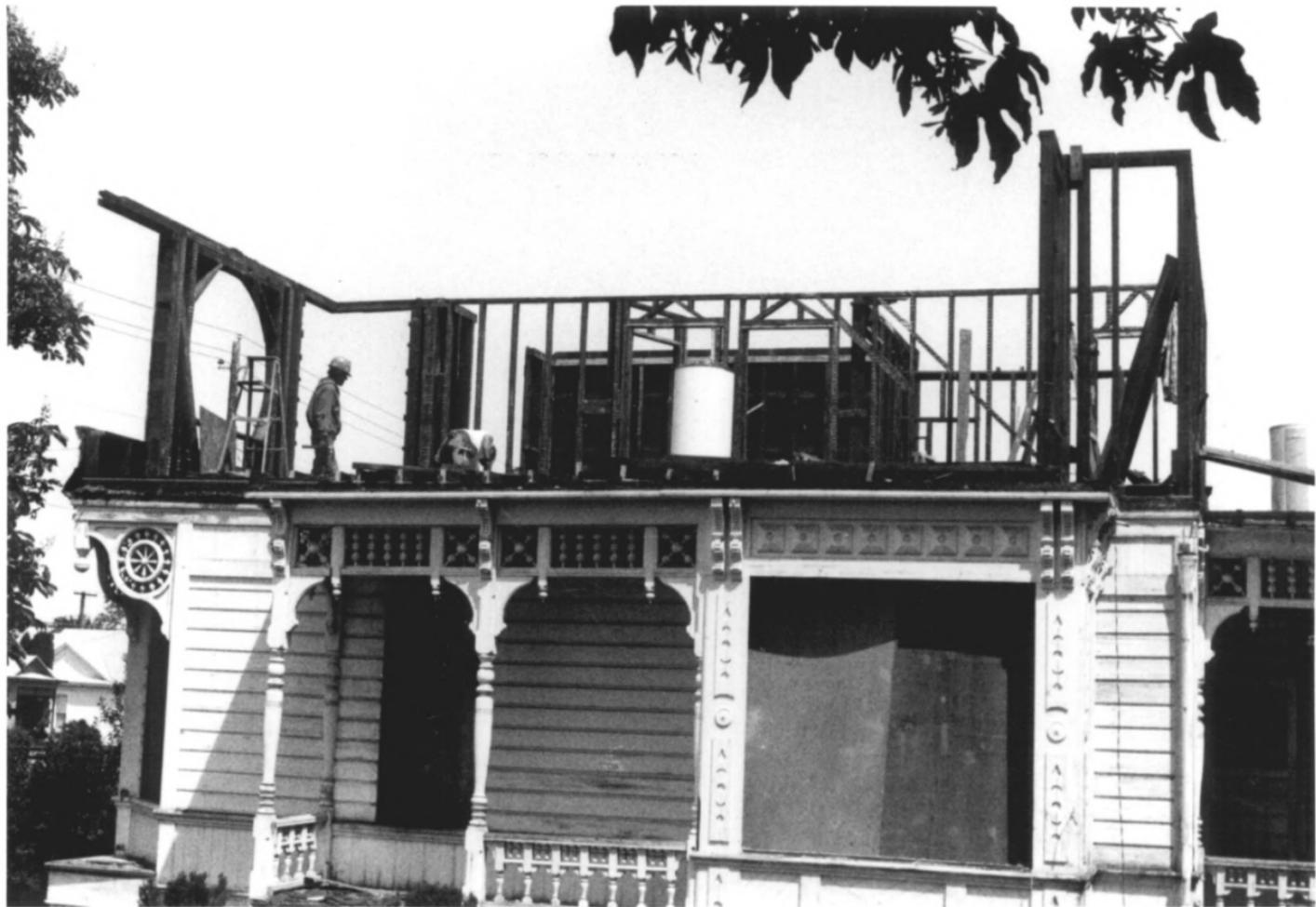
West elevation showing removal of second story. Balloon construction was cut off at floor and later reconstructed in the platform style with original 19th century building materials.
