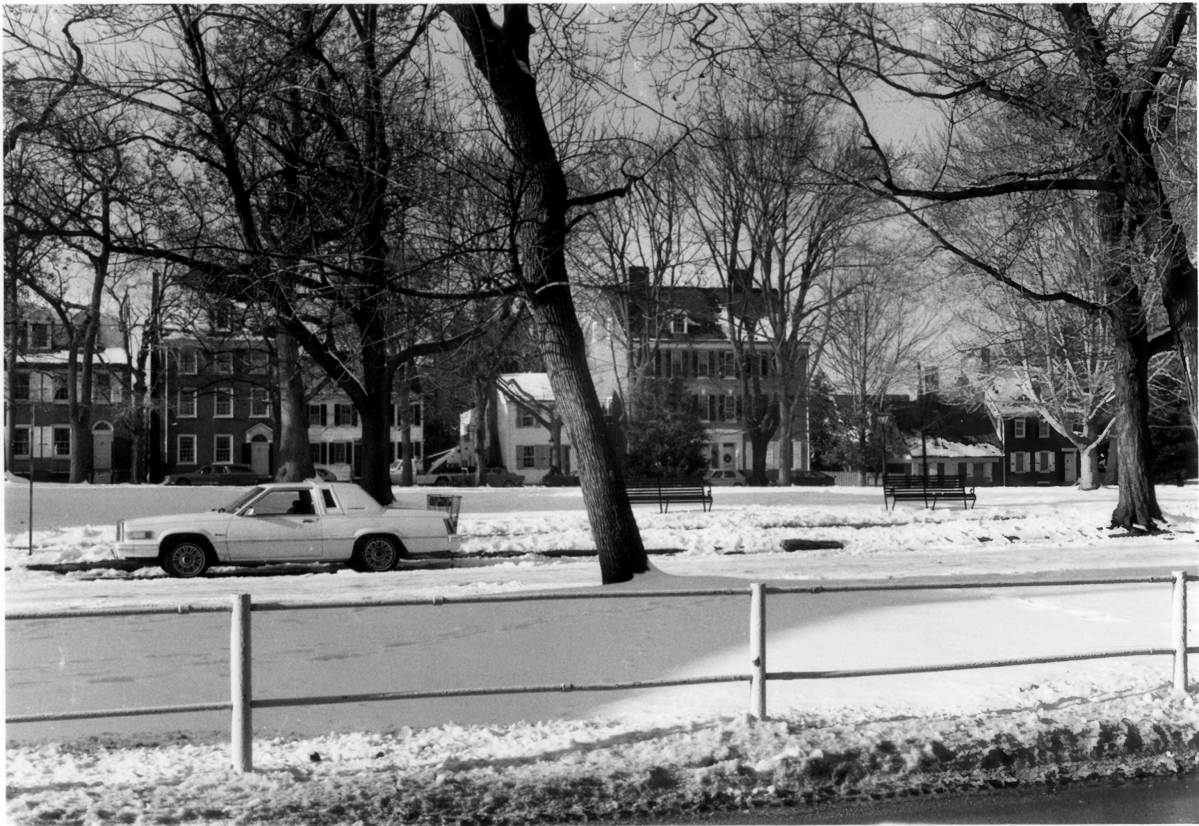
N-349 VIEW ACROSS THE GREEN TOWARD 3RD ST.
