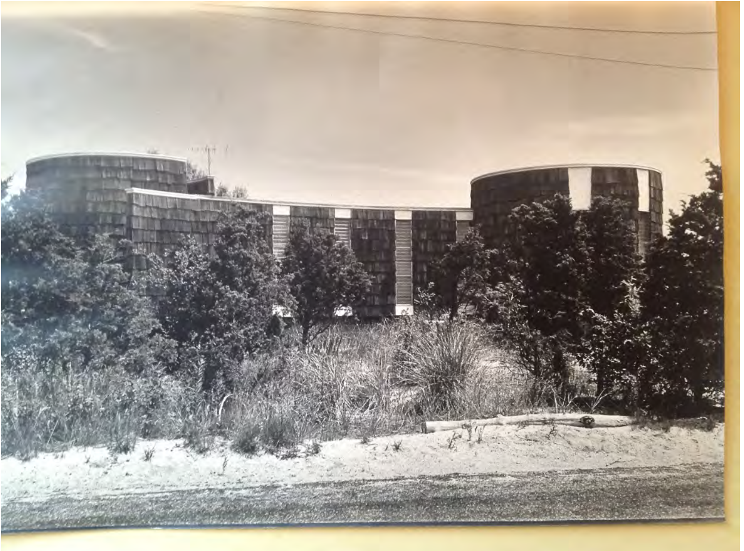
Supplemental Photo 17. Edwin Heitman House, Barnegat Light, New Jersey (1961). Photograph from the Tofani Collection, Athenaeum of Philadelphia.
