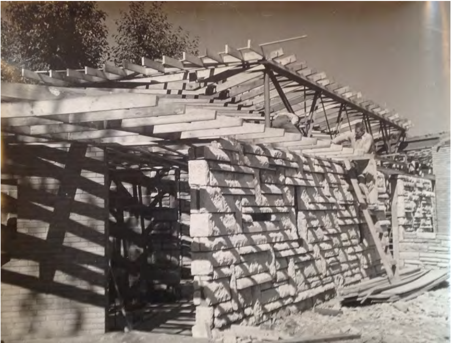
Supplemental Photo 23. Dr. and Mrs. Robert Green House, Philadelphia. Under construction.
