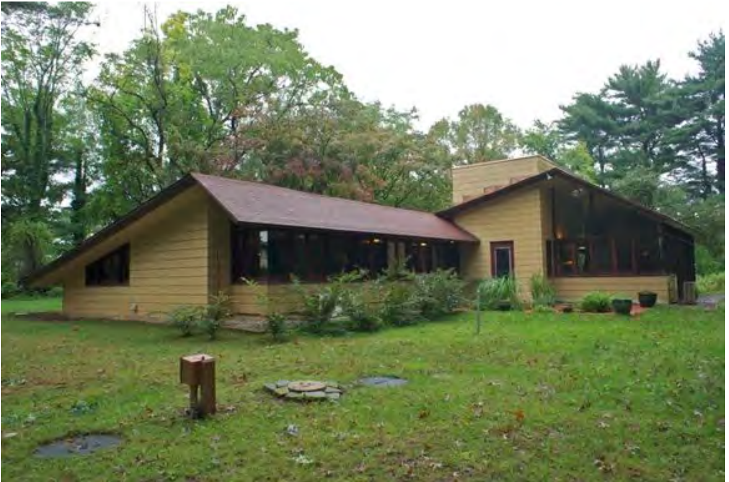
Supplemental Photo 7. Sweeton House, Cherry Hill, New Jersey. Designed by Frank Lloyd Wright (from PrairieMod website: www.prairiemod.com ).
