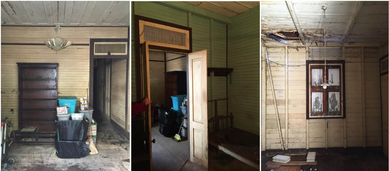
Figures 8 to 10: Living room, master bedroom and bedroom/dressing room of Casa Vigil (note the woodwork, drop-ceiling finishing, partitions and transoms), 2017. (YMCR)
