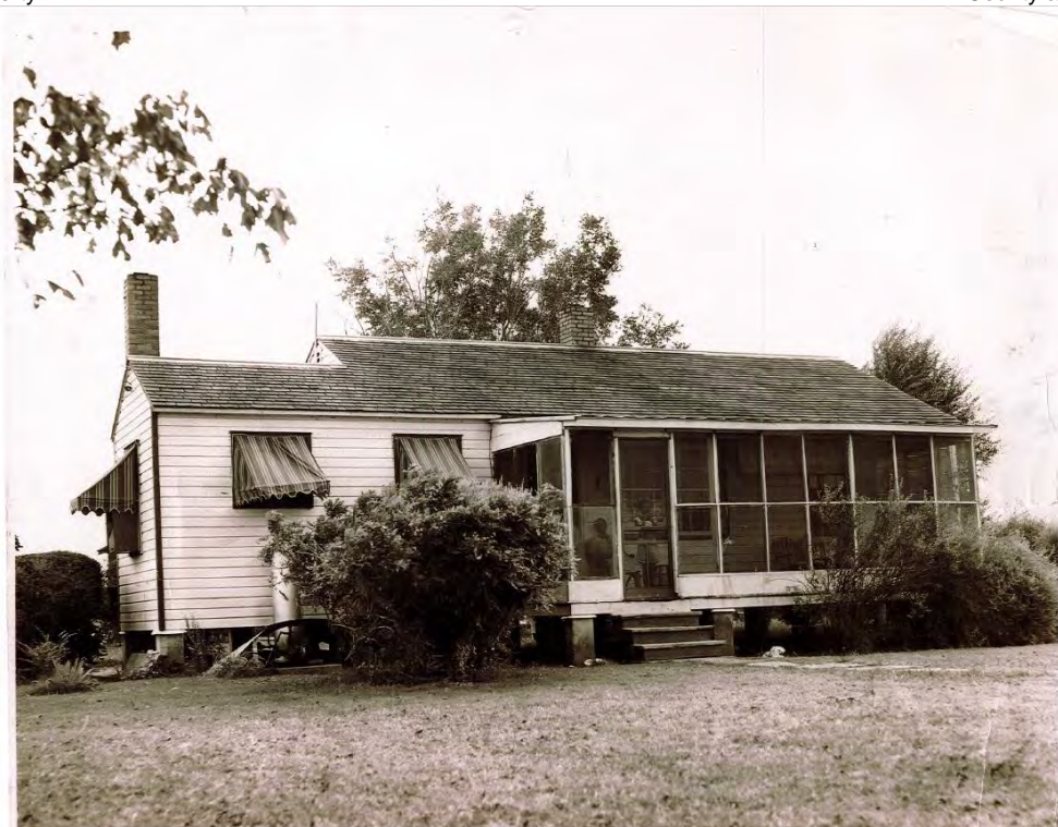
Lakeview Project House ca. 1970 Files of the AR Historic Preservation Program
