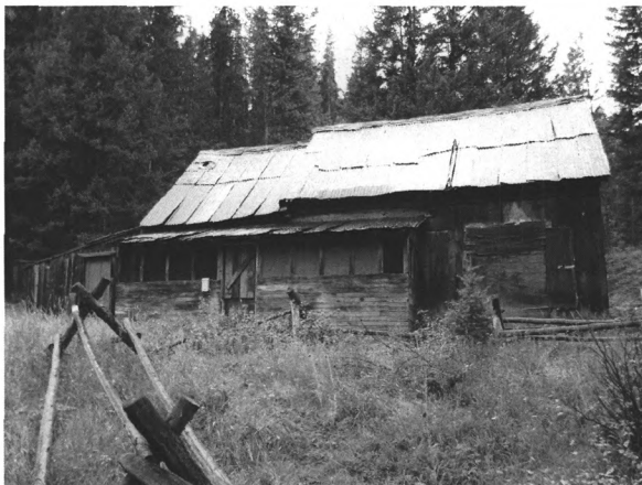
Photo 0039. Feature 41, Kreiger House, facing west.
