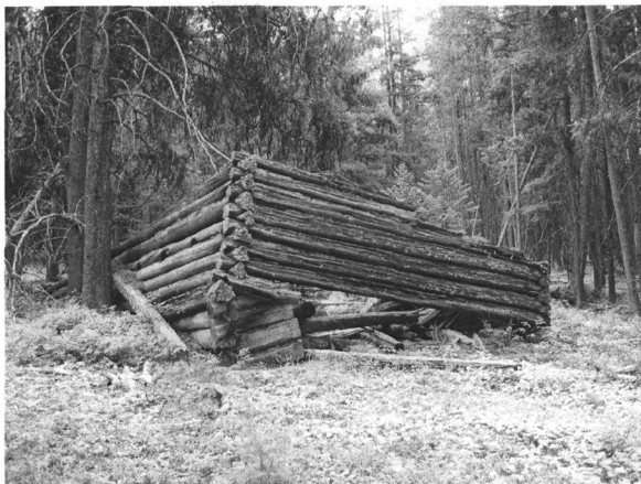
Photo 0054. Feature 74, log building, facing east.
