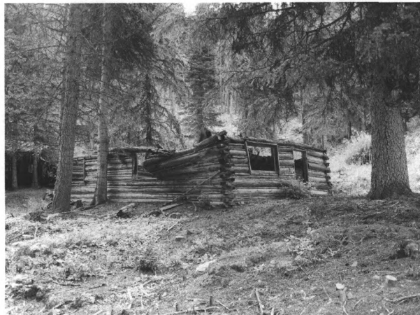
Photo 0059. Feature 100, log building, facing east.
