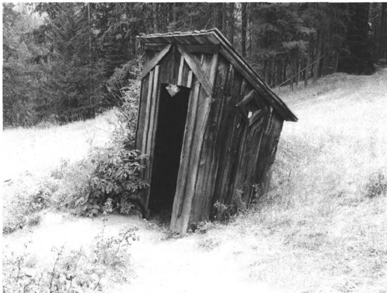
Photo 0019. Feature 18a, outhouse, facing southeast.
