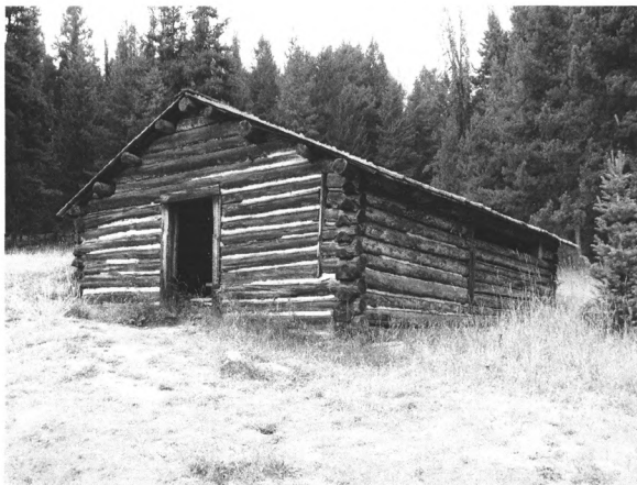
Photo 0013. Feature 13, log building, facing southwest.
