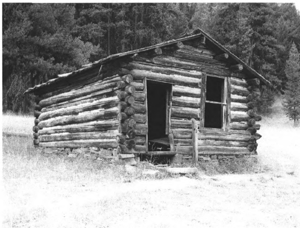
Photo 0017. Feature 17, Post Office, facing southwest.
