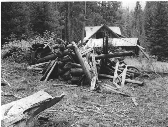
Photo 0066. Feature 113, log building, facing east.
