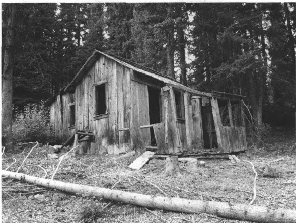
Photo 0058. Feature 99, frame building, facing southeast.
