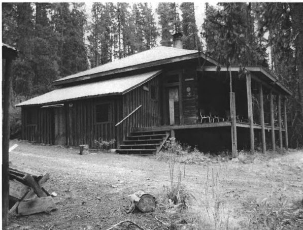
Photo 0063. Feature 105, Fitzgerald House, facing south.
