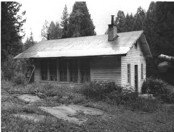
Photo 0037. Feature 40, Schoolhouse, facing northwest.
