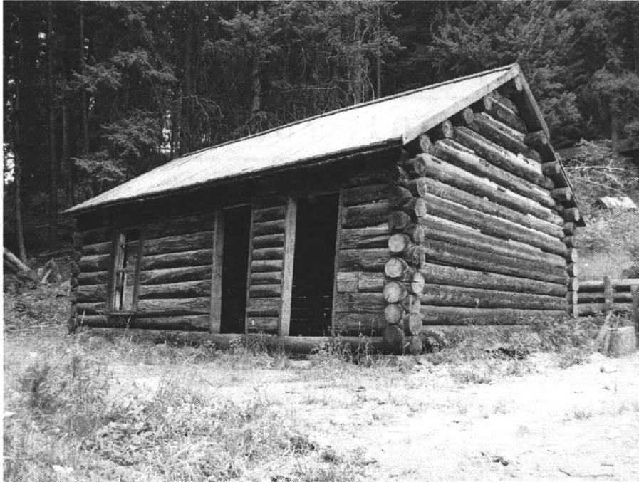
Photo 0029. Feature 33, log building, facing southwest.
