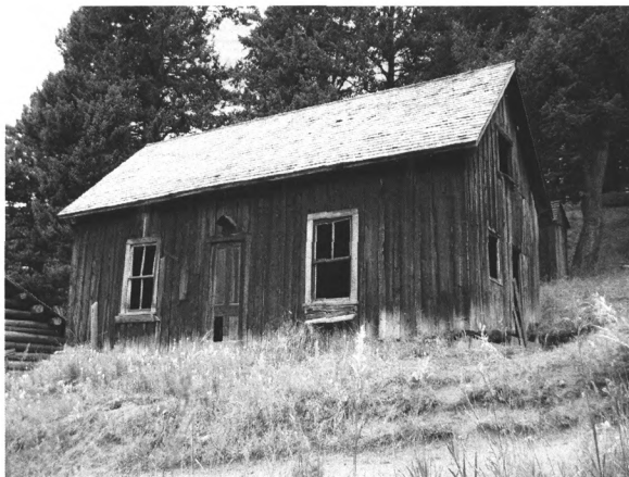
Photo 0041. Feature 45, Hannifen House, facing west.
