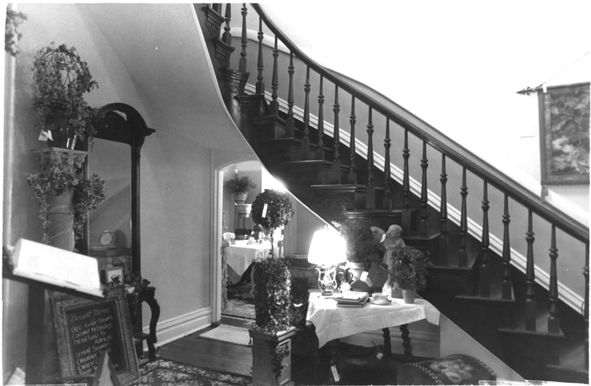
NORTHINGTON-DEATH HOUSE MONTGOMERY COUNTY, TN
