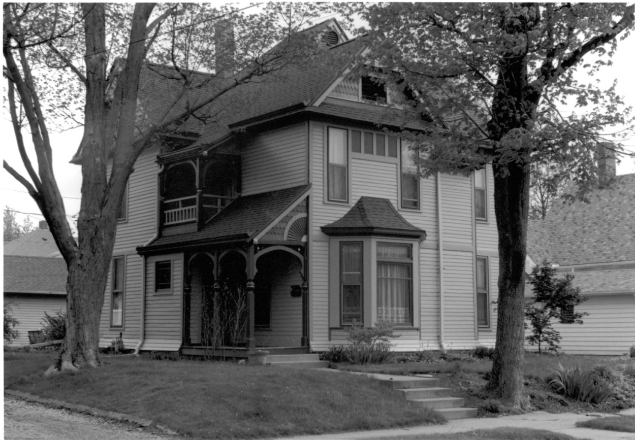
453 S. CLAY ST.; CHRISTIAN RIDGE HIST. DIST., FRANKFORT, CLINTON CO.; IN, PHOTO NO. 30
