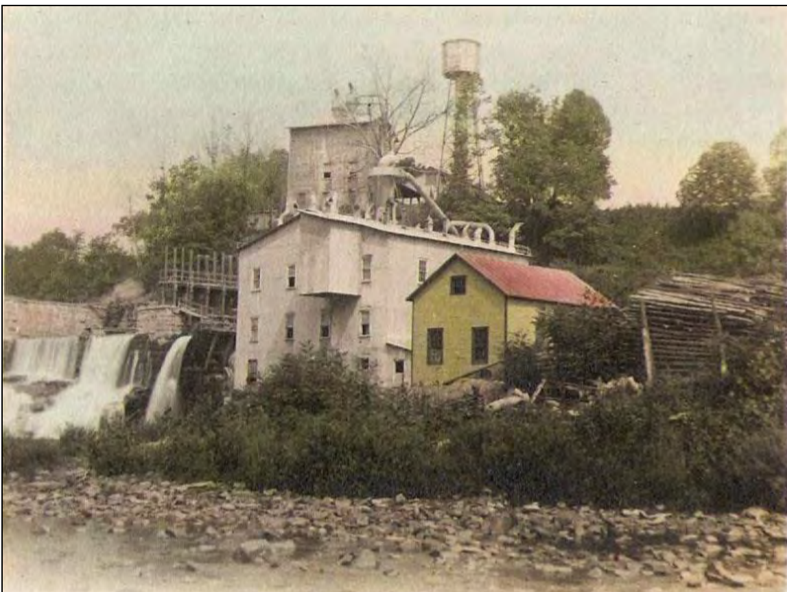
Fig.5: View of Eastern Dynamite Co., formerly Hudson River Pulp & Paper Mfg. Co., ca; 1906.
