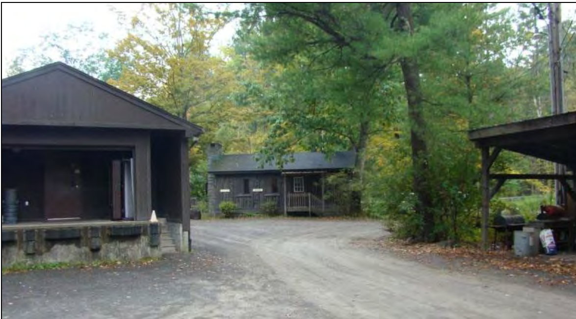
Fig. 9: View of SUNY New Paltz Ashokan Field Campus Bunkhouses prior to demolition in 2012. From Phase 1 Cultural Resource Survey, Ashokan Field Campus Demolition Project Town of Olive, Ulster County, New York, November 30, 2012.
