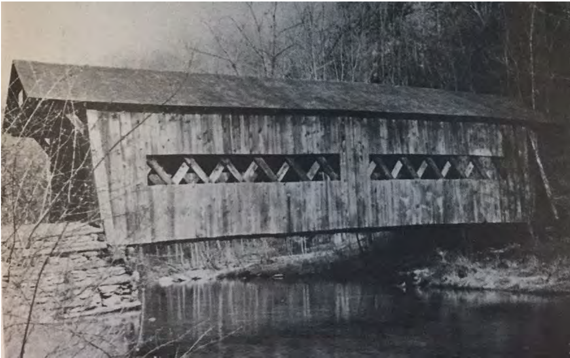
Fig.6: View of Turnwood Covered Bridge after relocation to Ashokan in ca. 1940. From Vera Van Steenberg Sickler, The Town of Olive Through the Years, Part One (1976).
