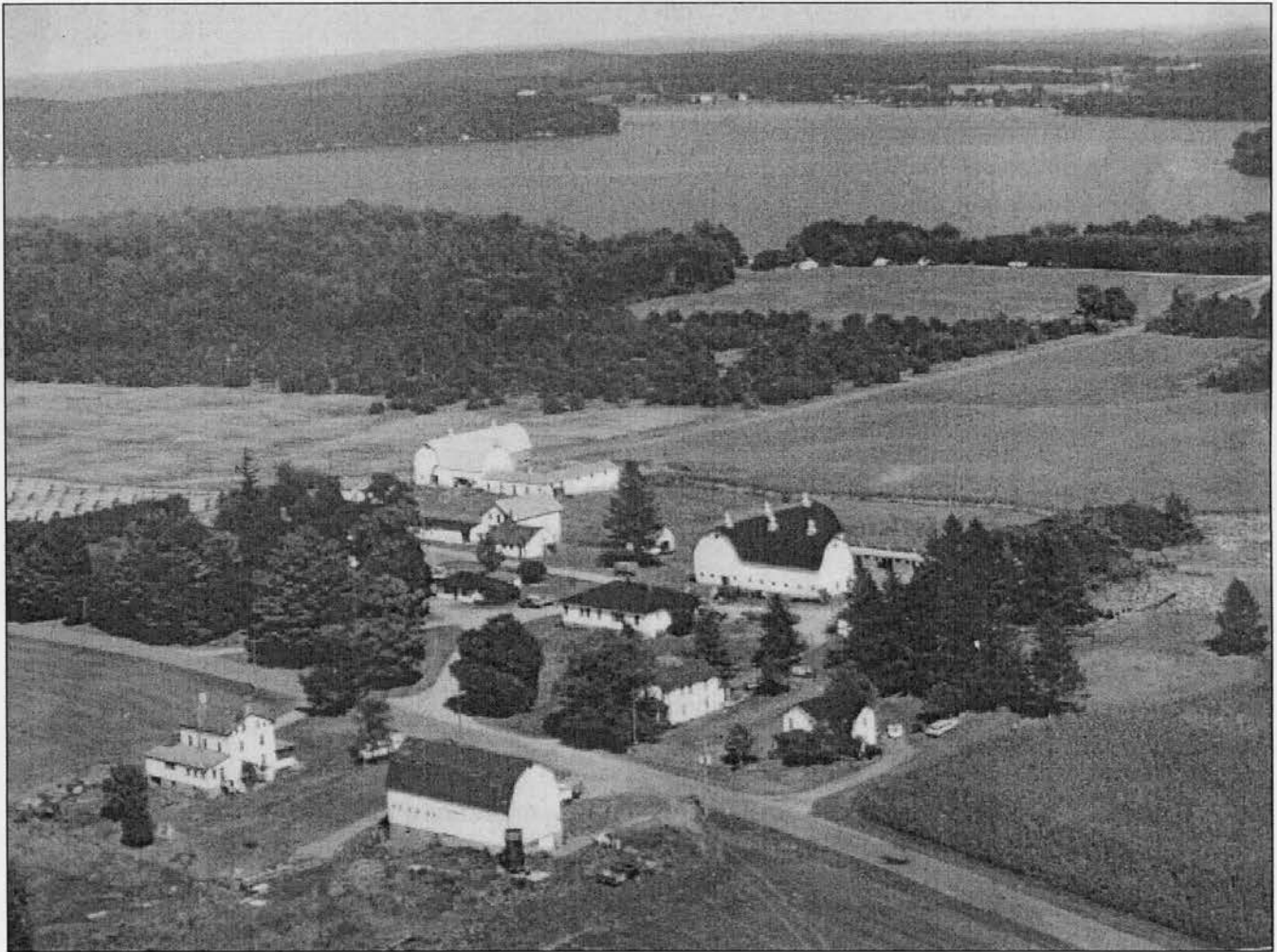
Aerial view of historic house and barn complex; looking northeastward toward Sodus Bay
