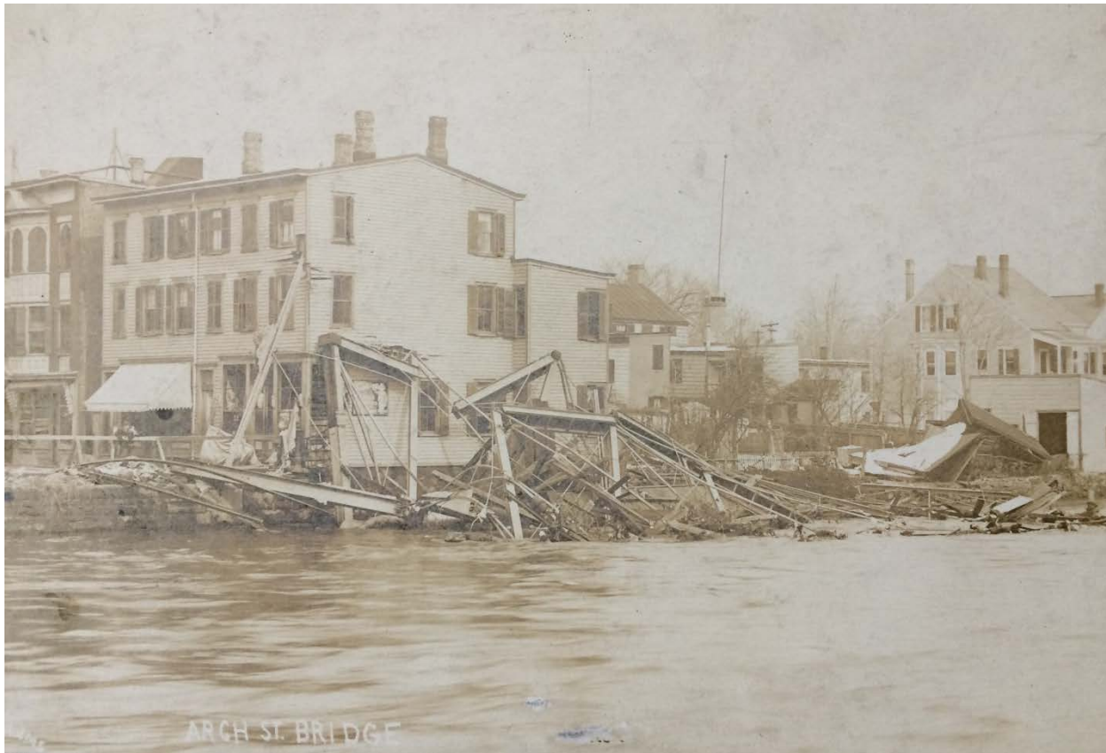
Figure 2. A view of the collapsed Arch Street Bridge following the Flood of 1902 facing south.
