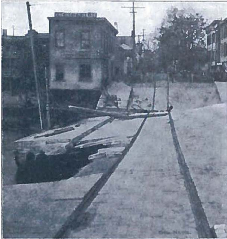
Figure 4. View northwest of the damaged deck of the Arch Street Bridge after the Flood of 1903.
