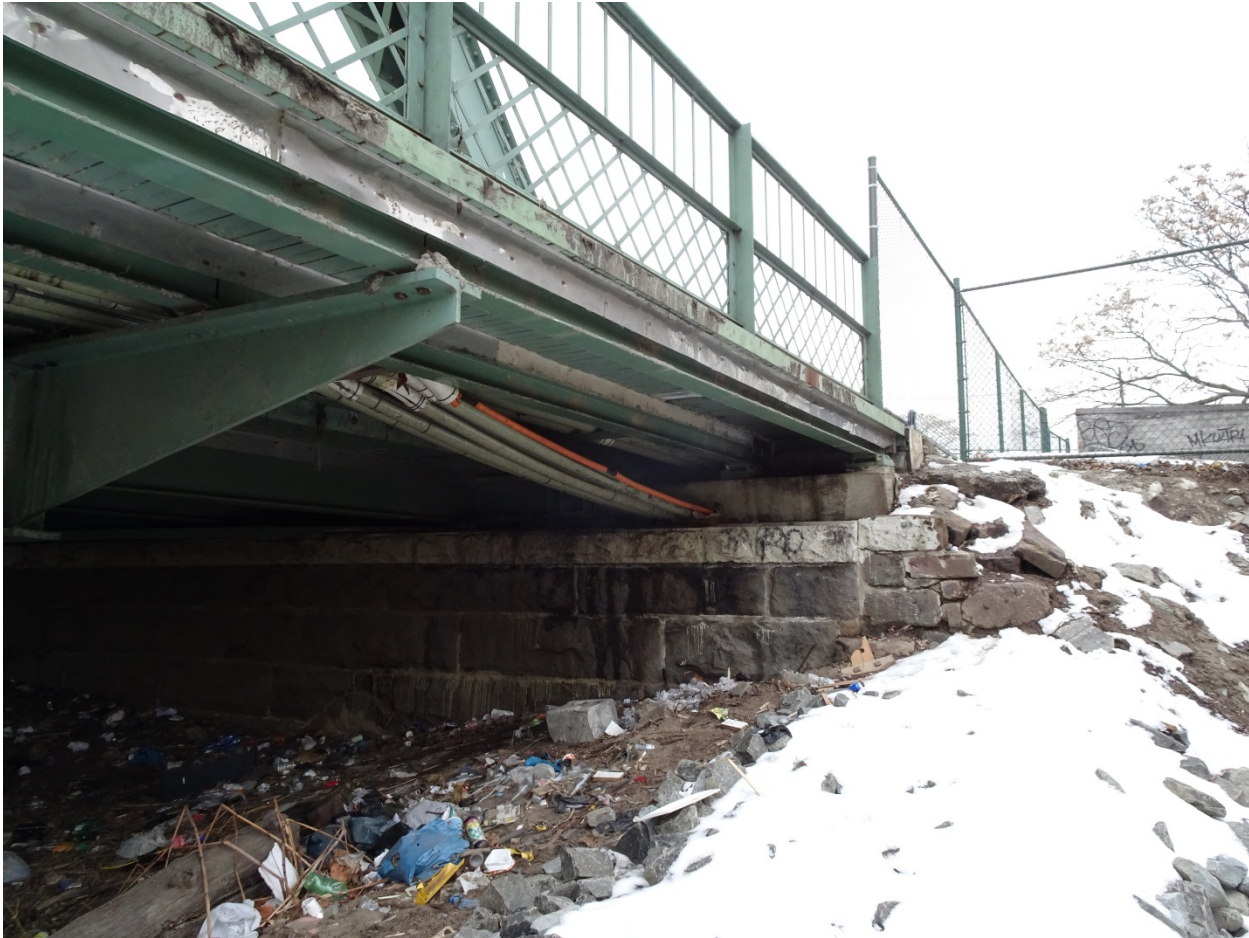
Photograph 4. North abutment, view northwest.
