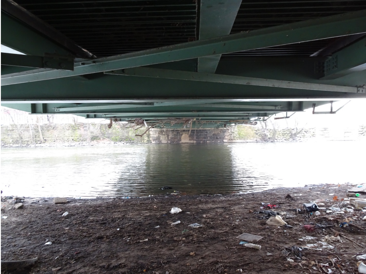
Photograph 5. South abutment from across the Passaic River, view southeast.
