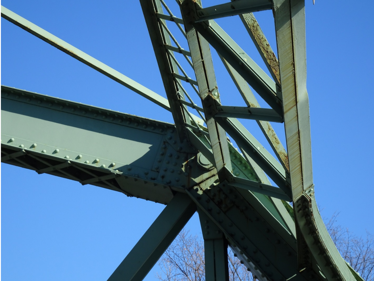
Photograph 9. Detail view of pinned connection, view southwest.
