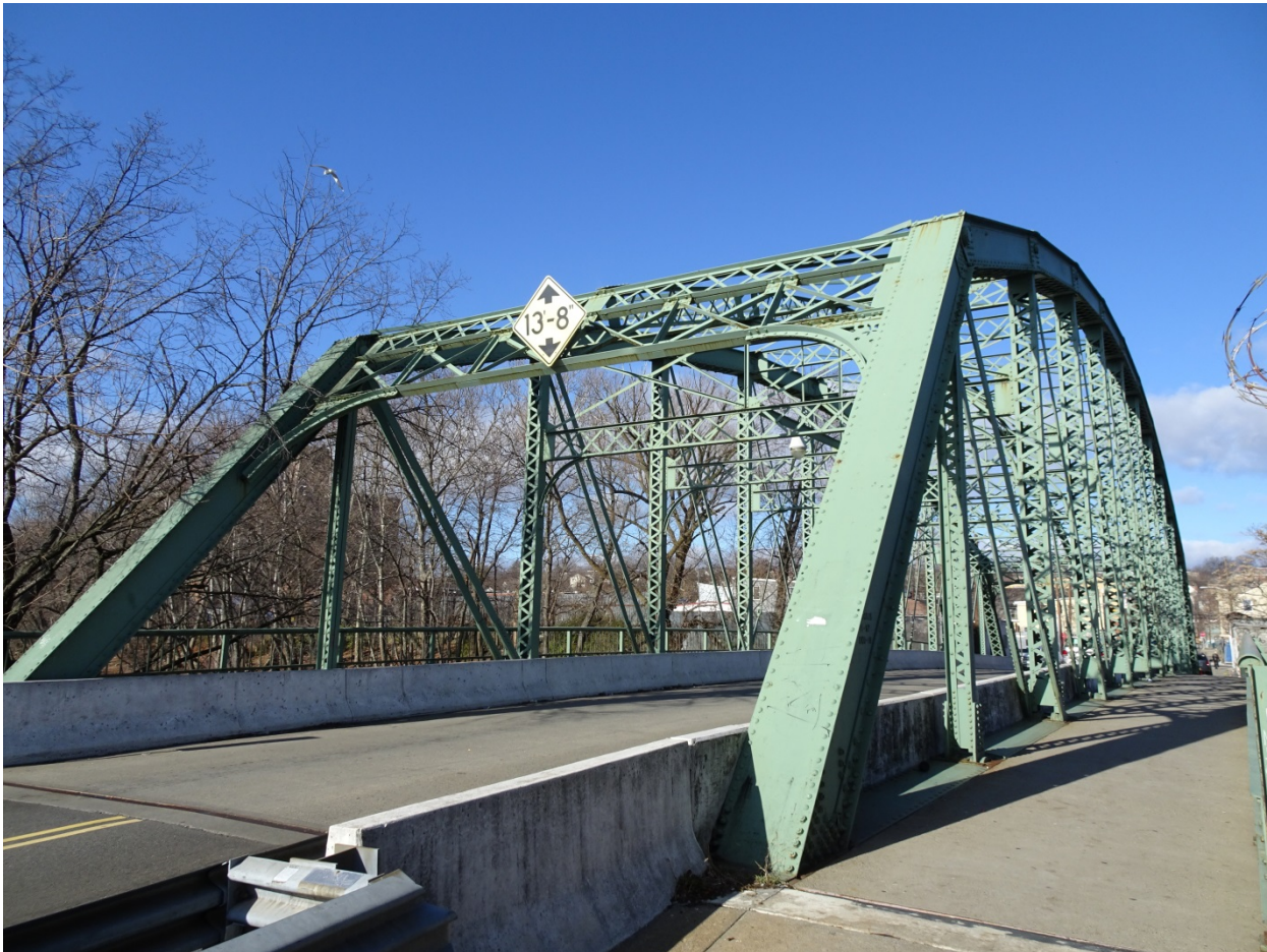
Photograph 1. Bridge approach from the south abutment, view northwest.
