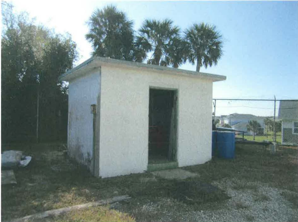
Photo # 8. Storage Building, camera facing south.
