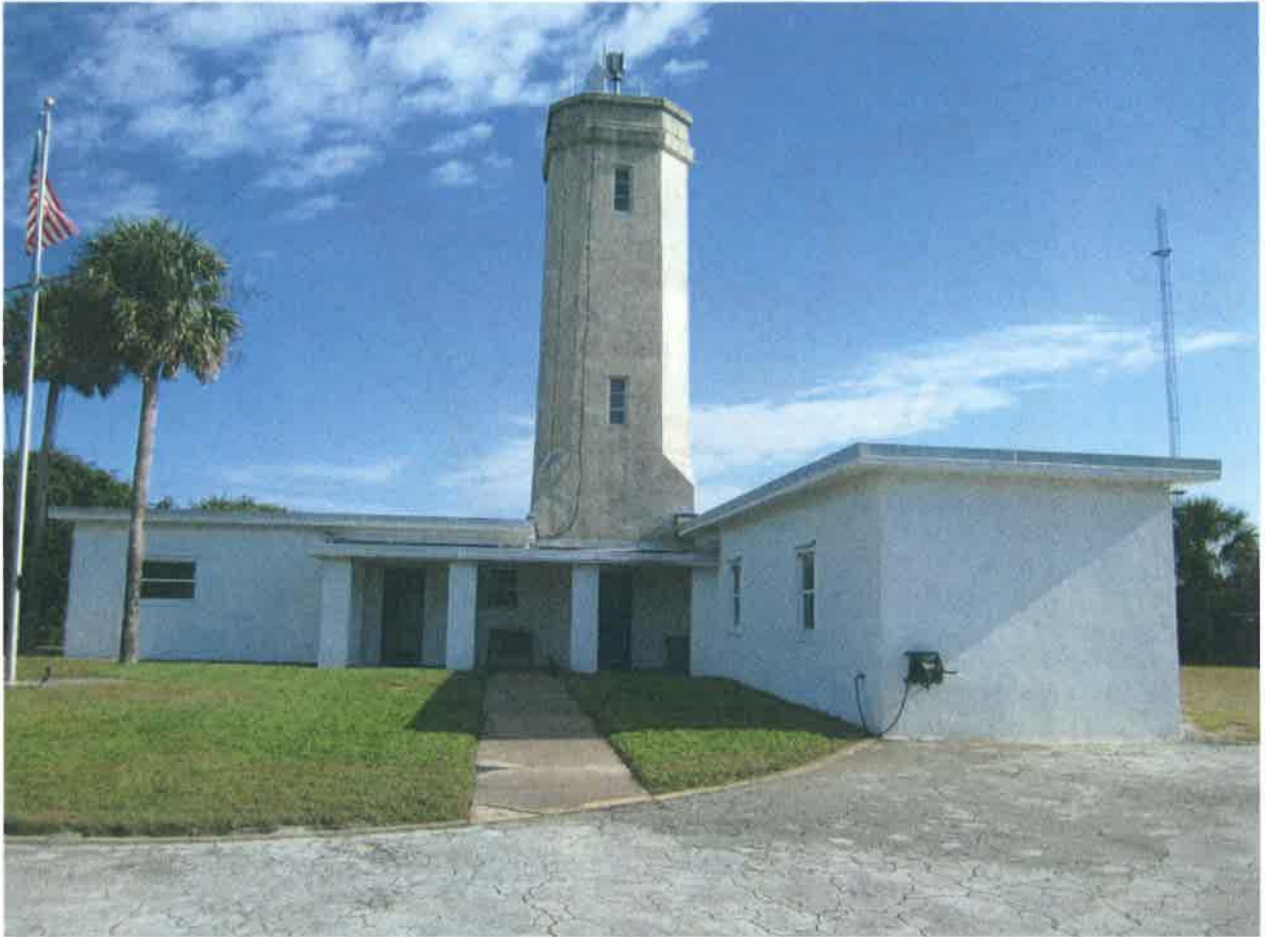
View of the St. Johns Light, camera facing northeast
