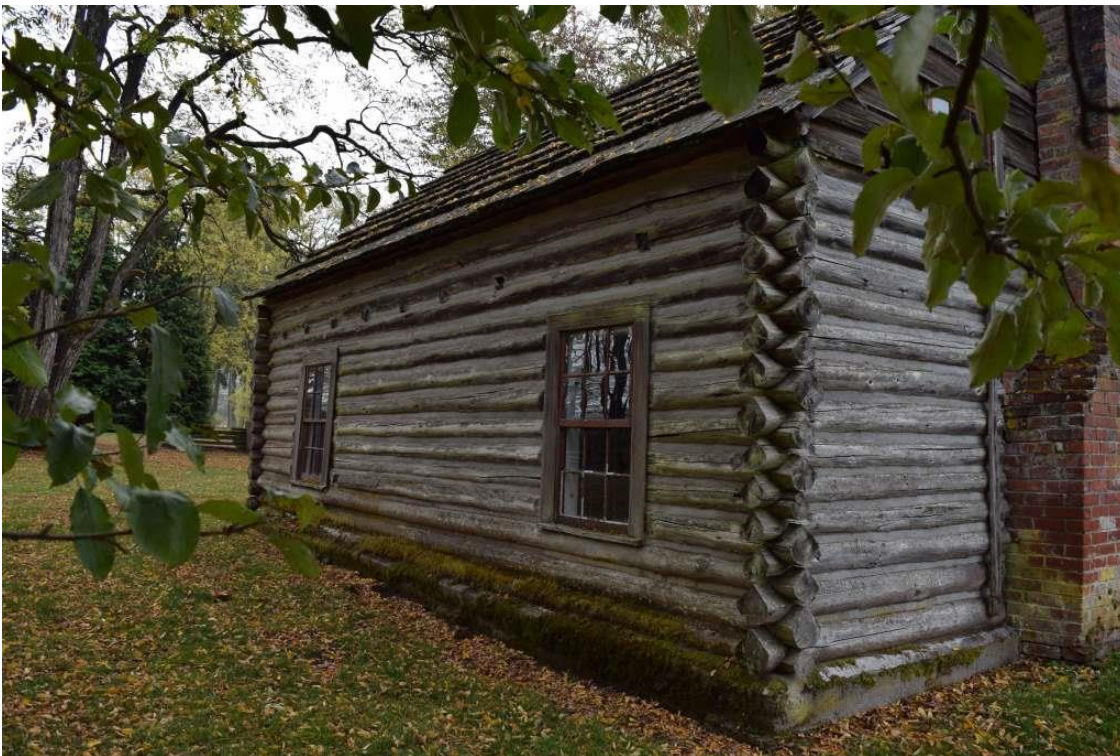
3 of 15. Looking southwest at northeast corner.
