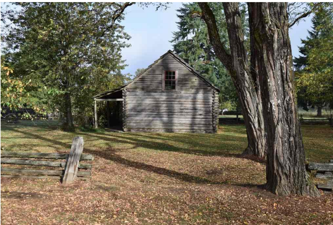
5 of 15. Looking north at south elevation from the southern property boundary.
