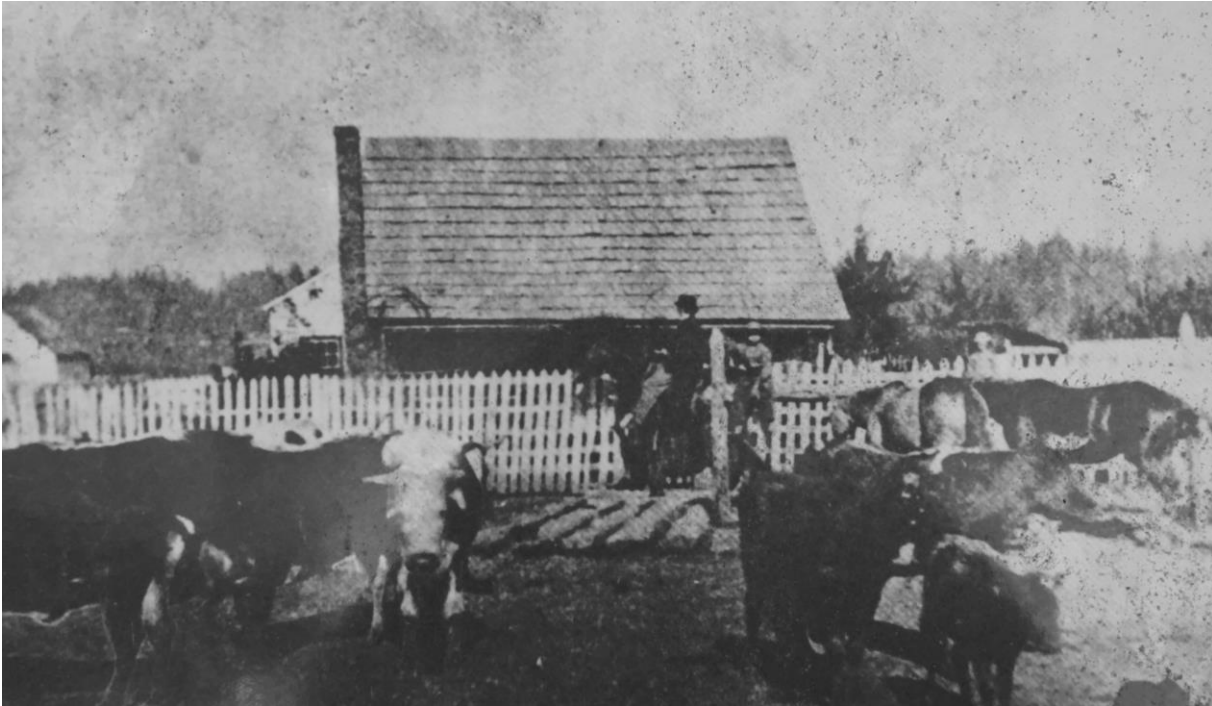
Image of original (1850) John R. Jackson House before addition, ca 1863, view looking east.
