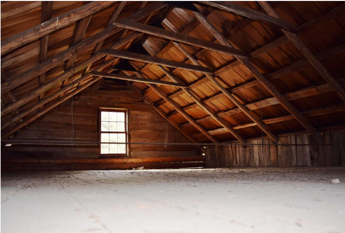
12 of 15. Attic interior looking south.
