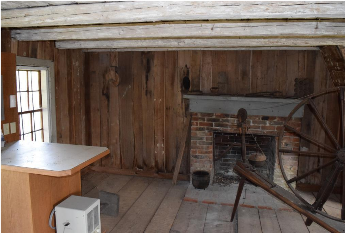
10 of 15. Interior looking north at fireplace, hearth and mantle.
