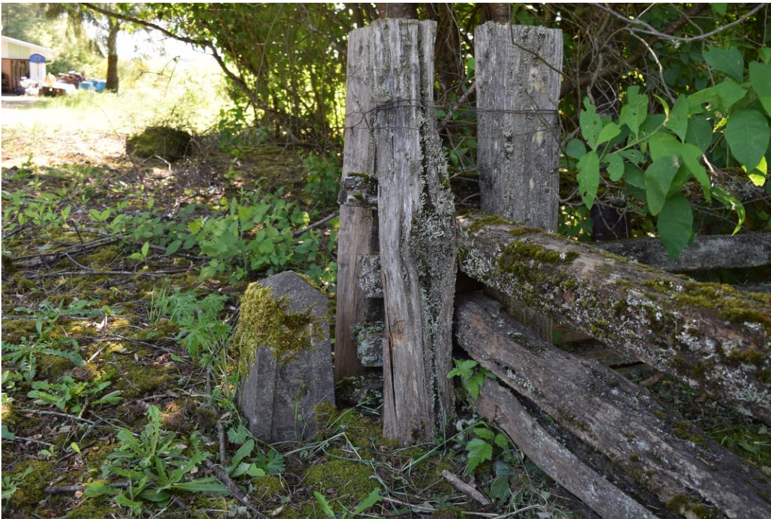
15 of 15. Northeast corner property marker, looking east.
