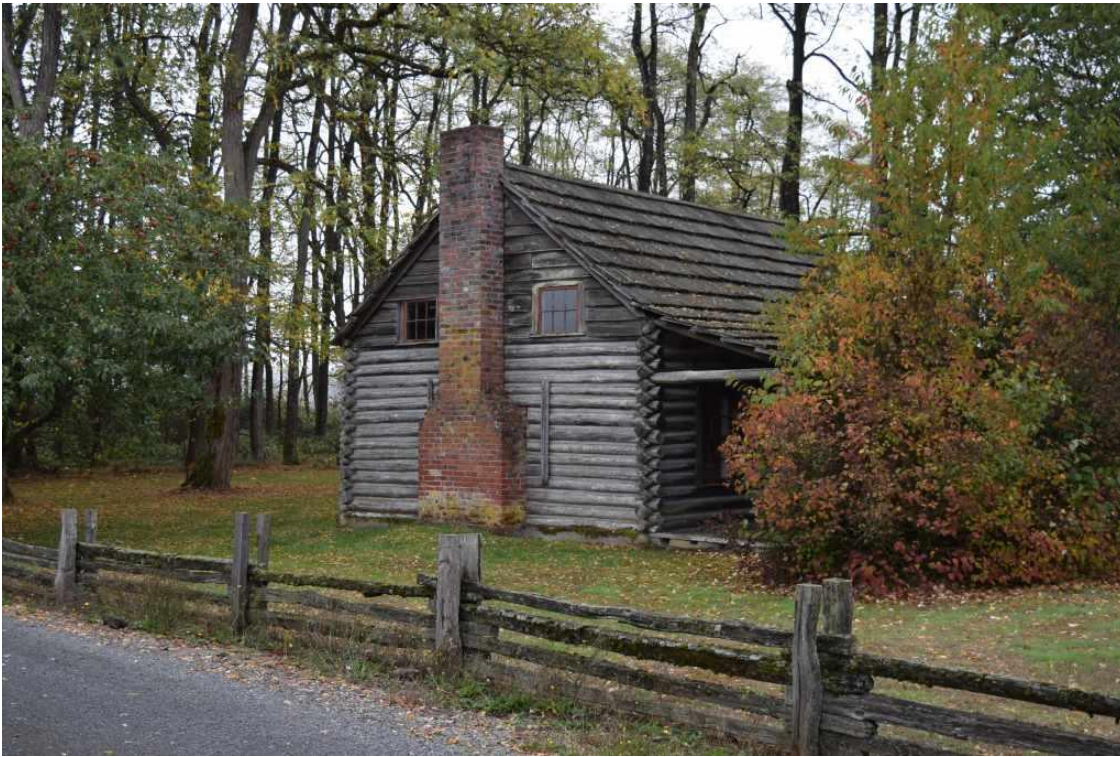
2 of 15. Looking southeast at northwest corner, CCC rail fence in foreground.
