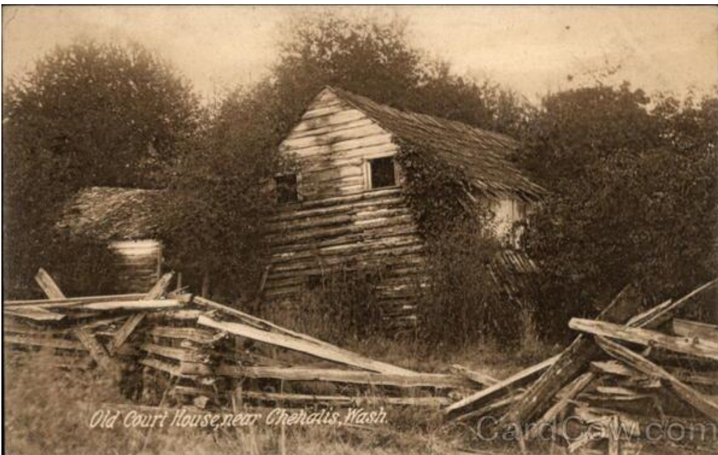
Image of original (1850) John R. Jackson House, ca 1910, showing further deterioration of cabin.
