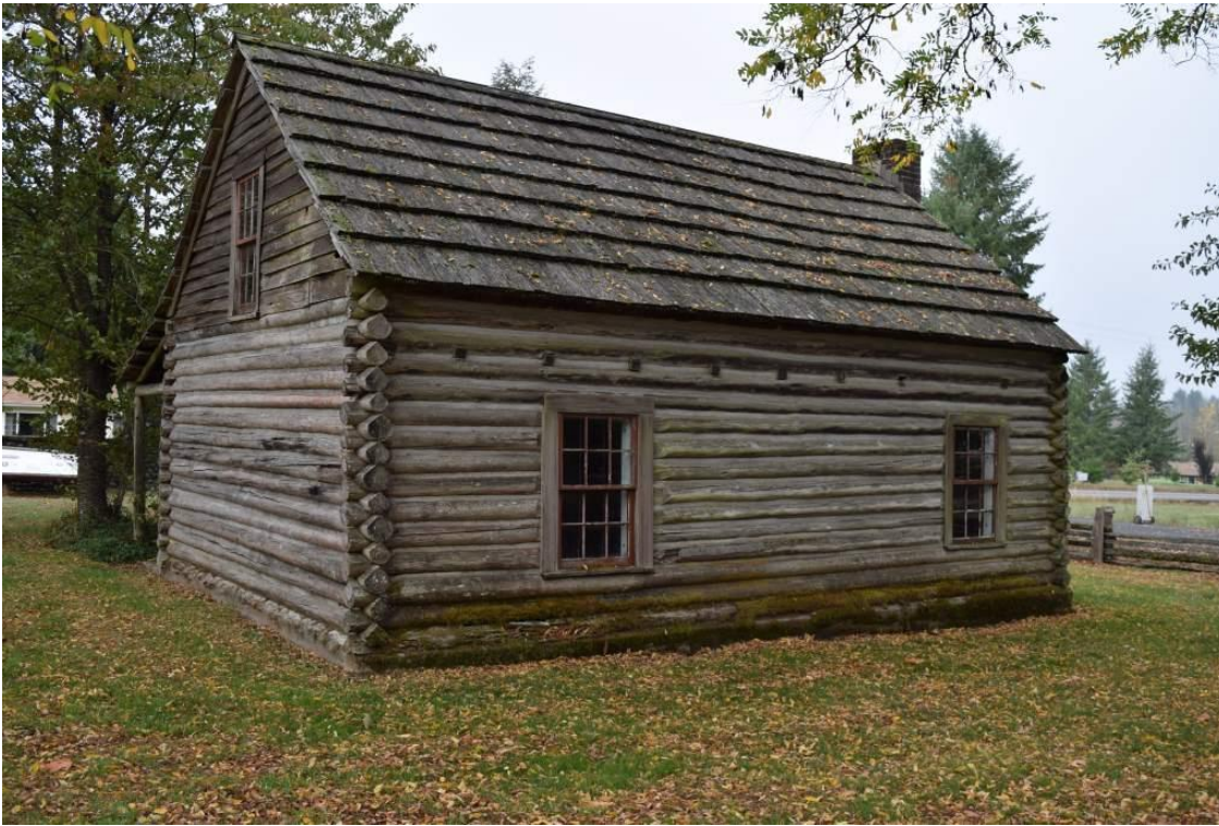
4 of 15. Looking northwest at southeast corner.
